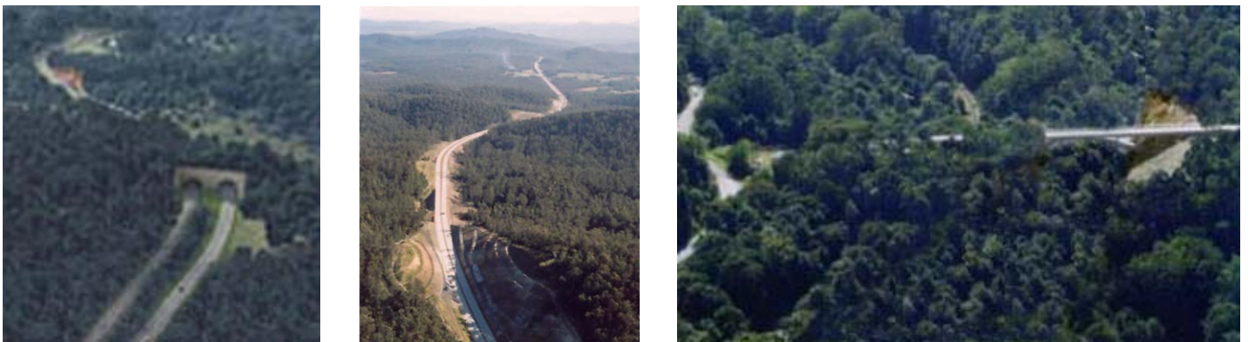
Figures 7.4 (Potential Urban Design Outcomes). Examples of potential landscape treatments for the Coastal Ridge Way. From left to right: a modified image based upon the Cudgen Road Tunnel on the Yelgun to Chinderah project demonstrating a tunnel through a forested area, a deep cutting on the Bulahdelah to Coolongolook Deviation demonstrating the scale of cutting required through an undulating terrain, and a modified image based upon a bridge along the Yelgun to Chinderah Pacific Highway upgrade demonstrating a bridge through a forested area.
