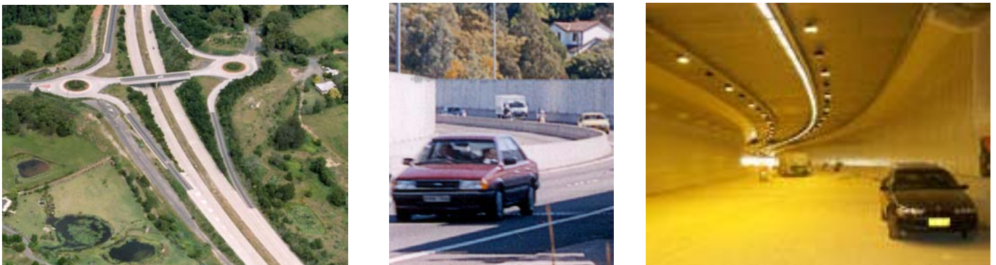
Figures 8.2 (Potential Urban Design Outcomes). Examples of potential urban design outcomes for the Existing Highway. From far left to right: an aerial view of Lyons Road / Pacific Highway interchange, an enclosed road corridor formed by walls on both sides on the Gore Hill freeway, and a tunnel along the Nundah bypass in Queensland.
