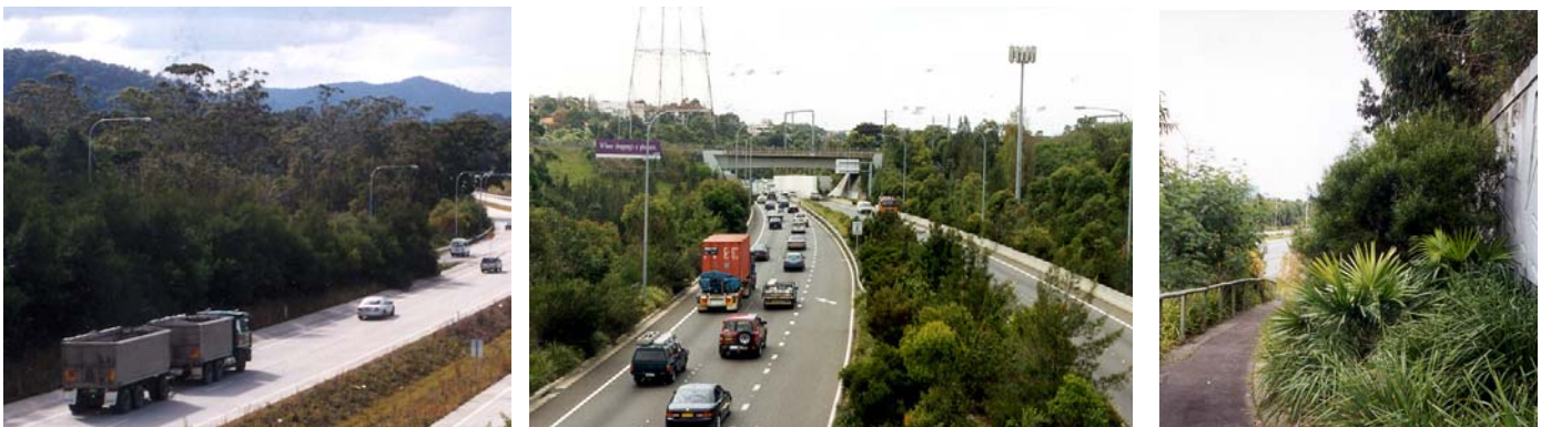
Figures 8.4 (Potential Urban Design Outcomes). Examples of potential landscape treatments for the Inner Bypass Options. From left to right: a new section of Pacific Highway looking north from Lyons Road overbridge, a vegetative zone on the Gore Hill freeway acting as a noise barrier, and a noise wall and integrated landscape solution along the Gore Hill freeway.
