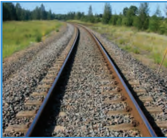
The North Coast Railway would pass to the west of the proposed upgrade in the Collombatti precinct.
