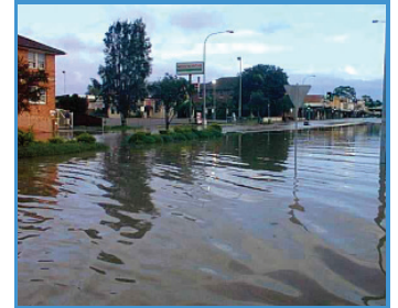
The March 2001 flood in Kempsey severed access along Smith Street in the Kempsey town centre
