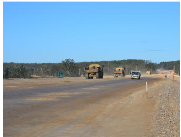
Compacting high traffic areas
