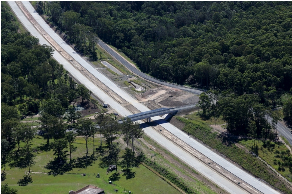
Bridge 2 Open to traffic
