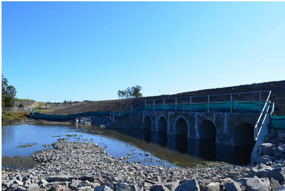
Cross drainage culverts at the unnamed drainage line north of Frederickton
