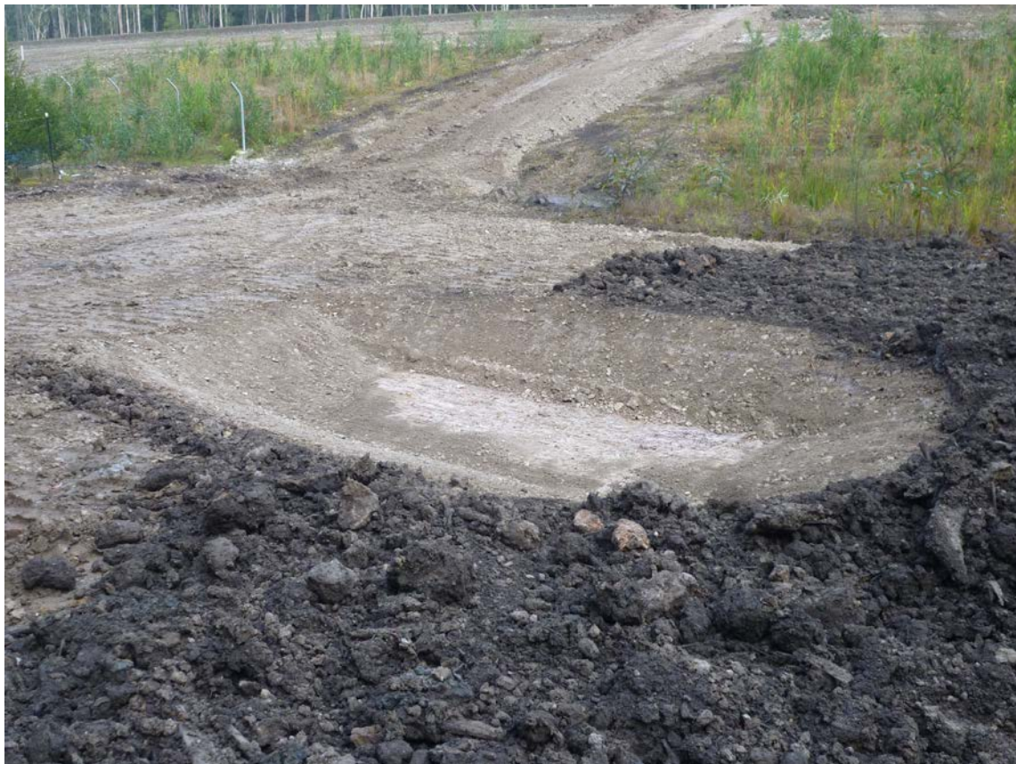
Green-thighed Frog Pond during construction in former sediment basin at Chainage 26000 – 26200
