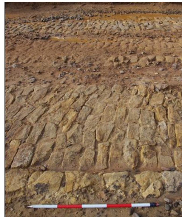
Potential Heritage Item – Road Pavement
