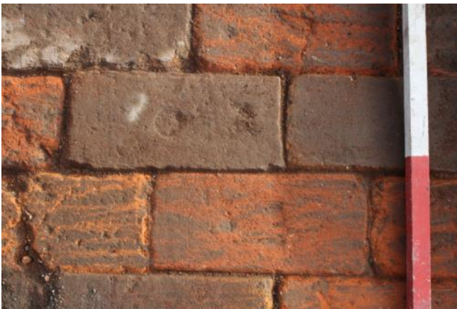
Plate 8: Triangle shaped frog on bricks exposed as part of the floor of the slab hut.
