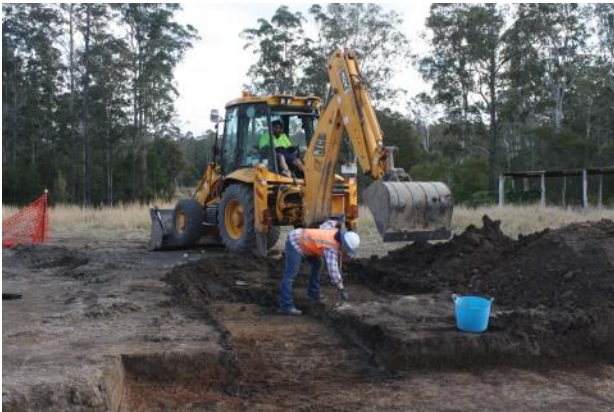
Plate 33: Machine excavation in the north west corner of Area 3, facing west. An artefact rich deposit [C074] was found below C001.
