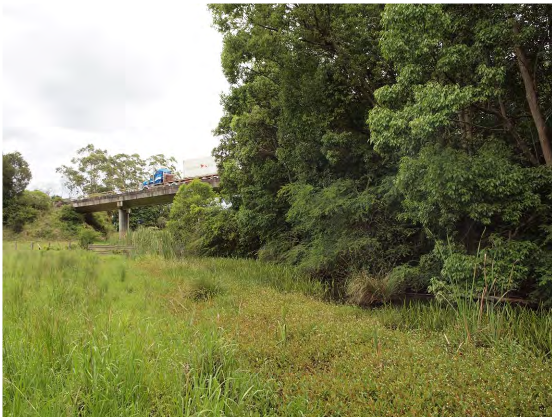
Plate 8: Crouches Creek with band of Maundia in the creek at the base of slope and edge of tree line. Existing Pacific Highway bridge, looking south-west.
