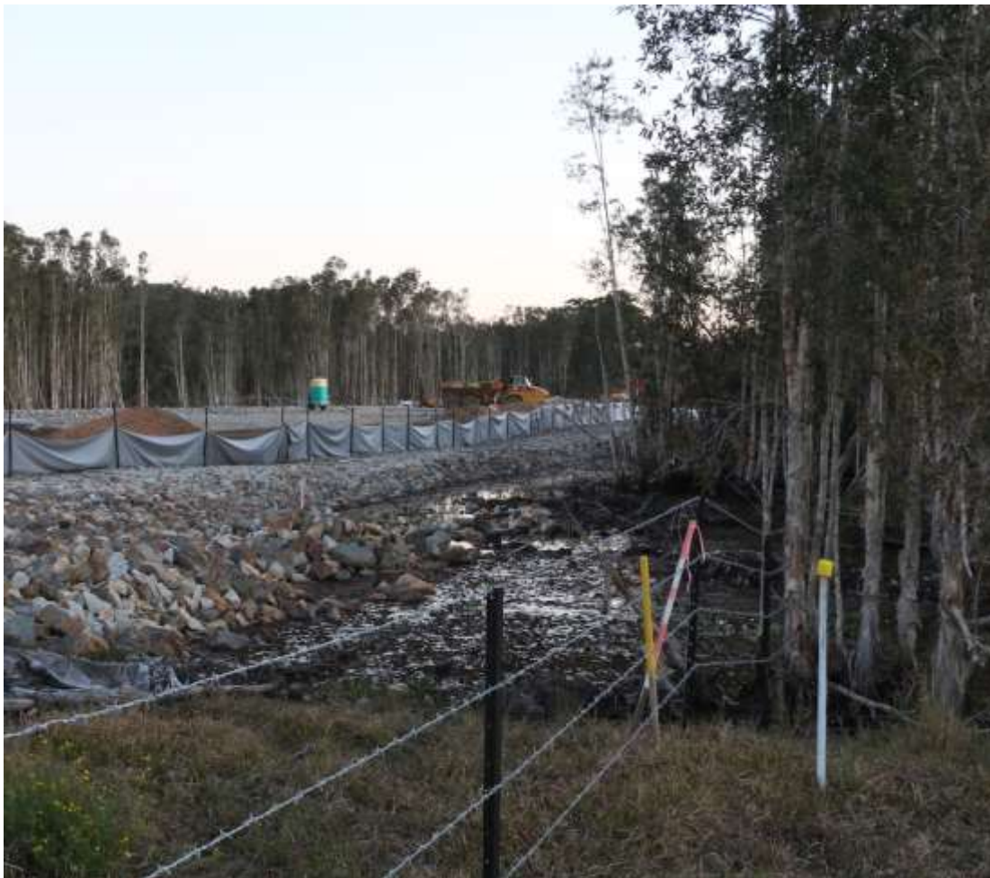
Plate 2.1 Construction at the Site in August 2015
