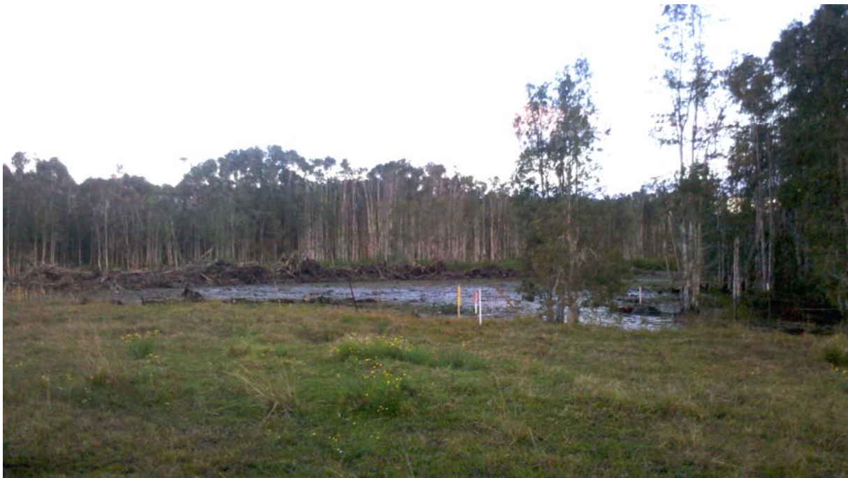
Plate 2.1 Vegetation clearing in June 2015 at the site
