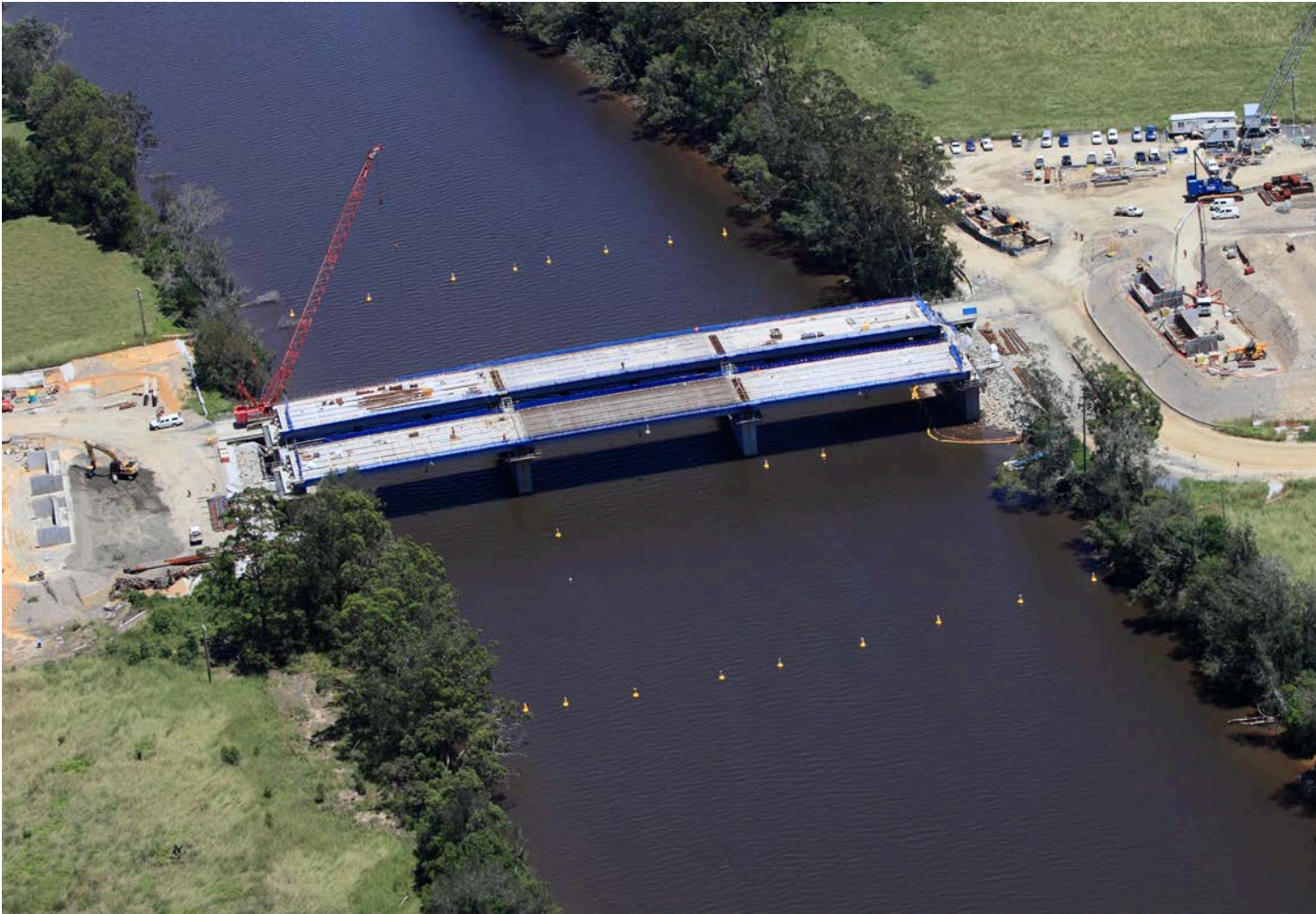
New bridge over Kalang River, January 2015
