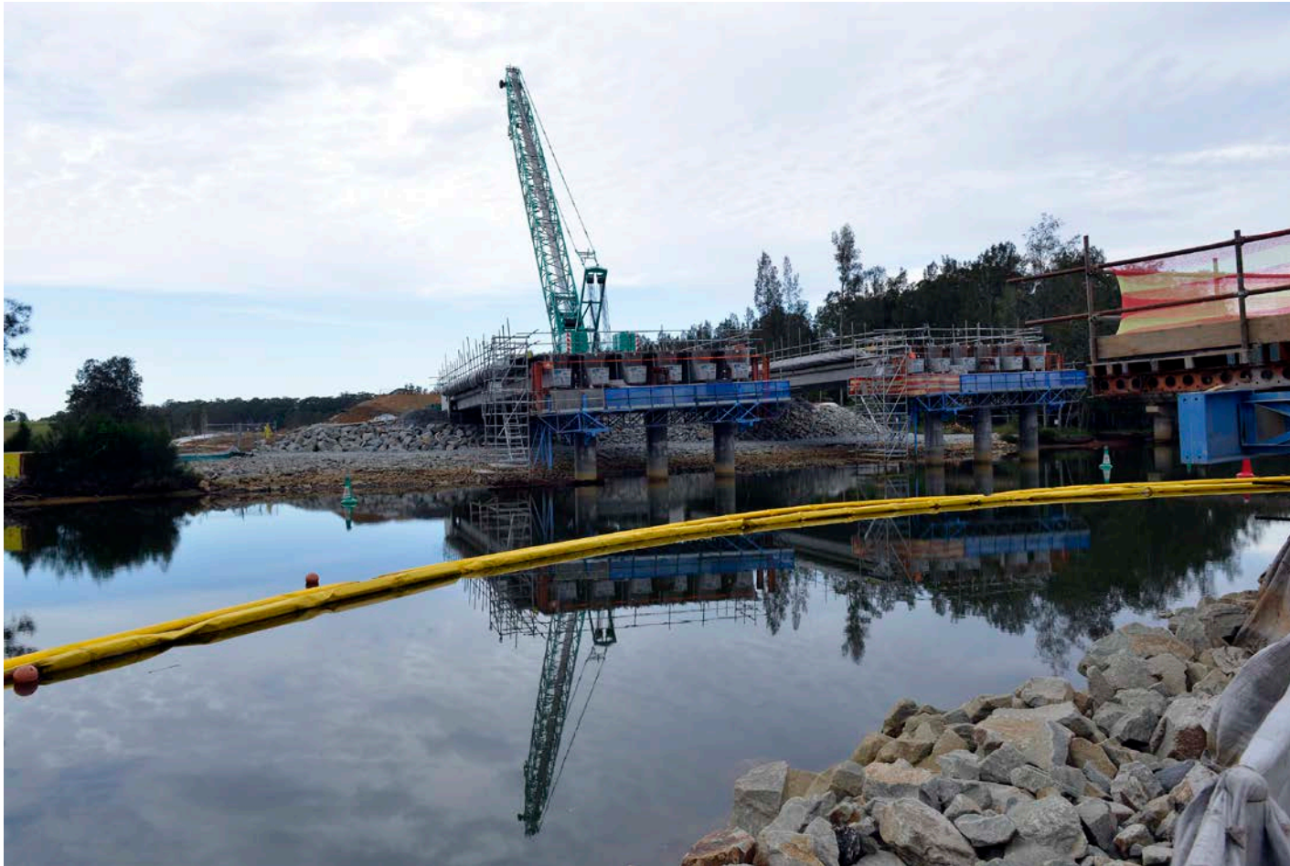
Deep Creek bridge, May 2015
