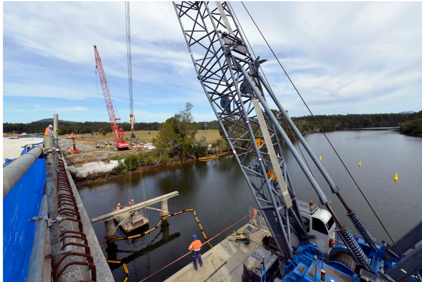
Temporary bridge being removed from Kalang River, May 2015
