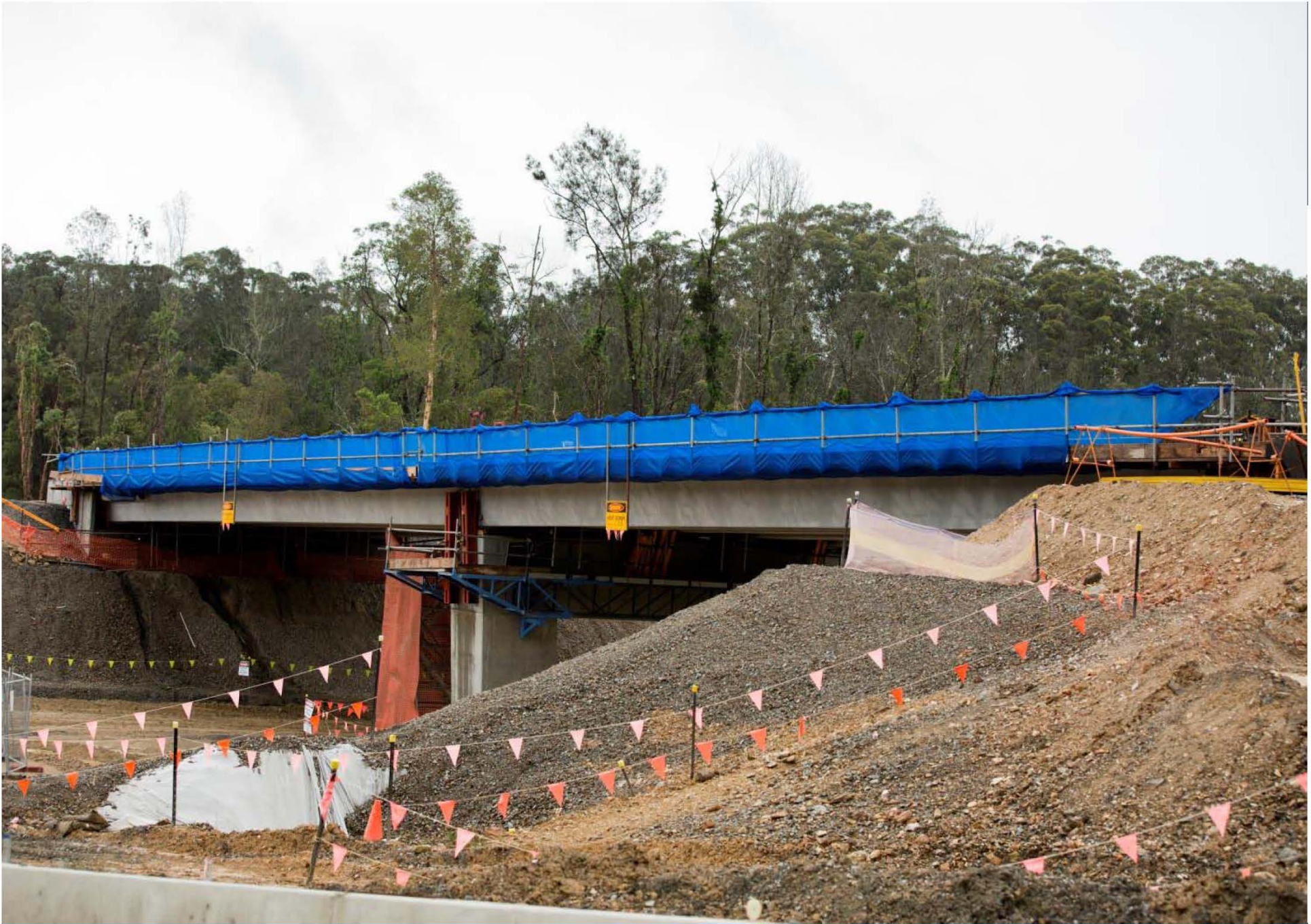
Short Cut Road bridge, November 2014
