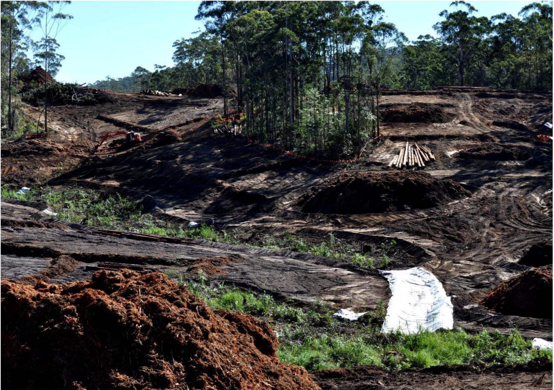
Clearing for main road, Ballards Road, June 2014
