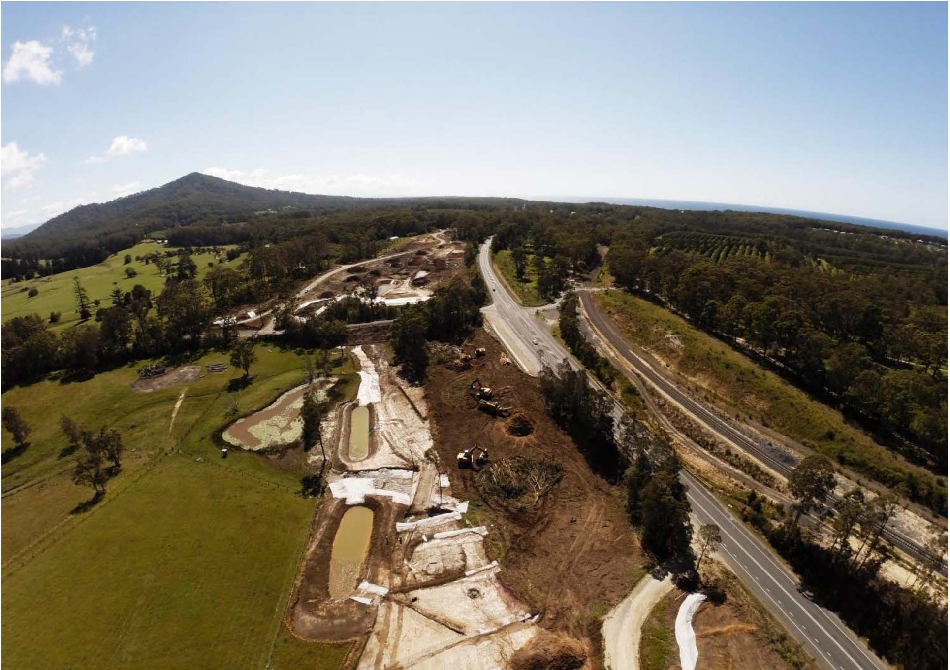
Deep Creek north view, April 2014
