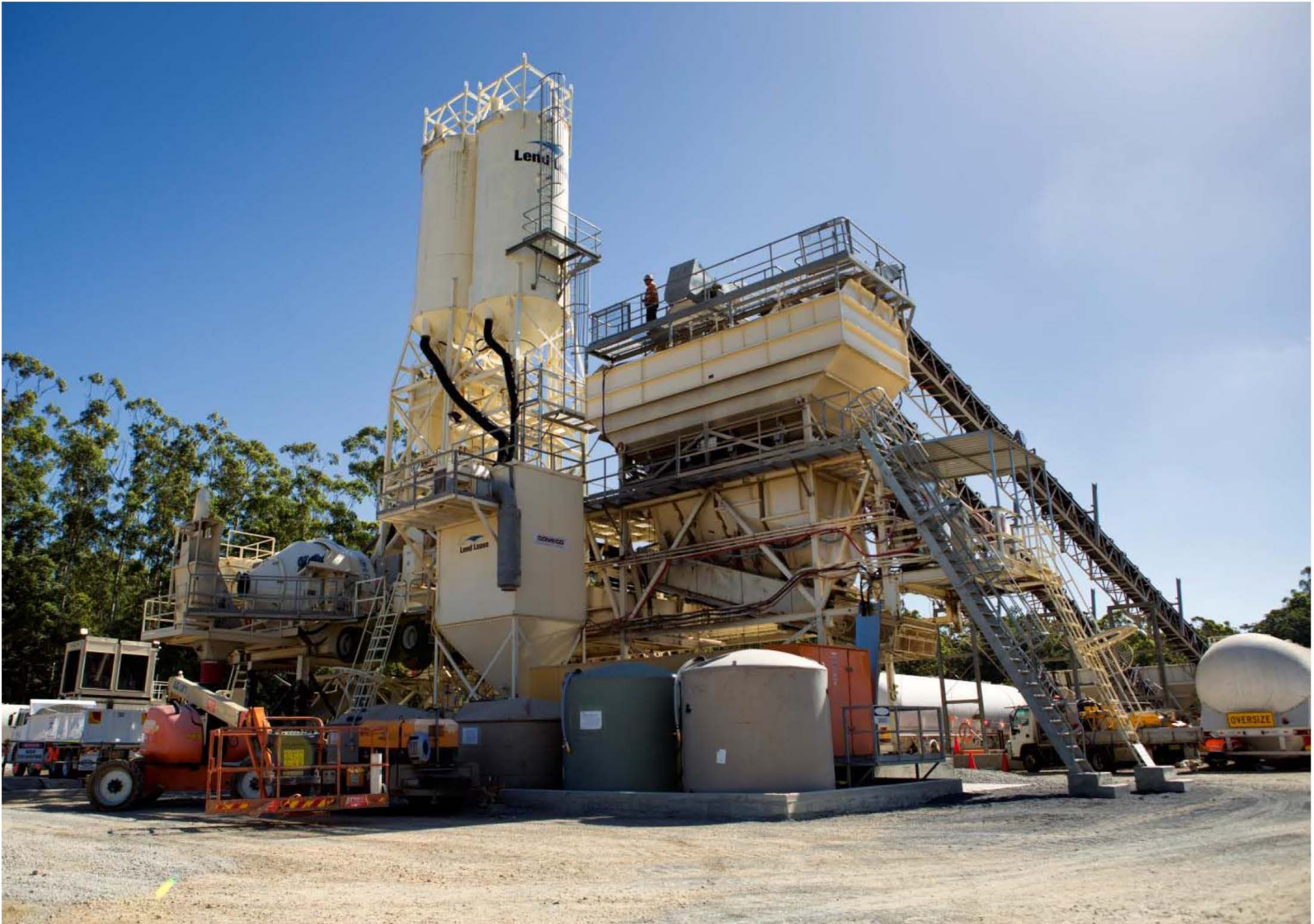
Site batch plant
