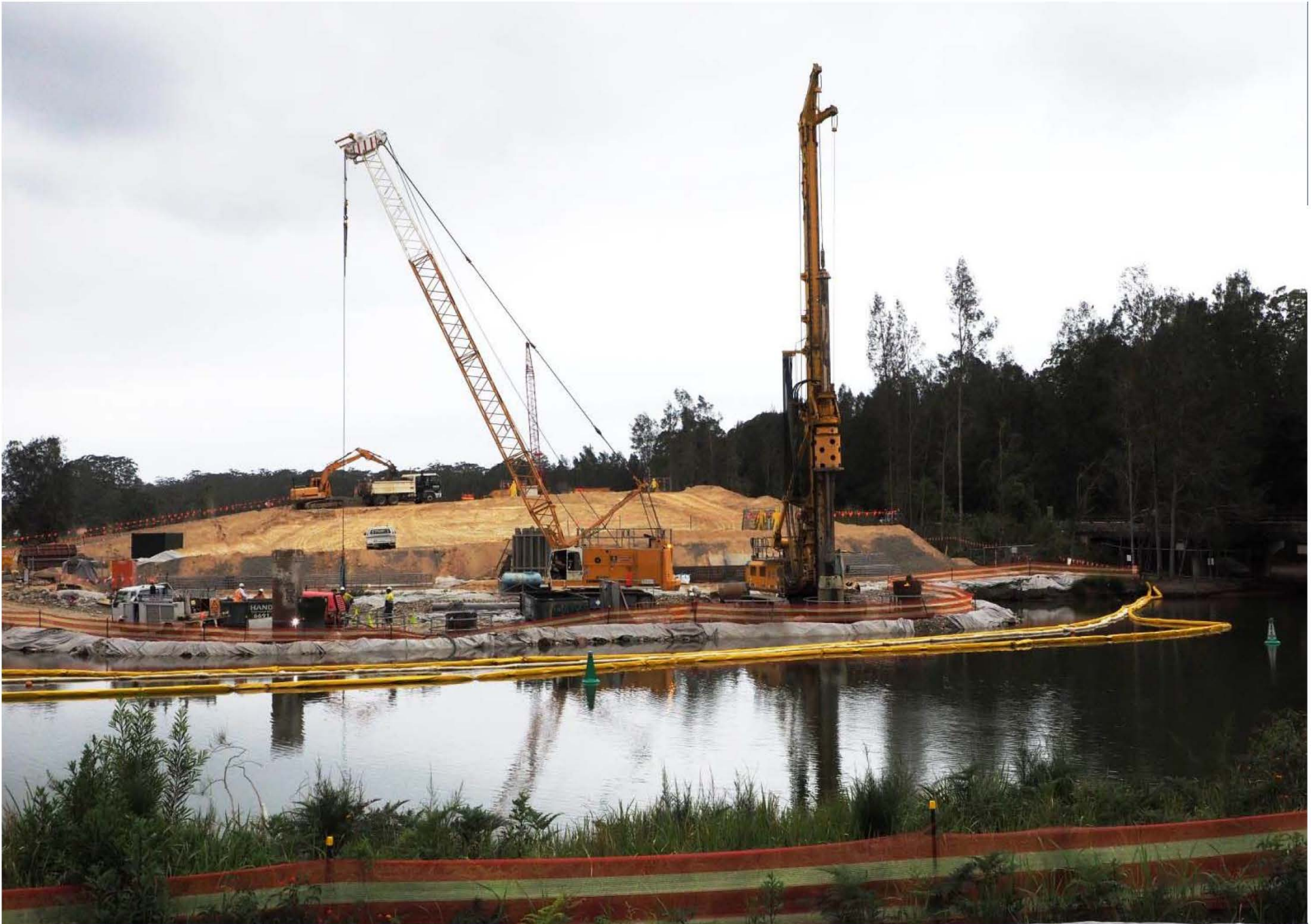
Piling at Deep Creek, November 2014
