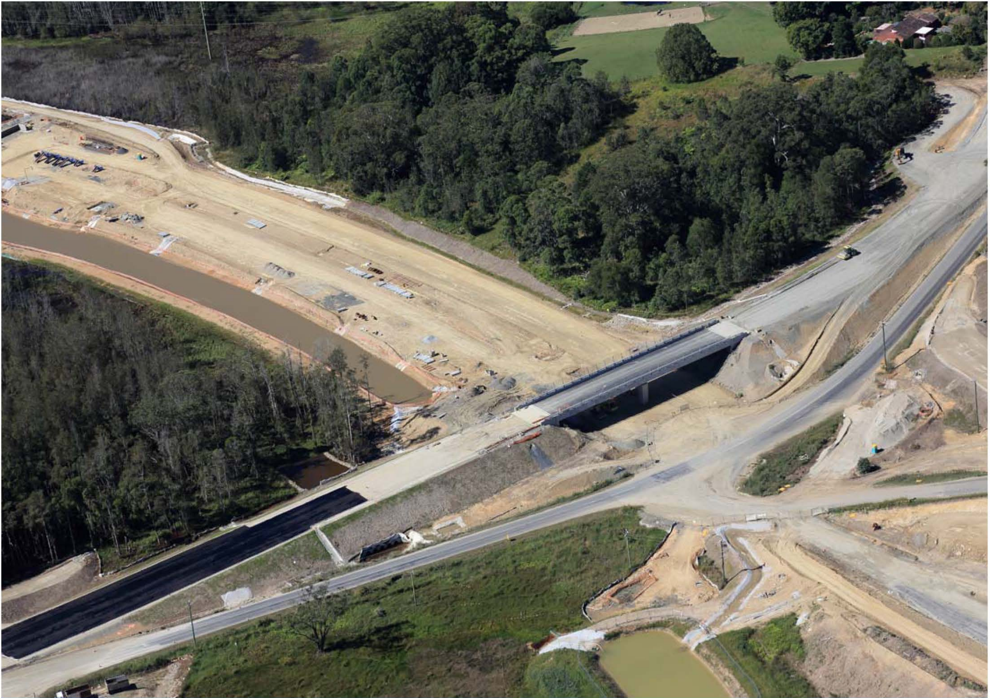
Short Cut Road bridge, April 2015
