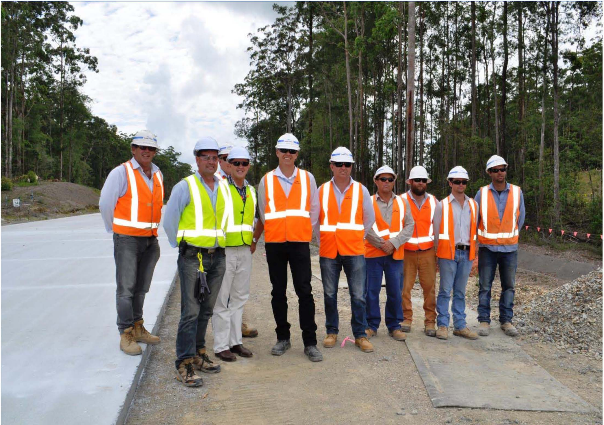
Media event to mark the start of paving, March 2015 - 82
