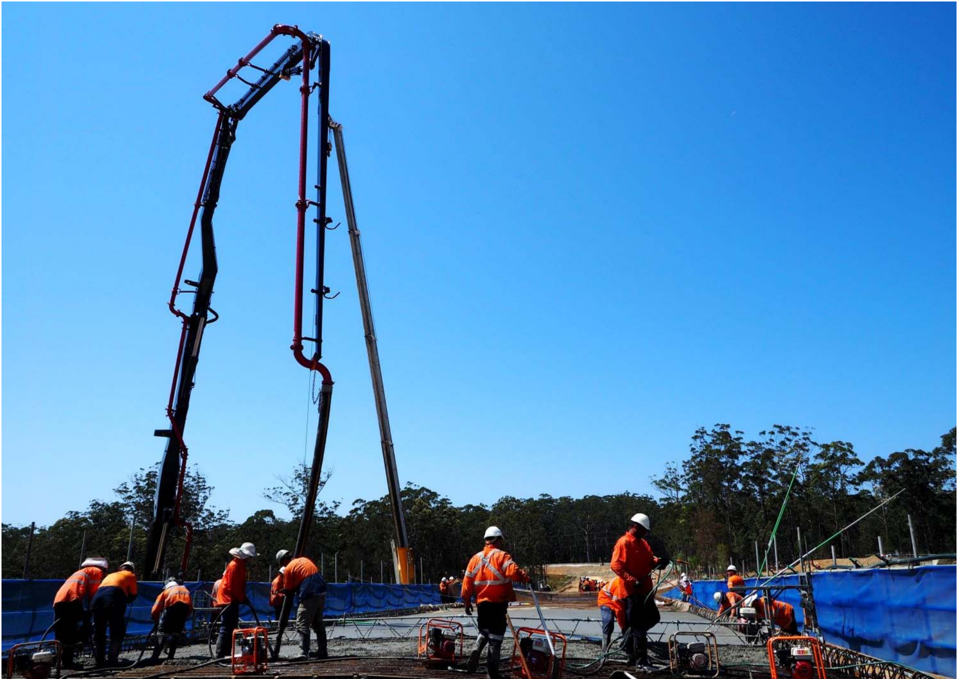
Ballards Road bridge, September 2014
