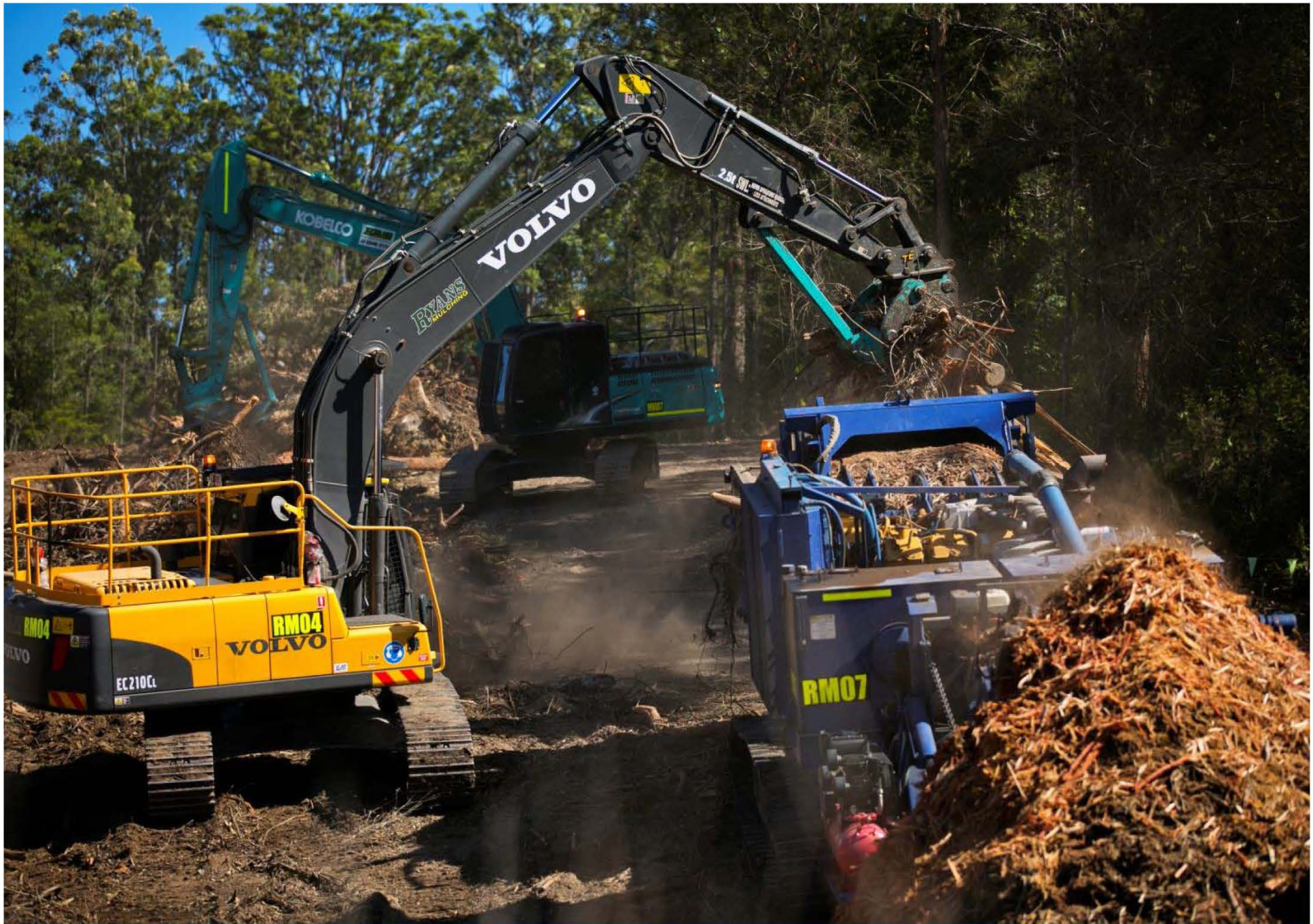
Clearing work at Cut 32, January 2014
