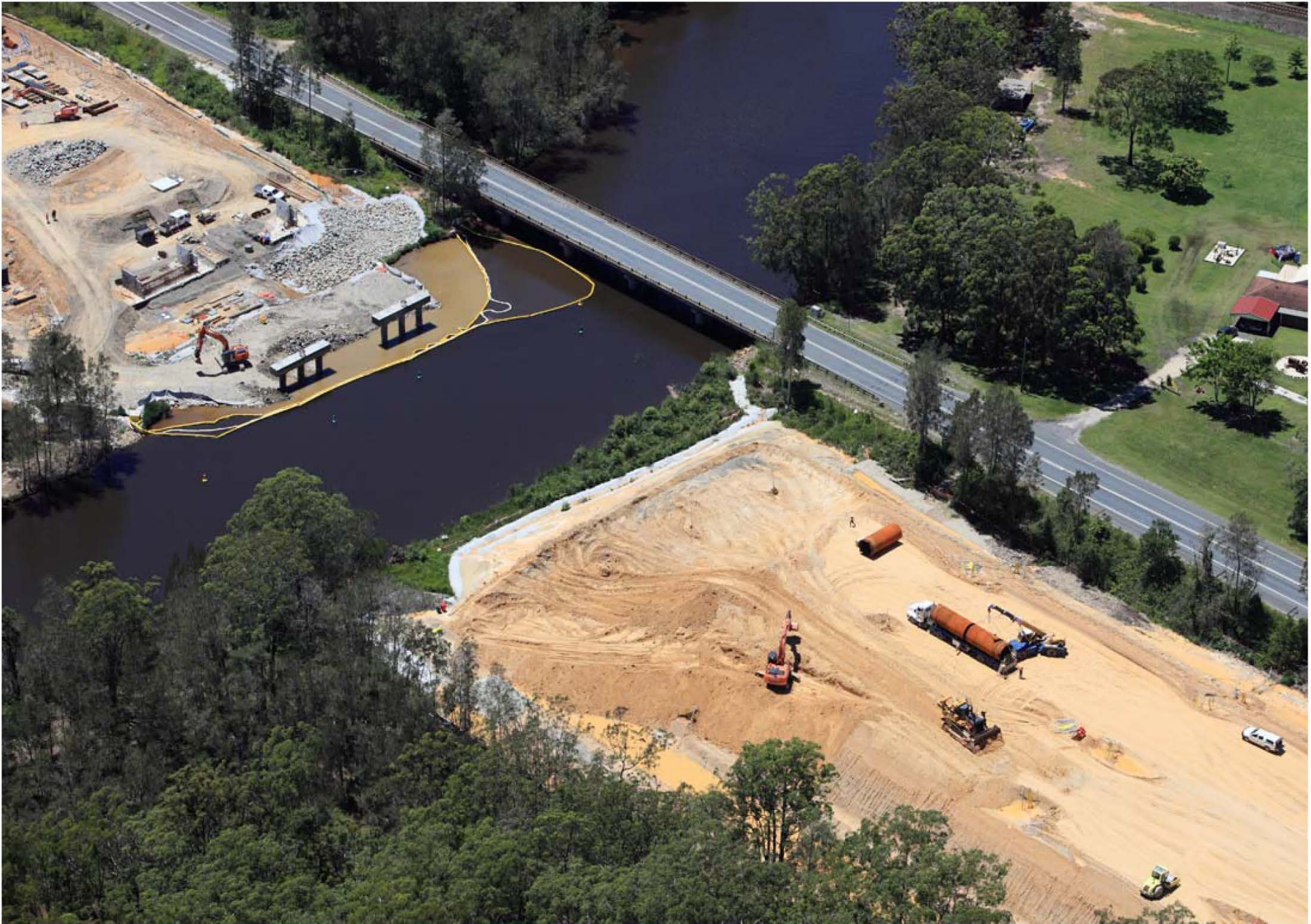
Twin bridges at Deep Creek, January 2015
