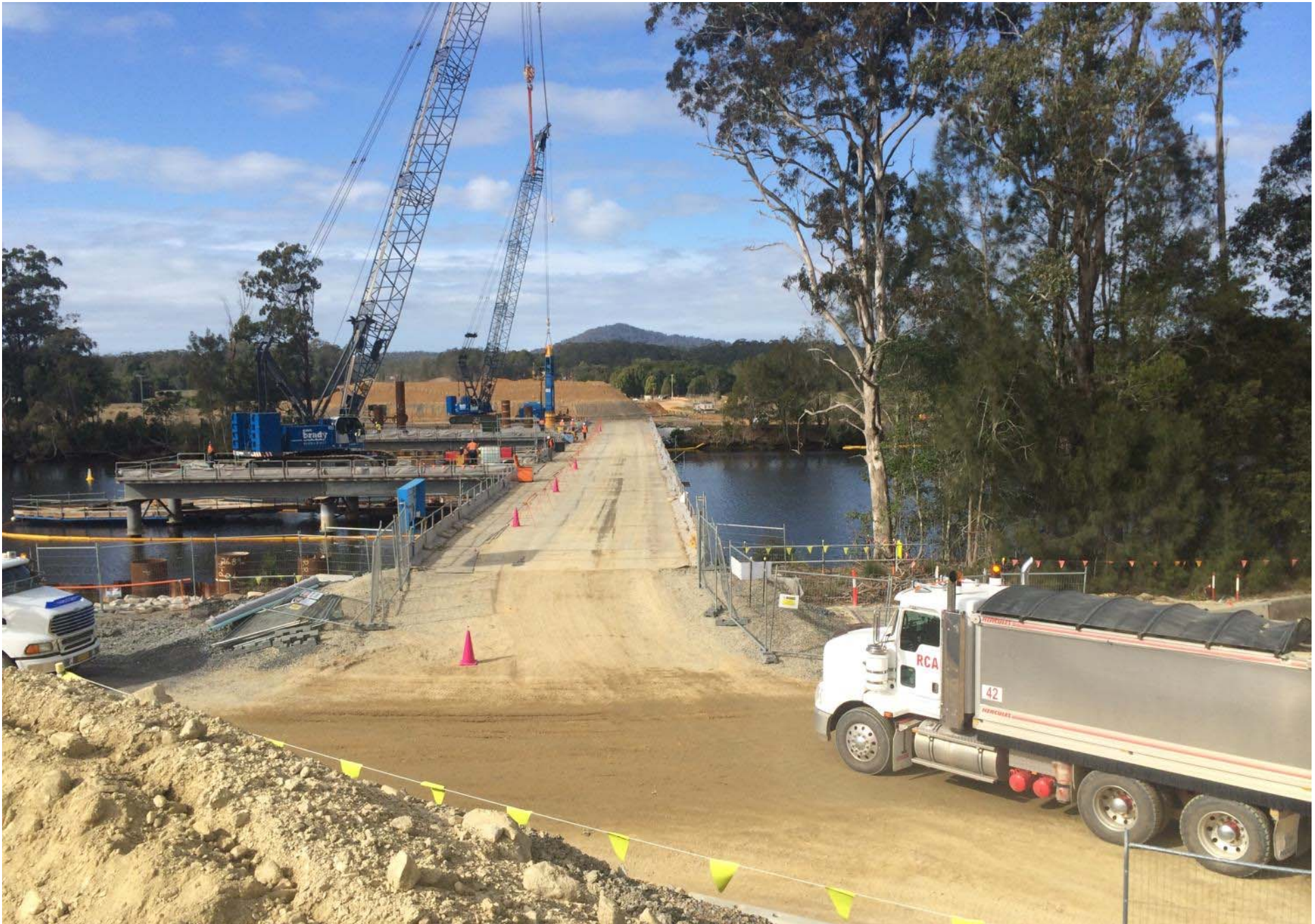
Kalang River temporary bridge, September 2014 - 32
