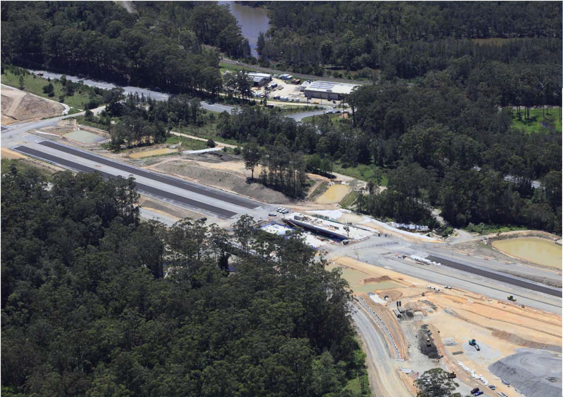
Boggy Creek and service road, November 2015 - 63
