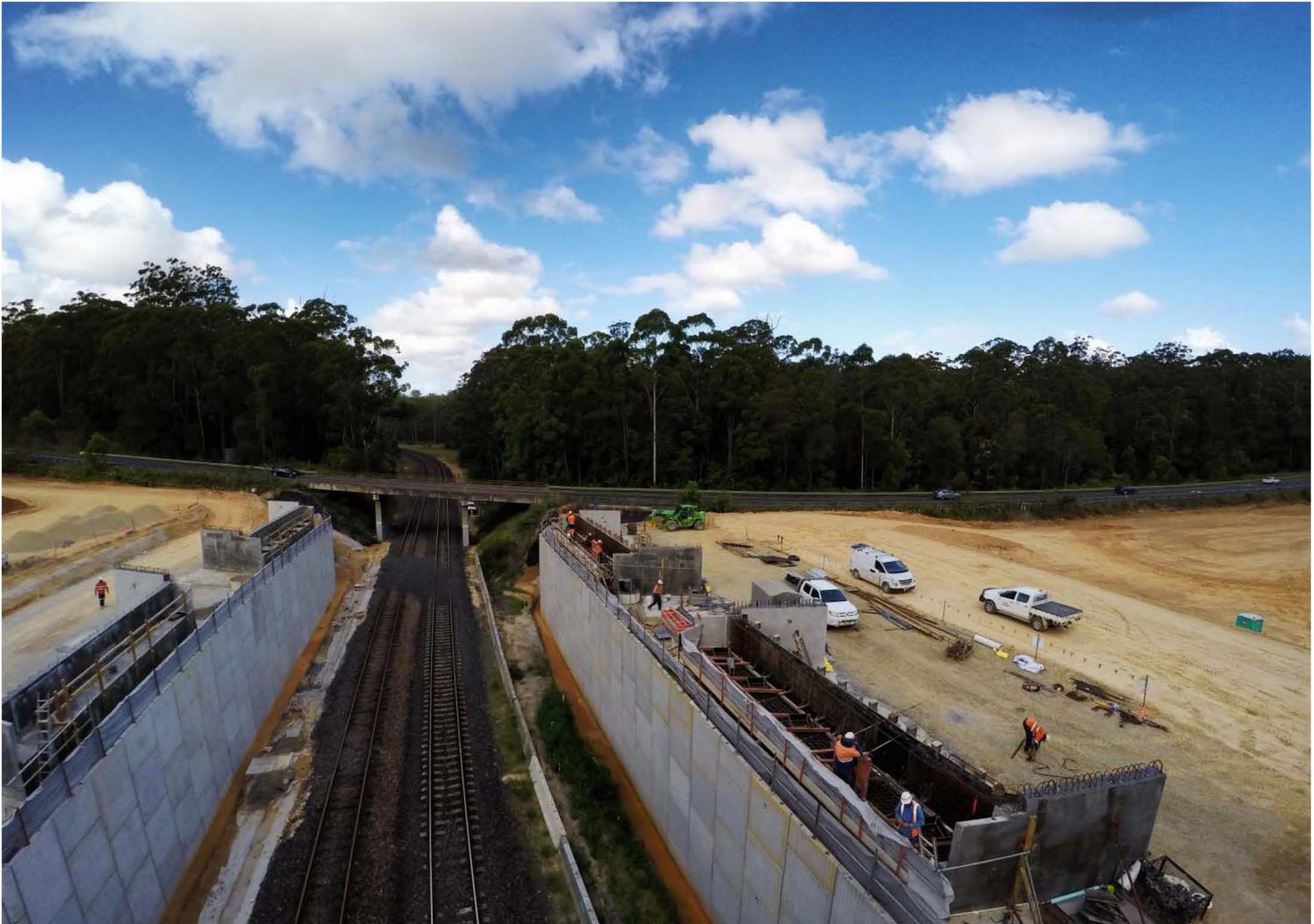
North Coast Rail bridge, February 2015
