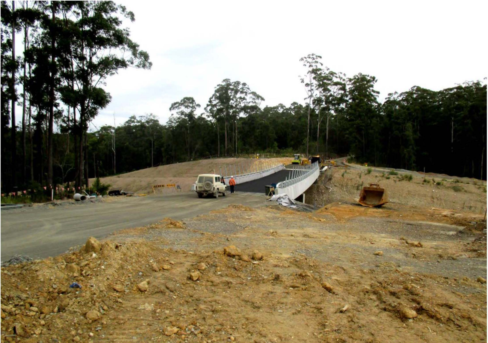
Martells Road bridge, May 2015
