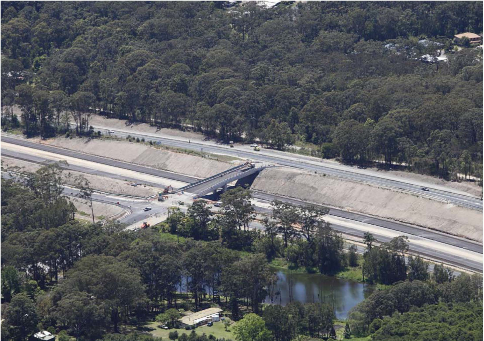
East West Road bridge, November 2015
