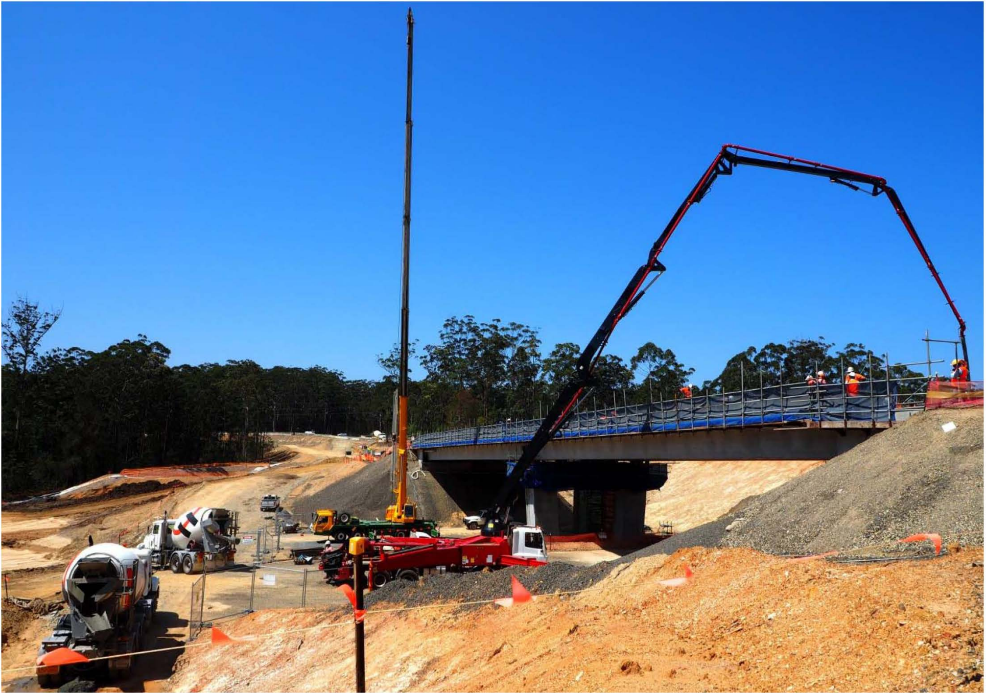
Deck pour at Ballards Road bridge, September 2014 - 17
