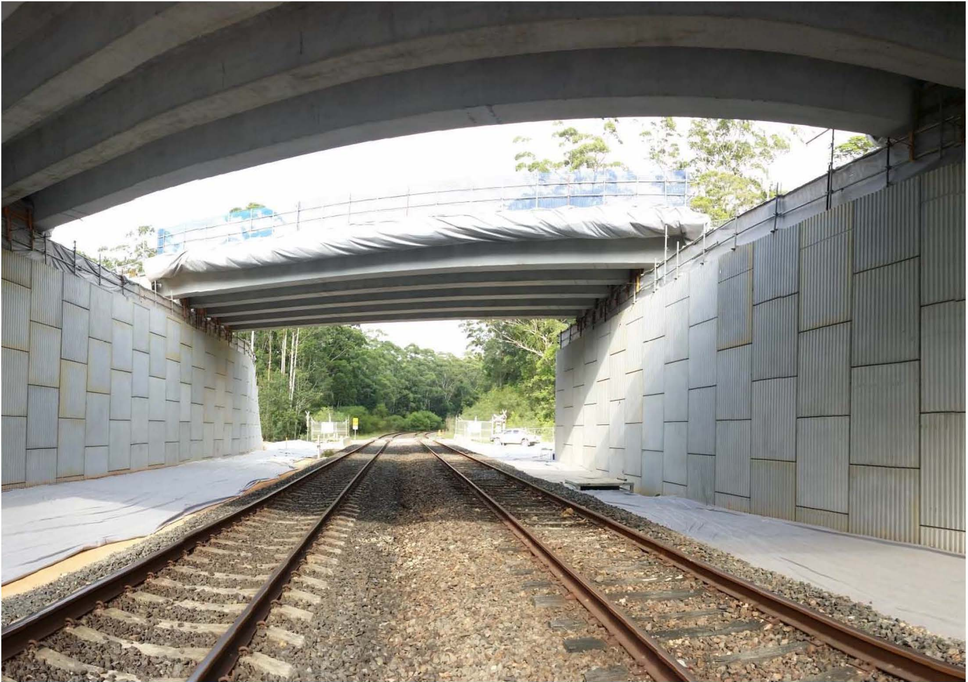
North Coast Rail bridge, March 2015
