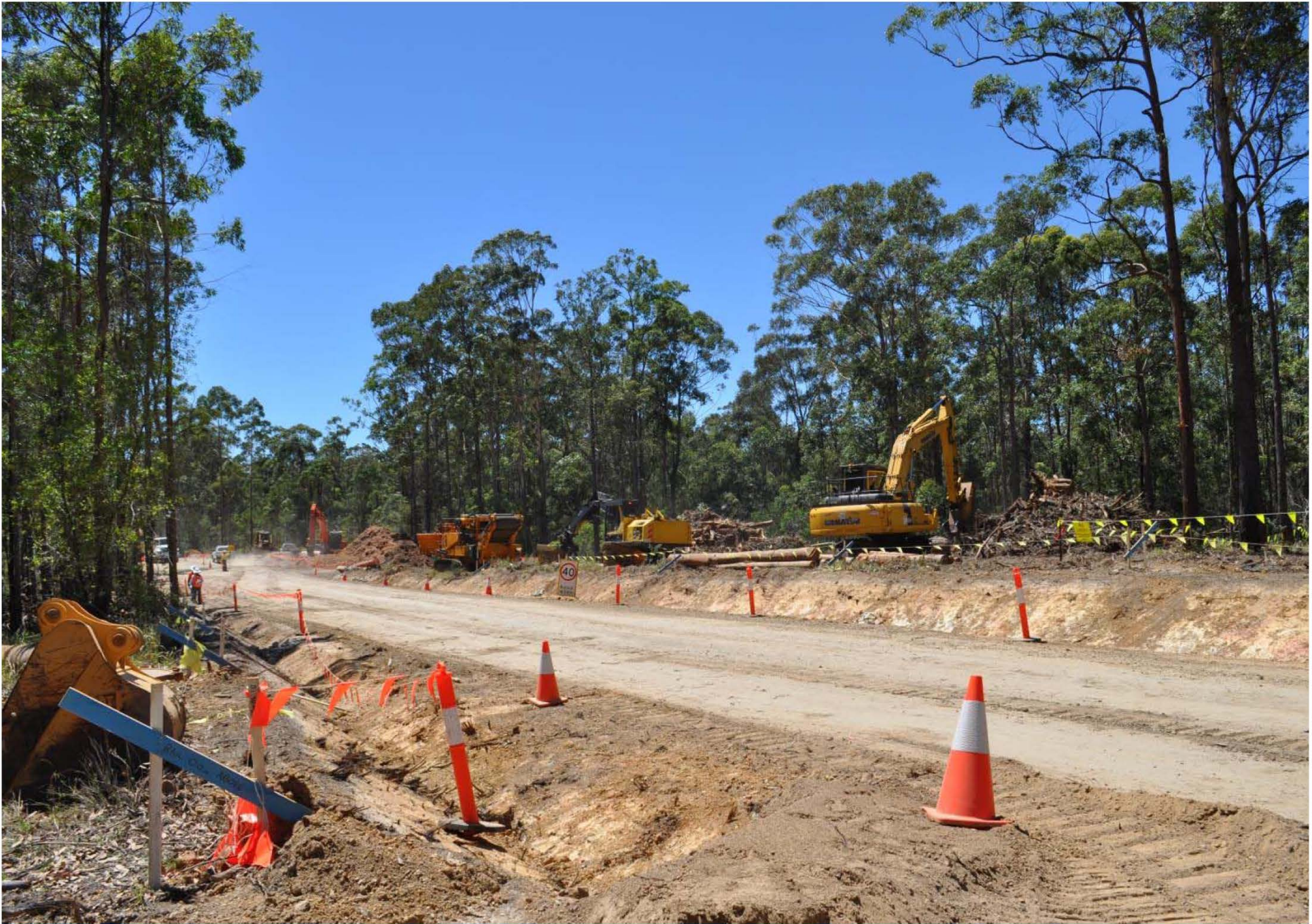
Widening of Ballards Road, December 2013
