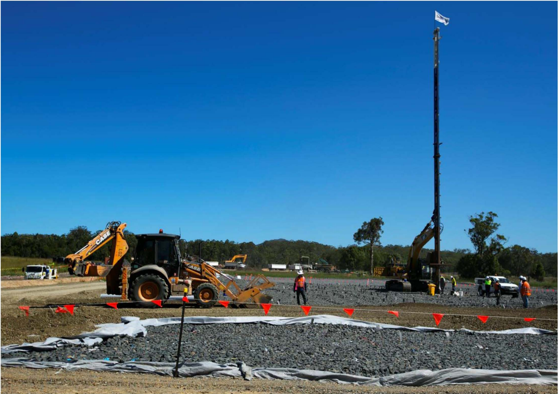
Soft soil work at Kalang River, January 2014
