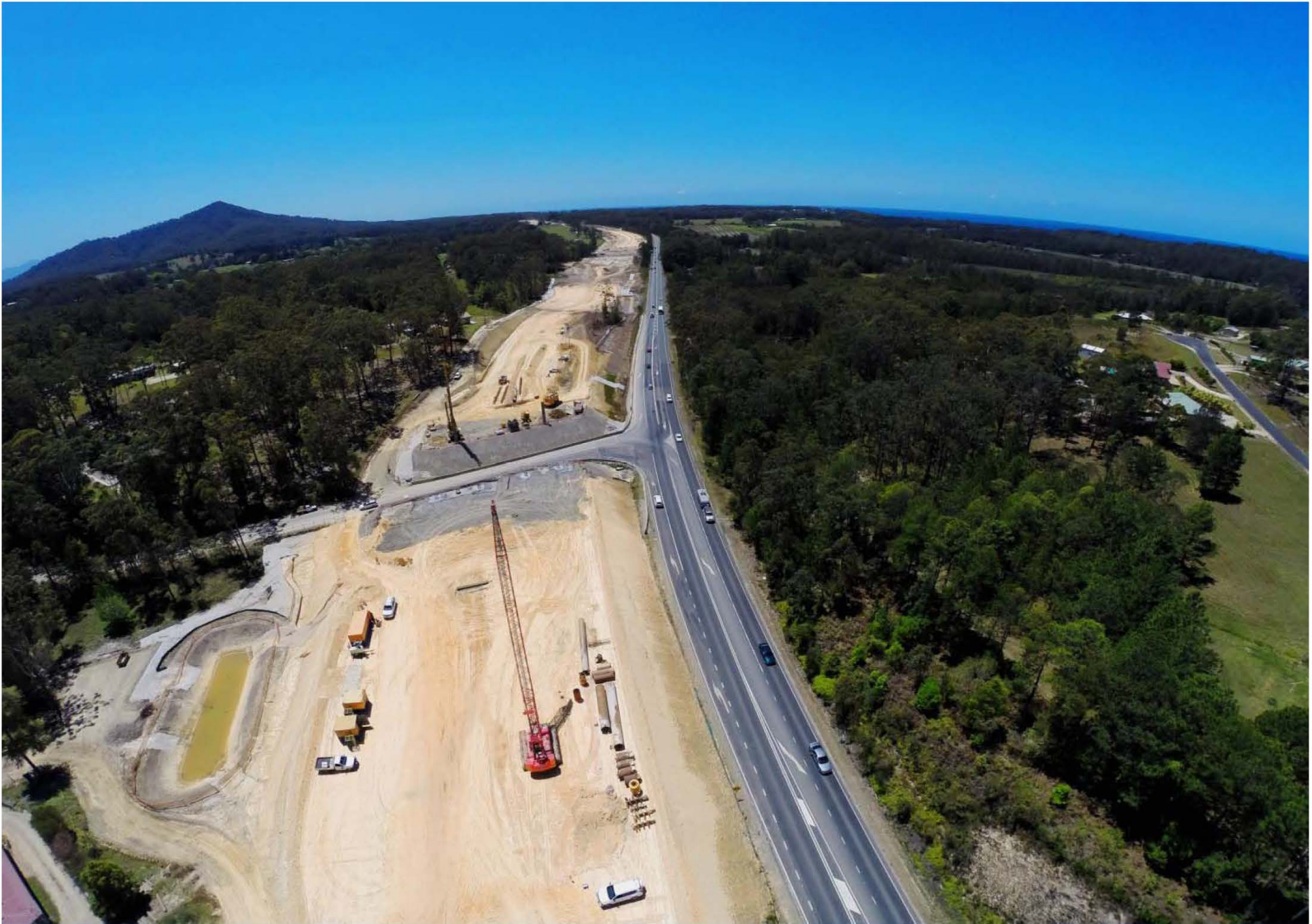
Valla Road bridge, October 2014
