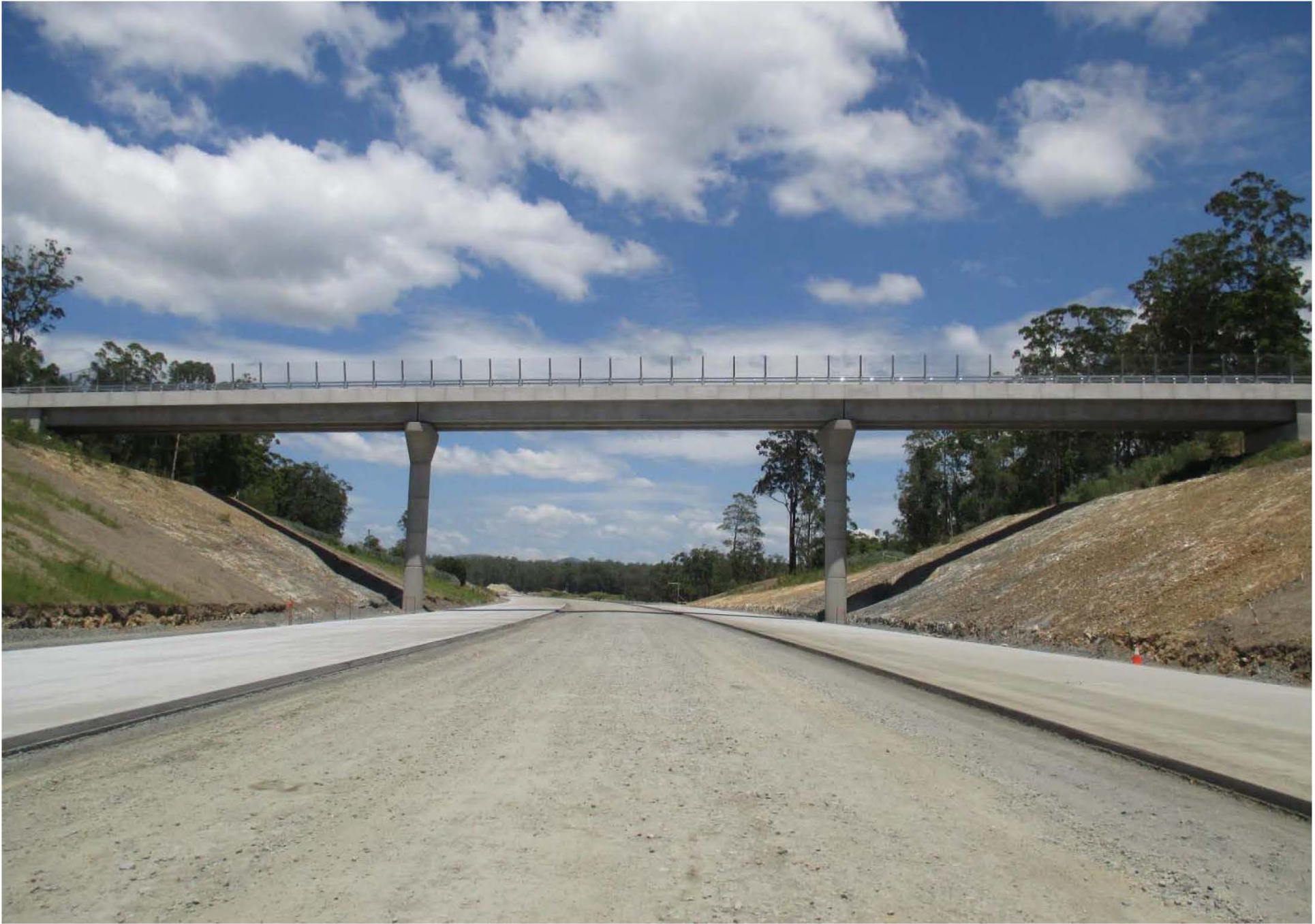
View to South Access Road G, February 2016
