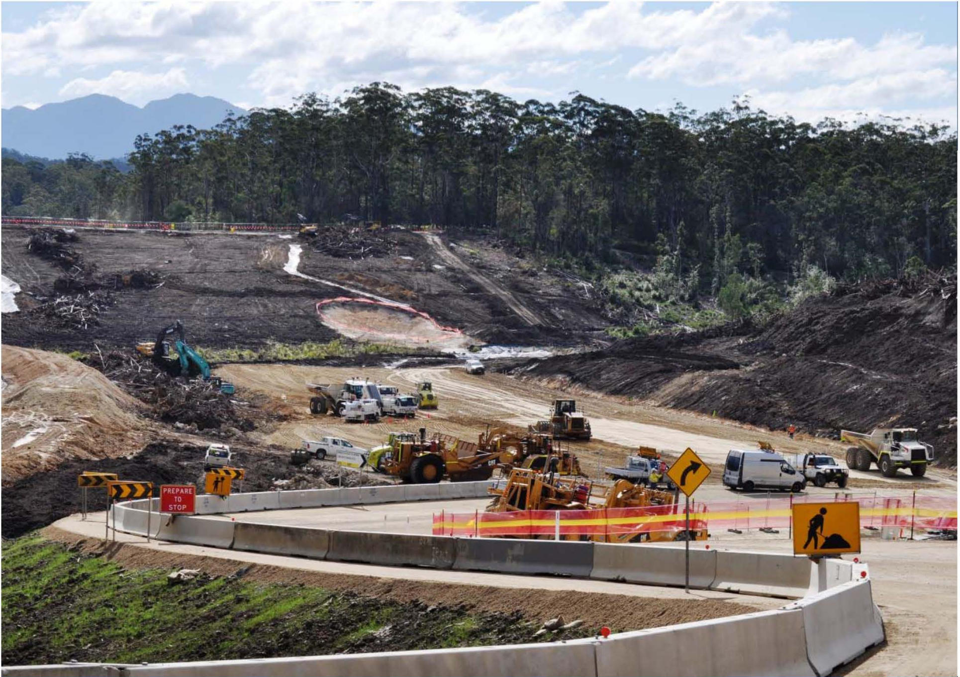
Traffic switch at Martells Road, June 2014
