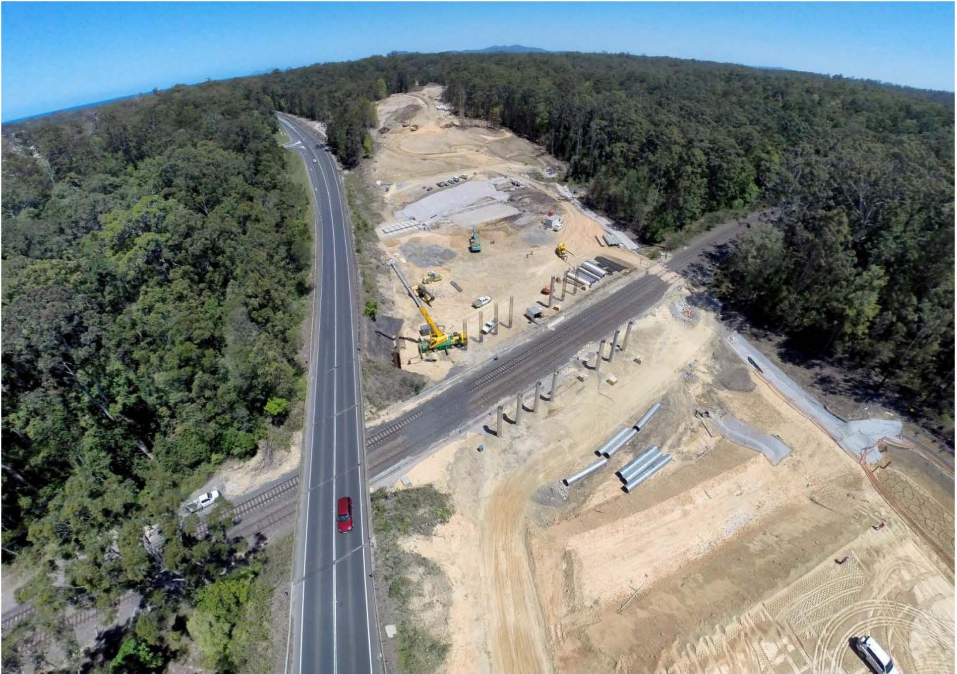
North Coast Rail bridge, October 2014
