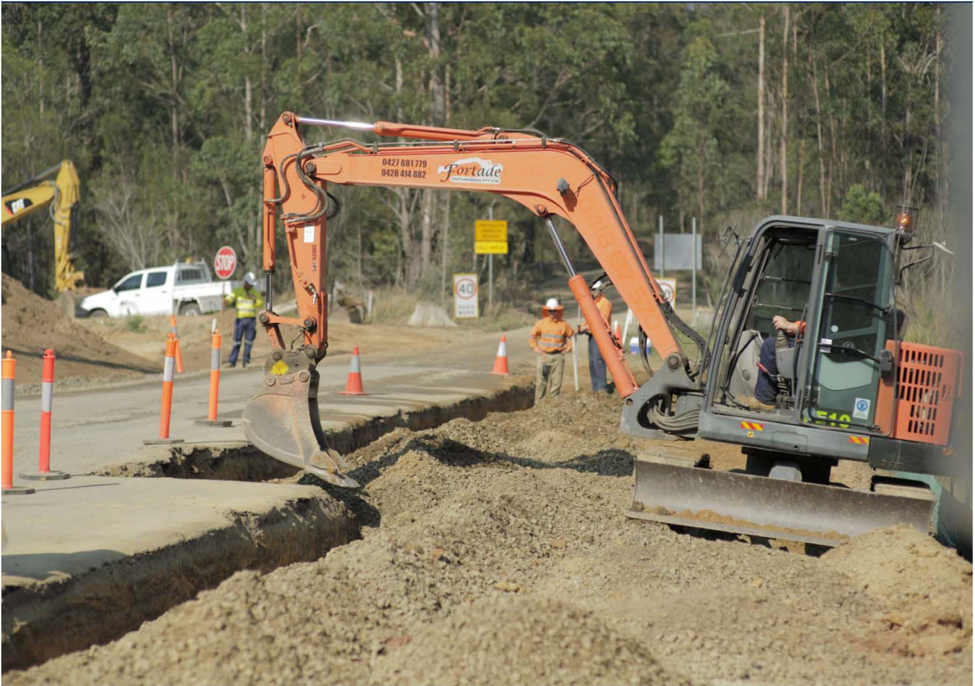
Widening of Ballards Road, November 2013
