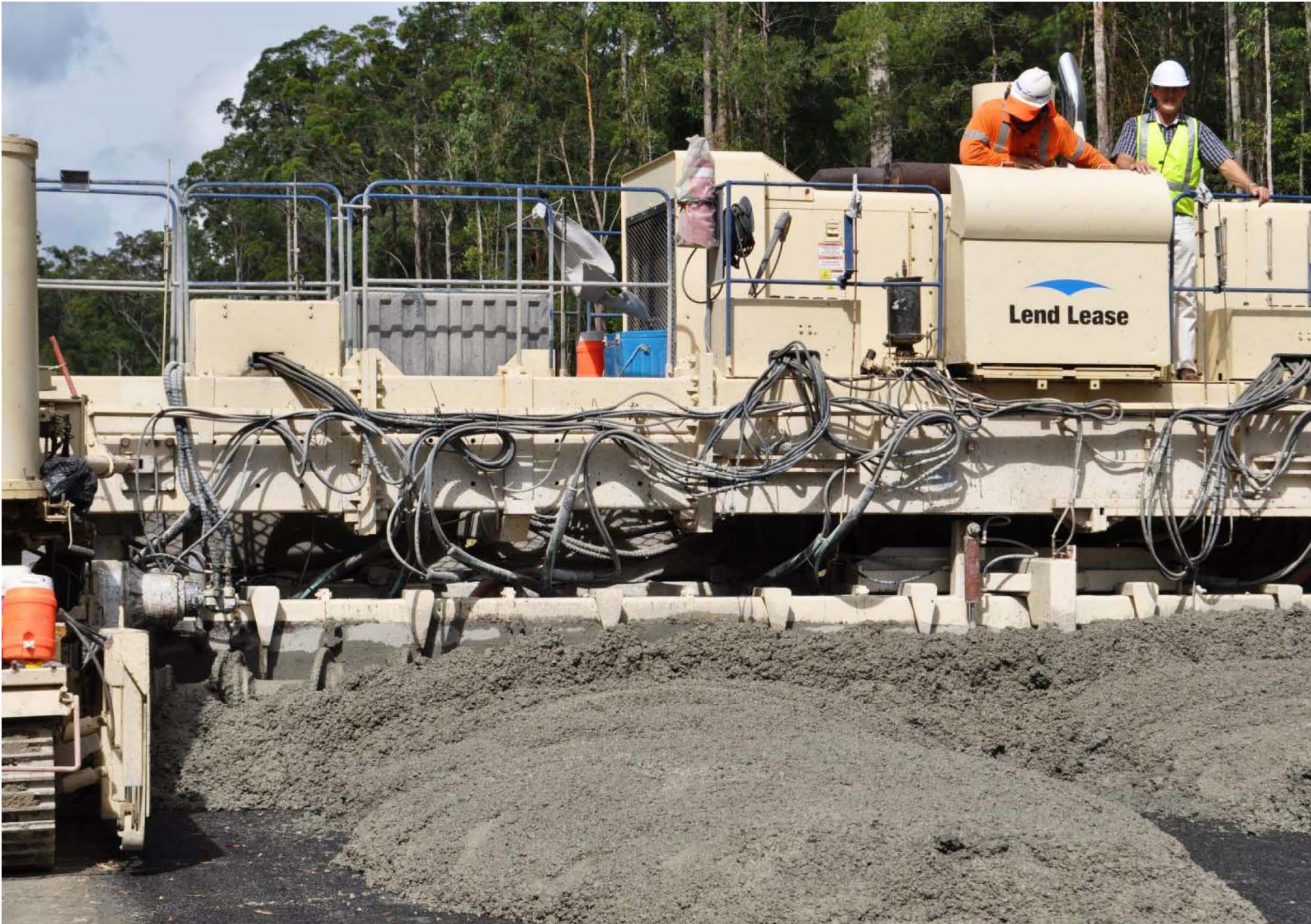
Paving began, March 2015
