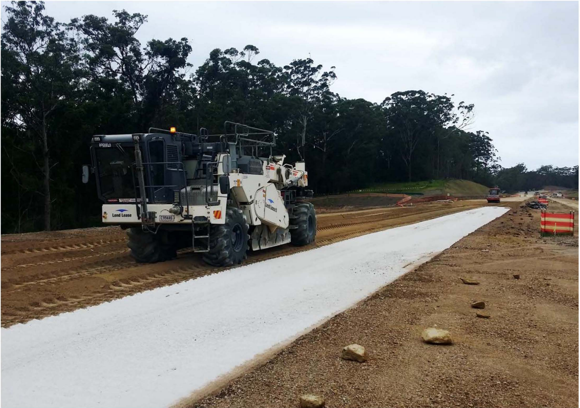
Stabilising work north of Burkes Lane, February 2015 - 95
