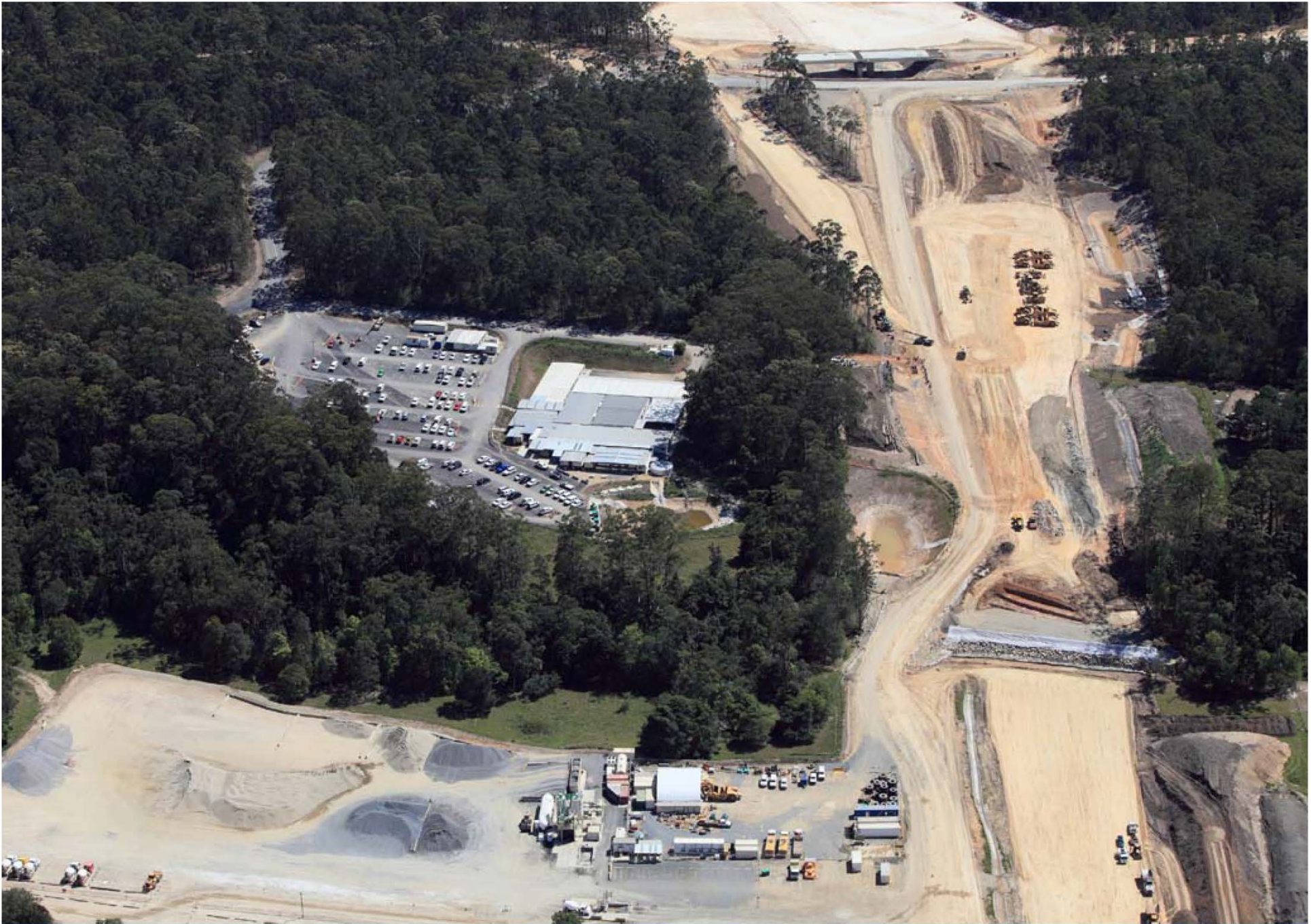
View of Ballards Road, October 2014
