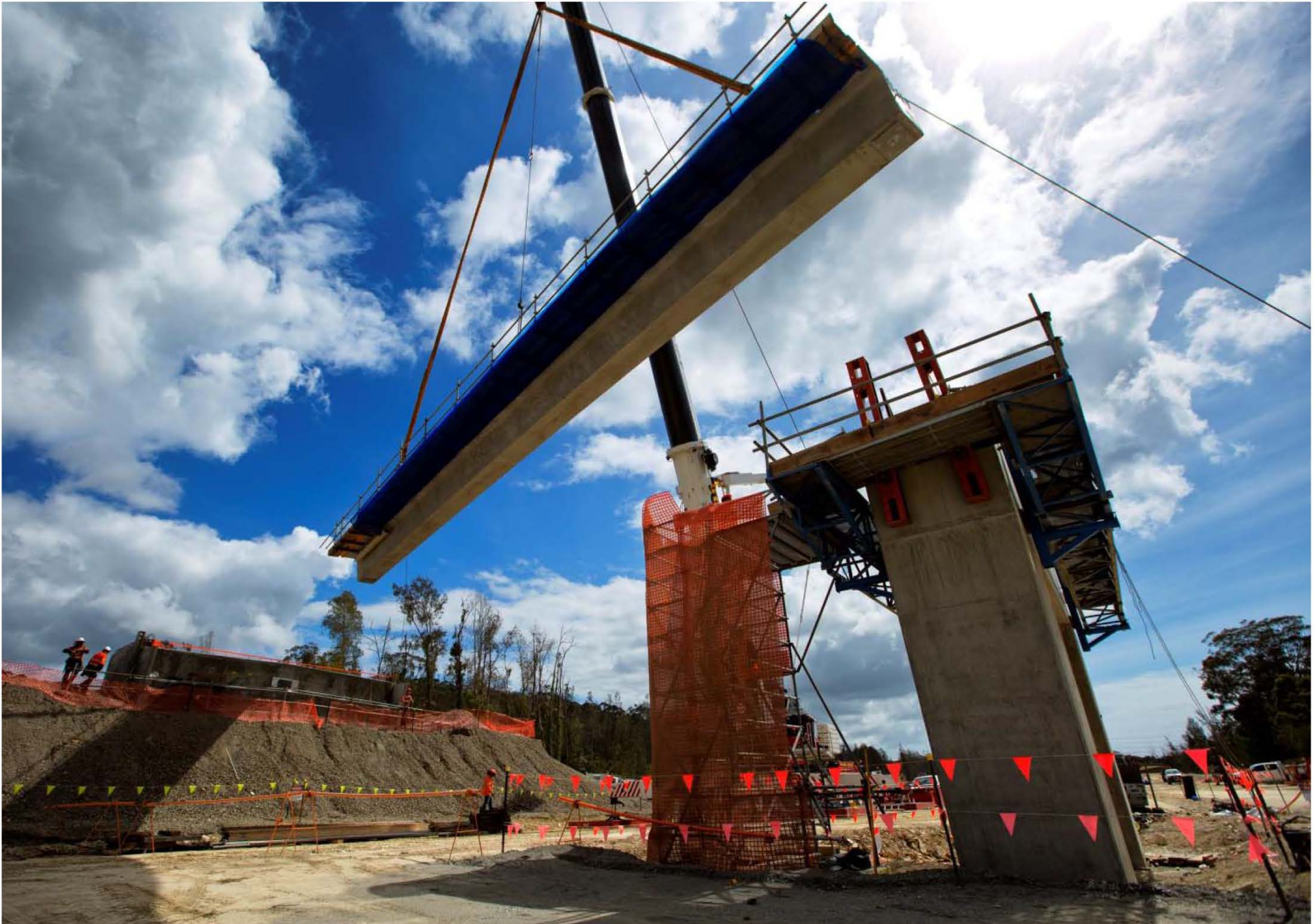
Short Cut Road bridge, November 2014
