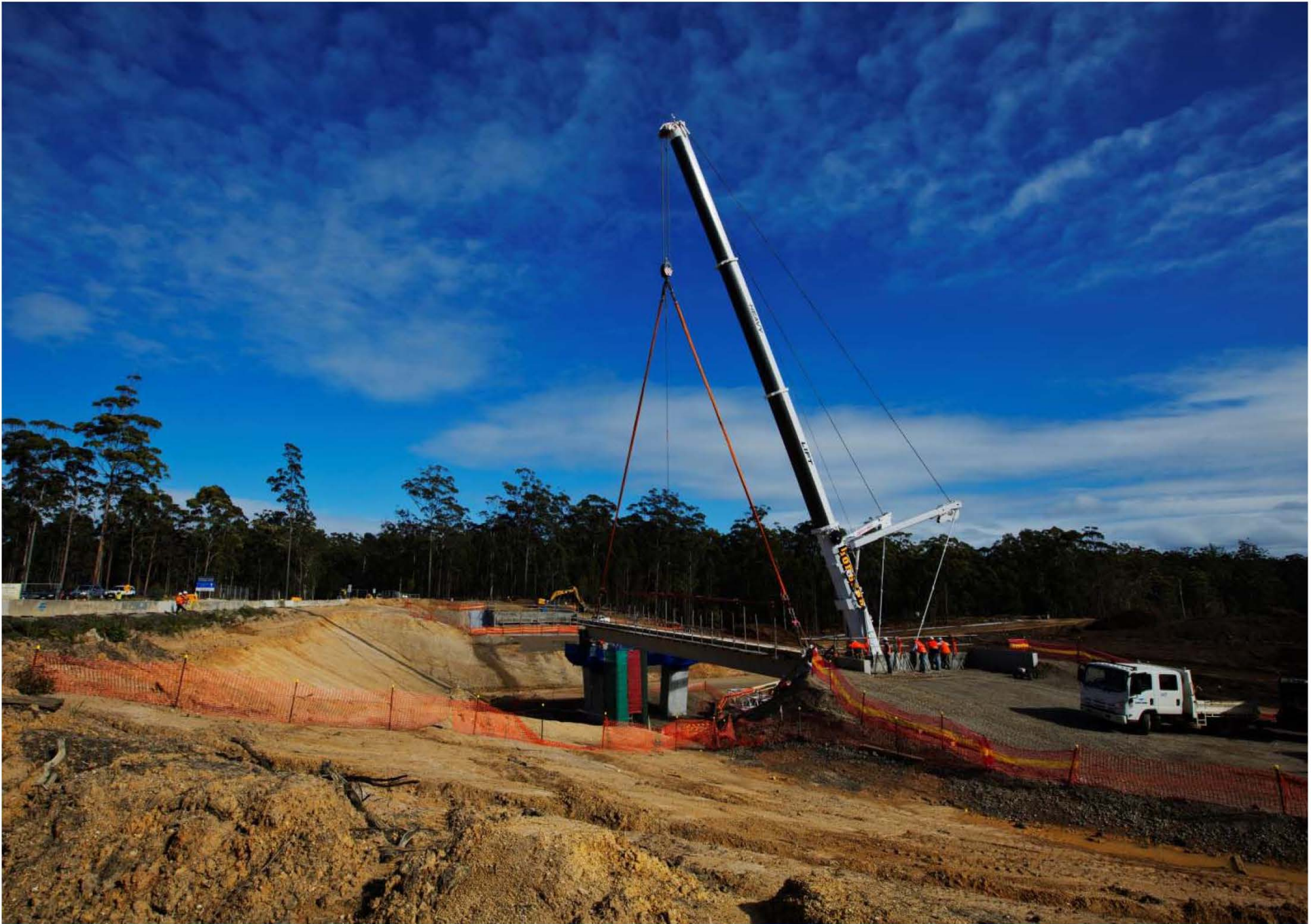
First girder placement at Ballards Road, August 2014- 14
