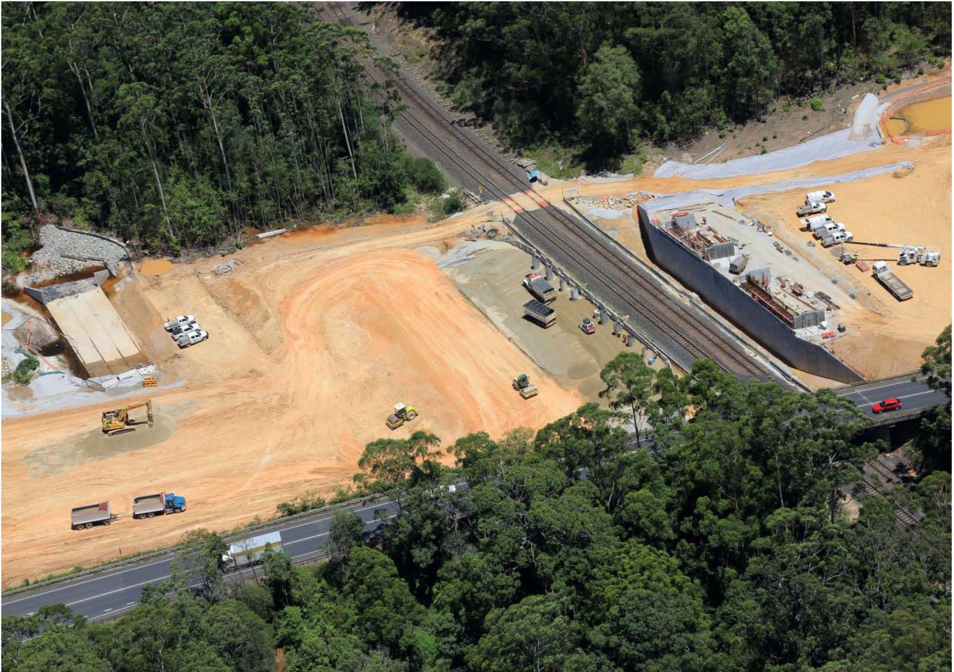
North Coast Rail bridge, January 2015
