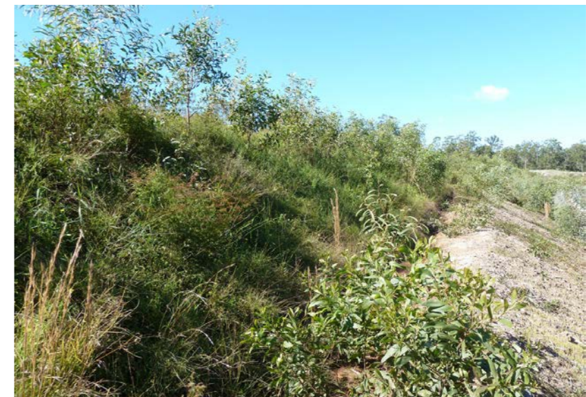
Excellent vegetation cover and species diversity resulting from topsoil management to preserve the soil seedbank at Pacific Highway Upgrade Glenugie. No Hydroseeding has been used on these embankments other than cover crop.
