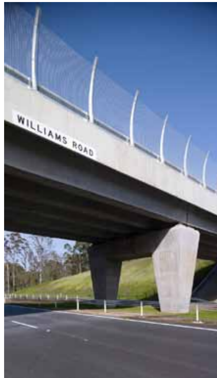
Bonville Overbridge Safety Screen and Pier Design
