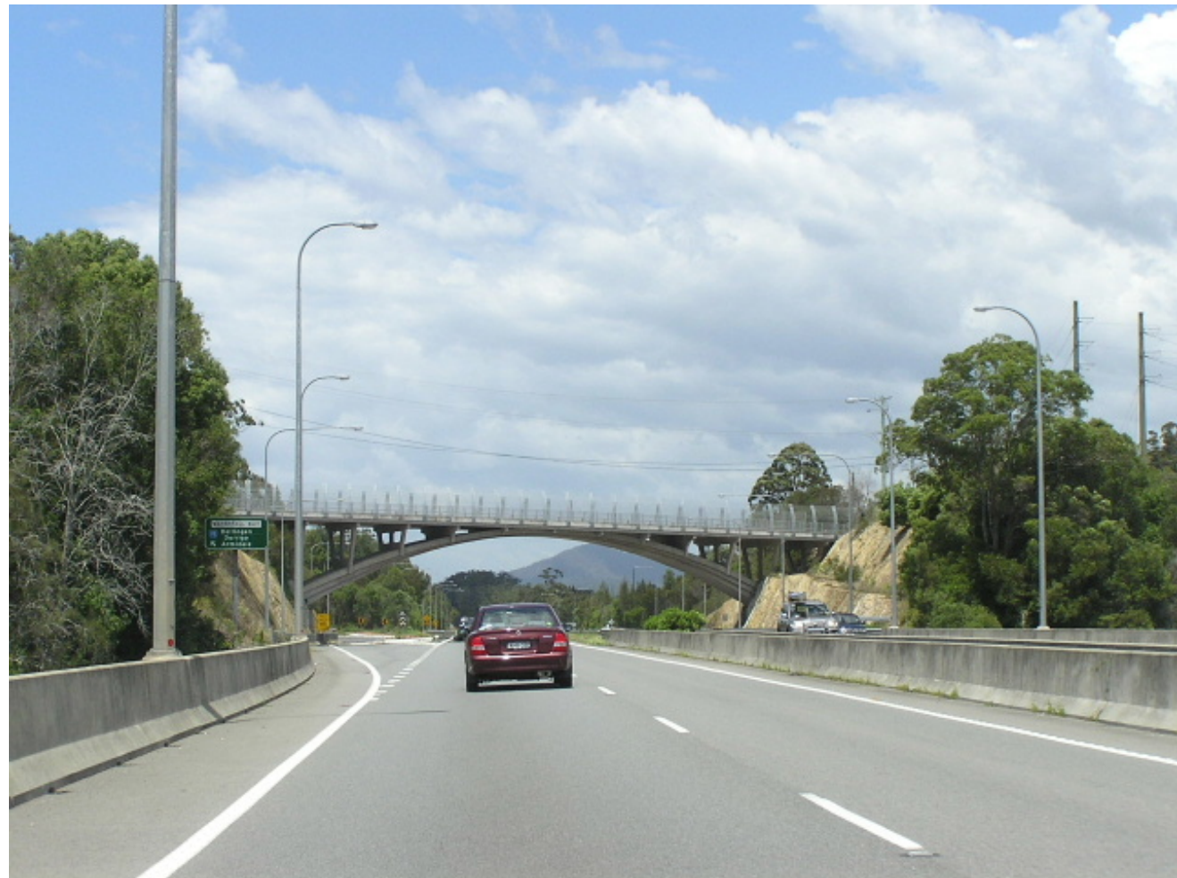
Looking south at the existing interchange with Waterfall Way
