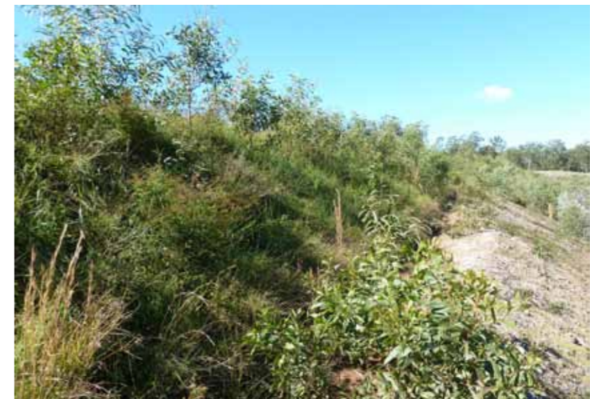
Excellent vegetation cover and species diversity resulting from topsoil management to preserve the soil seedbank at Pacific Highway Upgrade Glenugie. No Hydroseeding has been used on these embankments other than cover crop.
