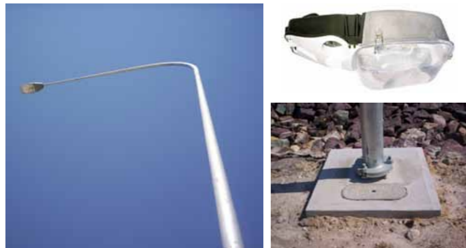
Roadway pole and outreach arm, luminaire and "slip base".
