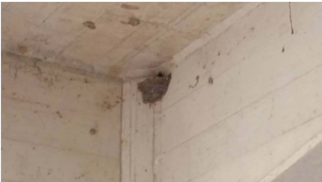
Plate 1-2. Micro bat suspected as Southern Myotis ( Myotis macropus ) inhabiting newly constructed swallow nests under the existing Pipers Creek Bridge.
