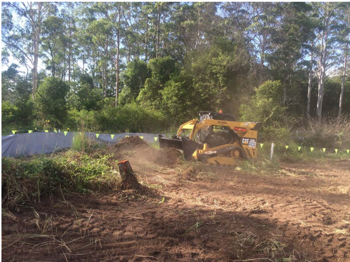
Plate 2: Stripping of vegetation in degraded giant barred frog habitat north of Cooperabung Creek on 24 November 2014.
