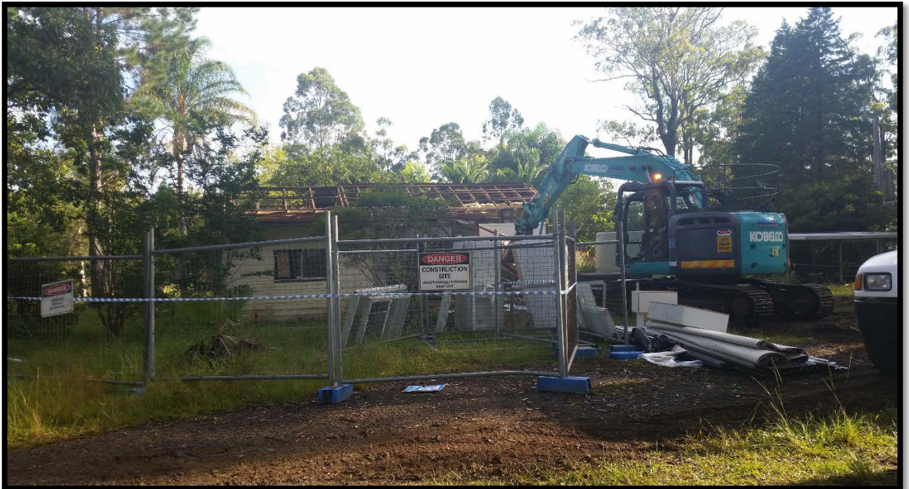
Plate 2-3. House being dismantled near Rodeo Drive was subject to micro bat inspections and works supervision.
