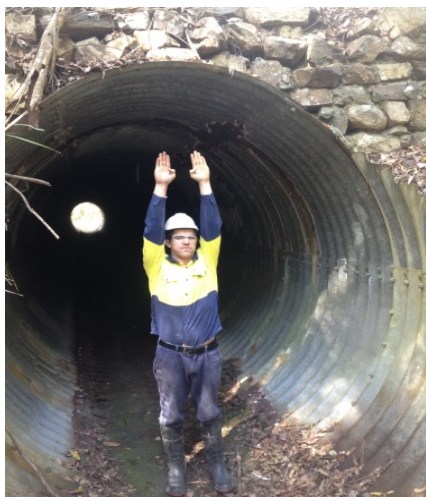
Plate 3. C599022 (chainage 22200) features 2x 3000mm galvanised pipes. The structure is likely a major microbat flyway and would present an entanglement hazard if curtained.
