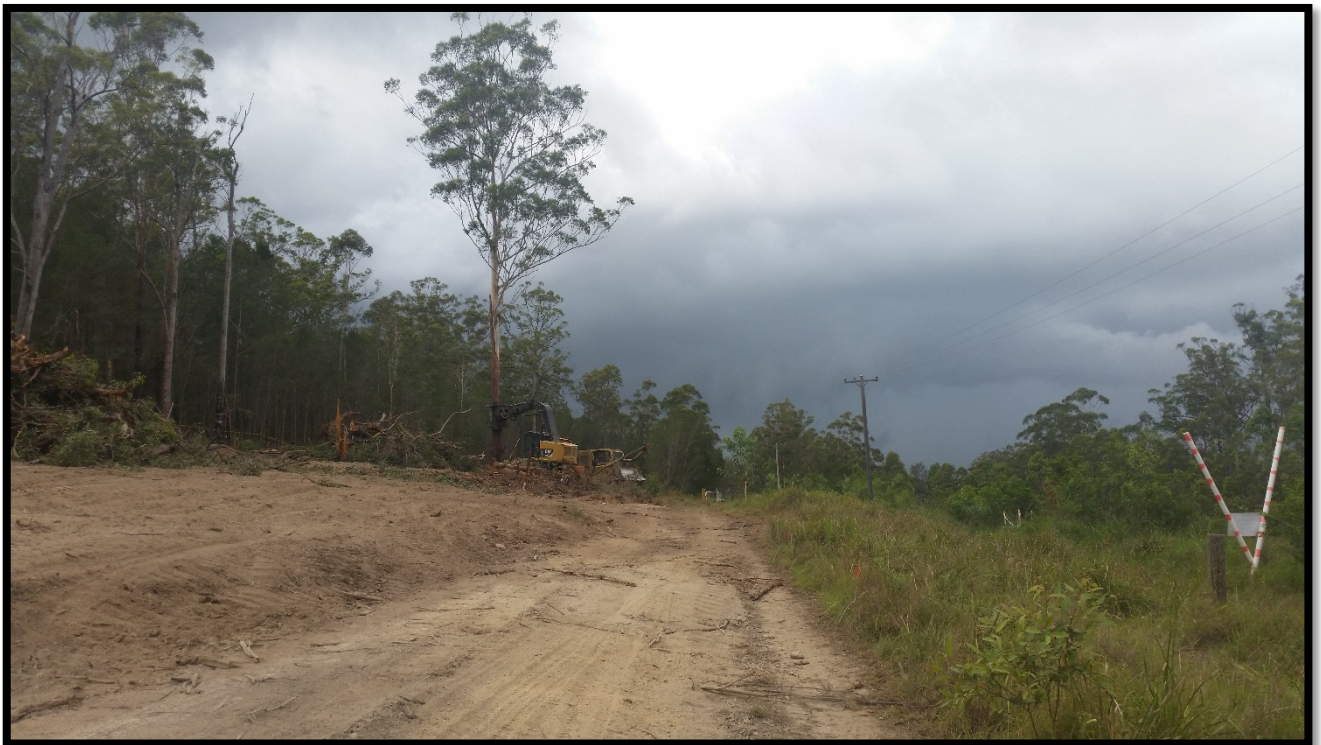
Plate 2-4. Clearing of habitat tree using harvester and dozer at ch. 33100.
