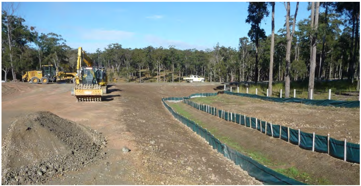
Topsoil application to final surface drainage infrastructure (St 1)
