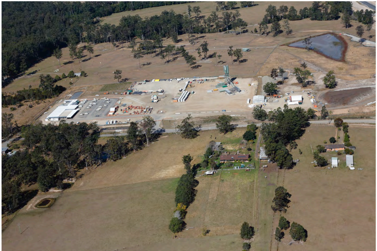
View of Stage 2 main construction compound, Kundabung (St 2)
