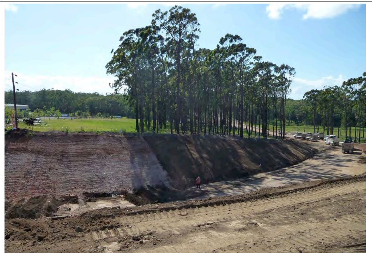
Placement of topsoil on Cut 1 batters – 5 February 2015 (St 1)
