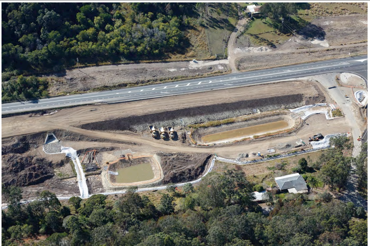
View of water quality control infrastructure and clear water drainage south of Cooperabung Creek (St 2)
