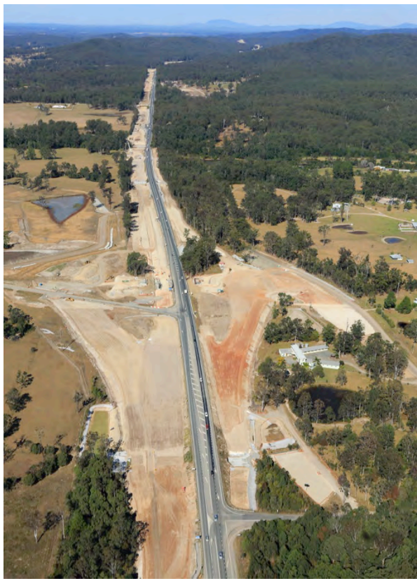
View south along alignment of the Kundabung interchange, Kundabung (St 2)
