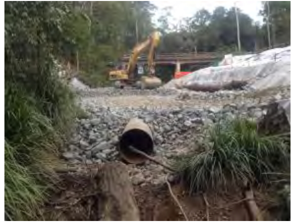
Piling pad installation Pipers Creek (St 2)
