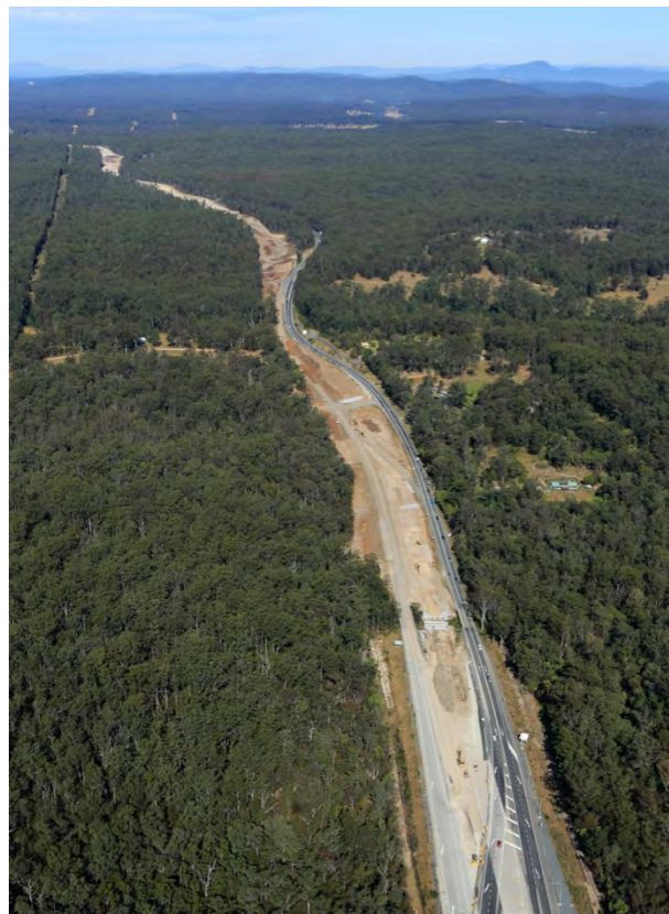
View south along alignment from the Kempsey Bypass tie-in (St 2)
