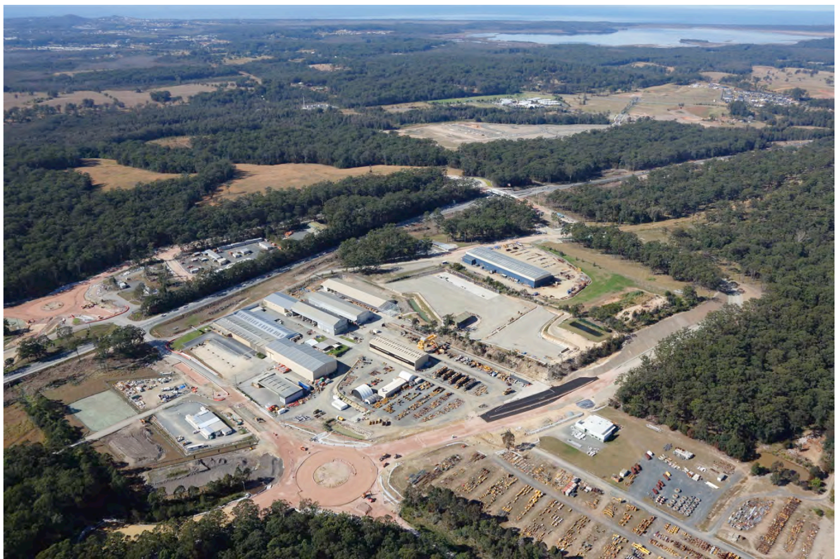
View southeast of Sancrox Traffic Arrangement works (St 1)
