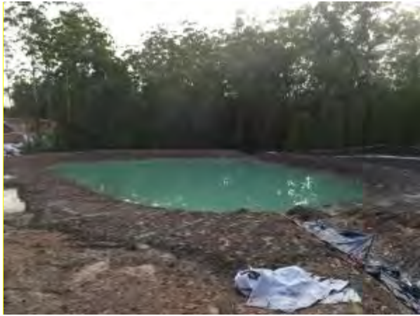
Permanent sediment basin (St 2)
