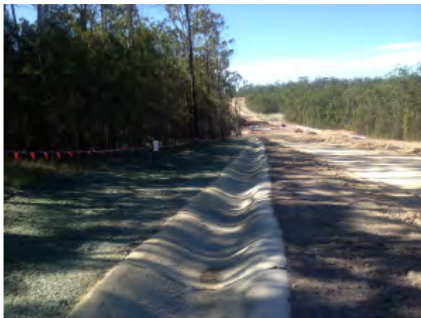
Clean water catch drain with hydromulch (St 2)
