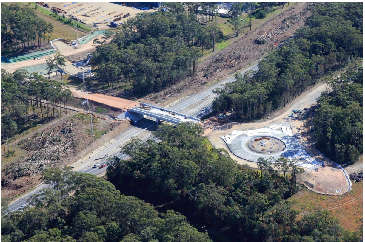
View northwest of new bridge over the existing Pacific Highway (St 1)
