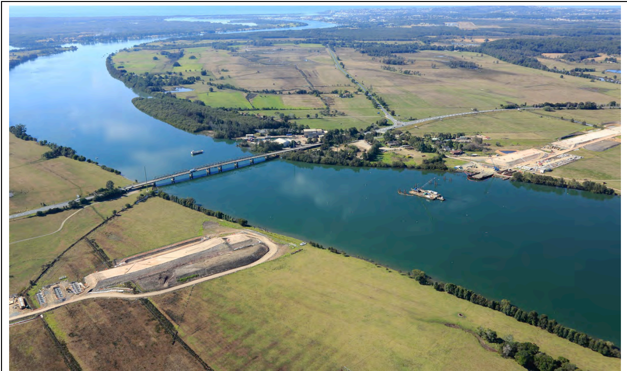
View east of alignment as it crossed over the Hastings River (St 3)
