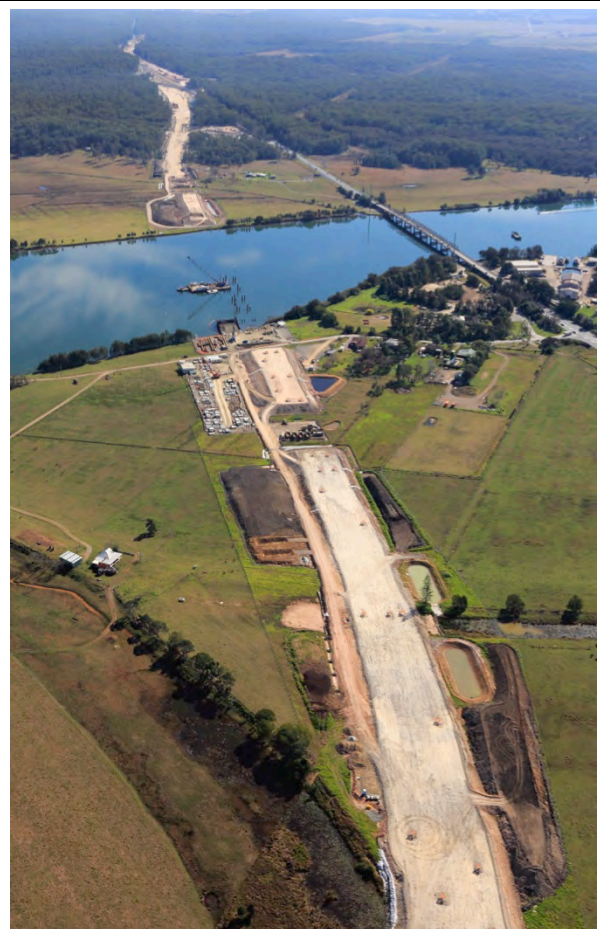
View north along alignment toward the Hastings River (St 3)
