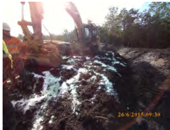
Addition of mulch ameliorants for mixing with topsoil – urea, sulfate of iron and lime (St 2)
