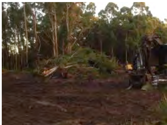
Bunding of timber immediately after clearing to manage tannins (St 2)
