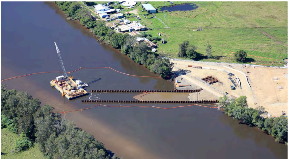
Silt curtains in place around temporary working platform works (St 3)
