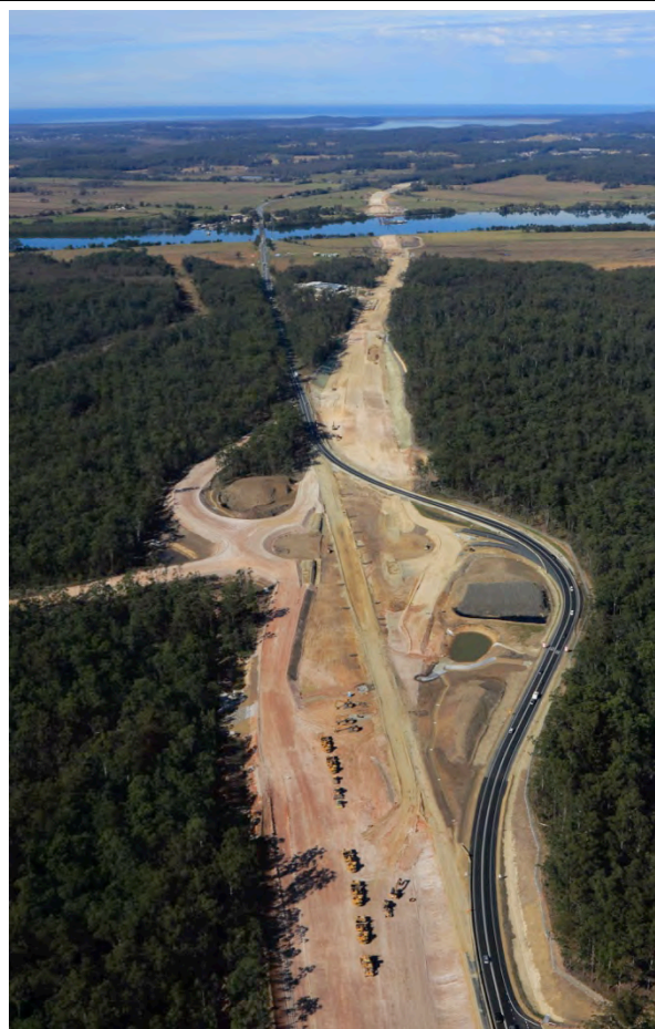
View looking south at the Blackmans Point Interchange (St 2)
