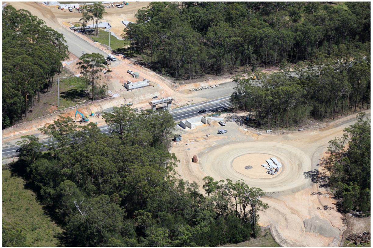
View west of new bridge over the existing Pacific Highway (St 1)
