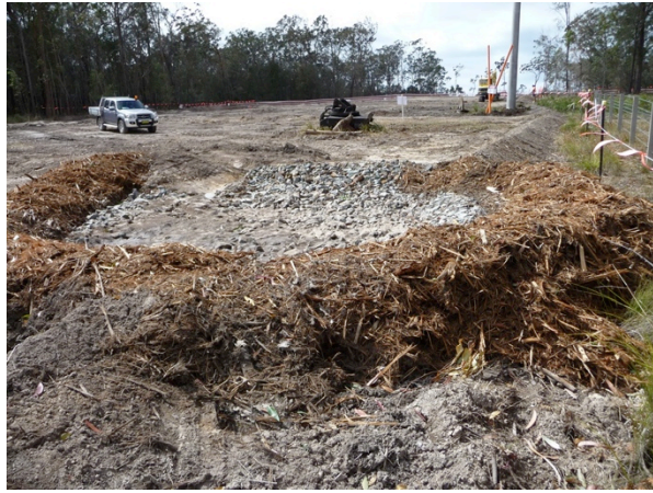
Mulch traps used along Service Road 3 as a sediment control measure (St 1)
