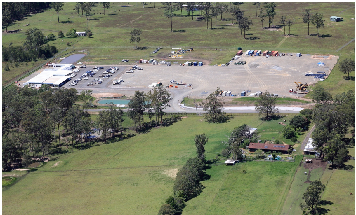
View of Stage 2 main compound of Kundabung Road (St 2)
