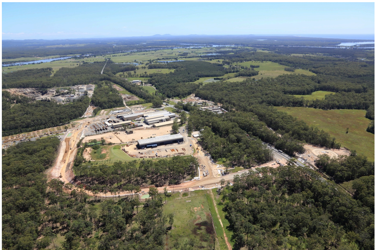
View north of Sancrox Traffic Arrangement works (St 1)
