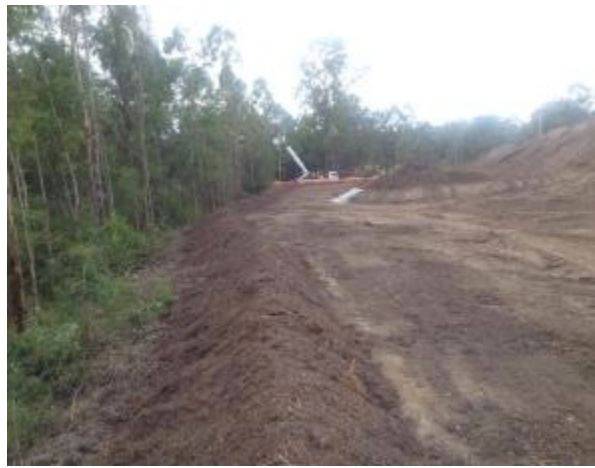
Mulch bunding in foreground. Bunding of mulch stockpile with spillway in background (St 2)
