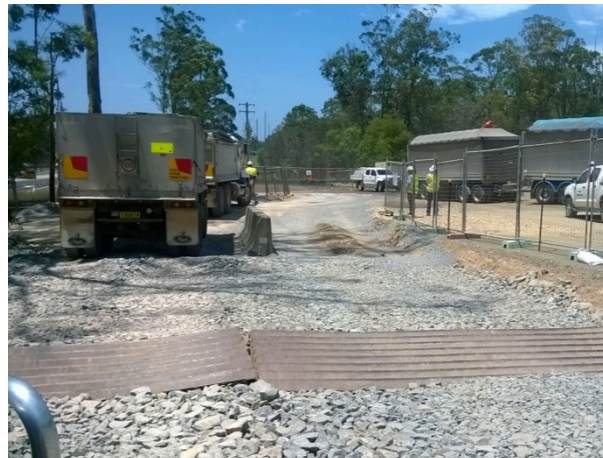
Rumble grid and rock access point to Ancillary Site 3 stockpile (St 1)
