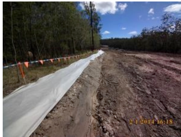
Upslope clean water diversion and clearing limit flagging delineation (St 2)
