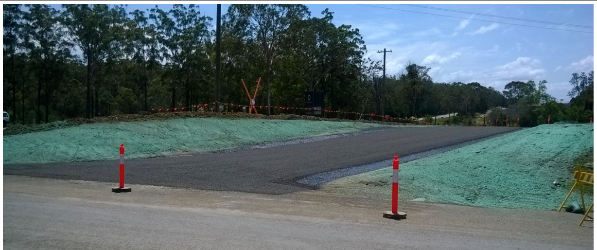
Hydromulching of batters along Cassegrains Winery temporary access (St 1)
