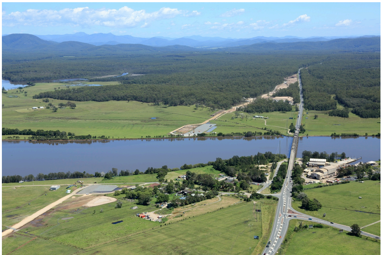
View north along alignment over the Hastings River (St 3)
