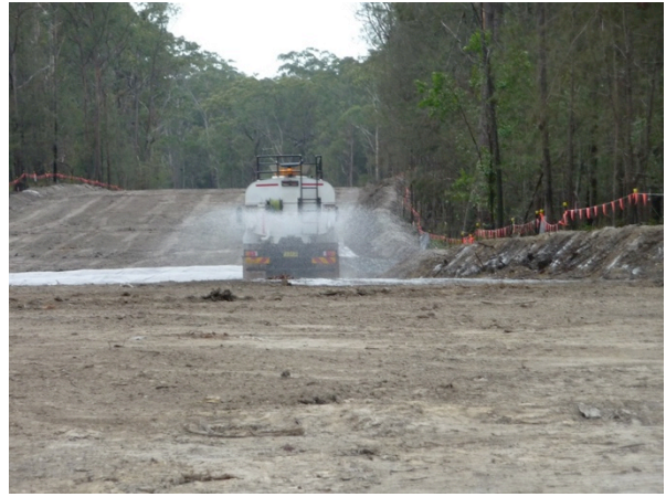
Stage 1: Dust suppression in progress on Service Road 3 (St 1)
