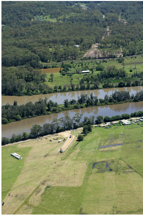
View north of Wilsons River along alignment (St 3)
