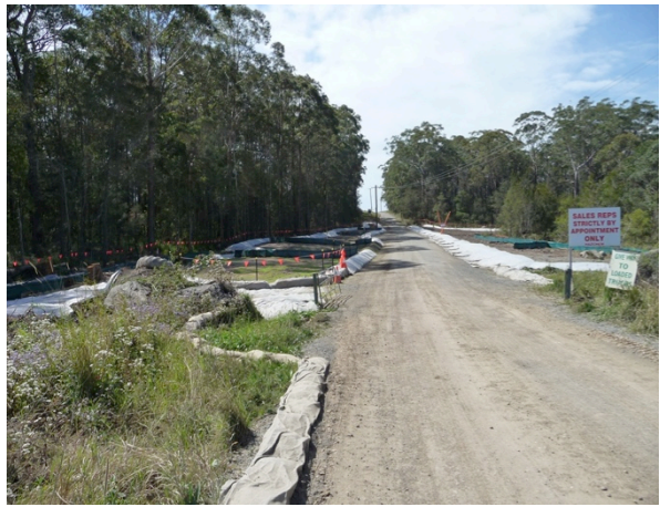
Erosion and sediment controls on Hansons Quarry Road (St 1)
