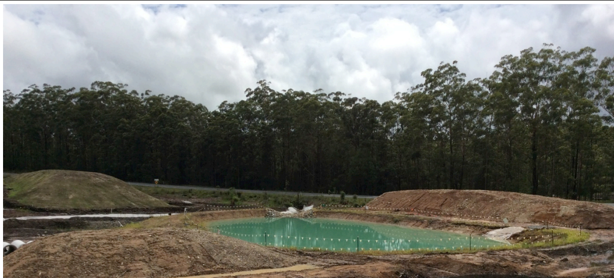
Water quality basin (St 3)
