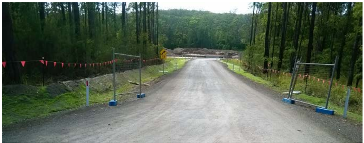
Revegetation of the shoulders on temporary quarry access track (St 1)
