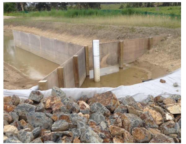
Sediment basin with baffle boards to increase sediment settling time (St 2)
