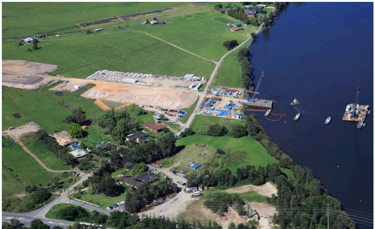
View of southern approach to the Hastings River crossing (St 3)
