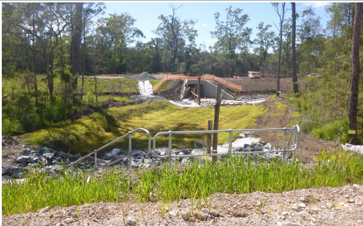
Widened median with fauna connectivity between shared water/fauna culverts (St 3)
