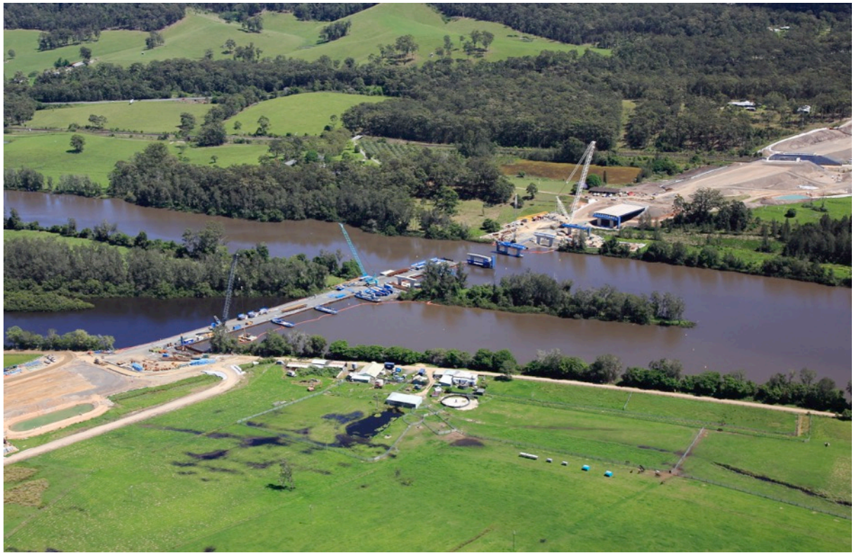
View north of Wilsons River crossing (St 3)
