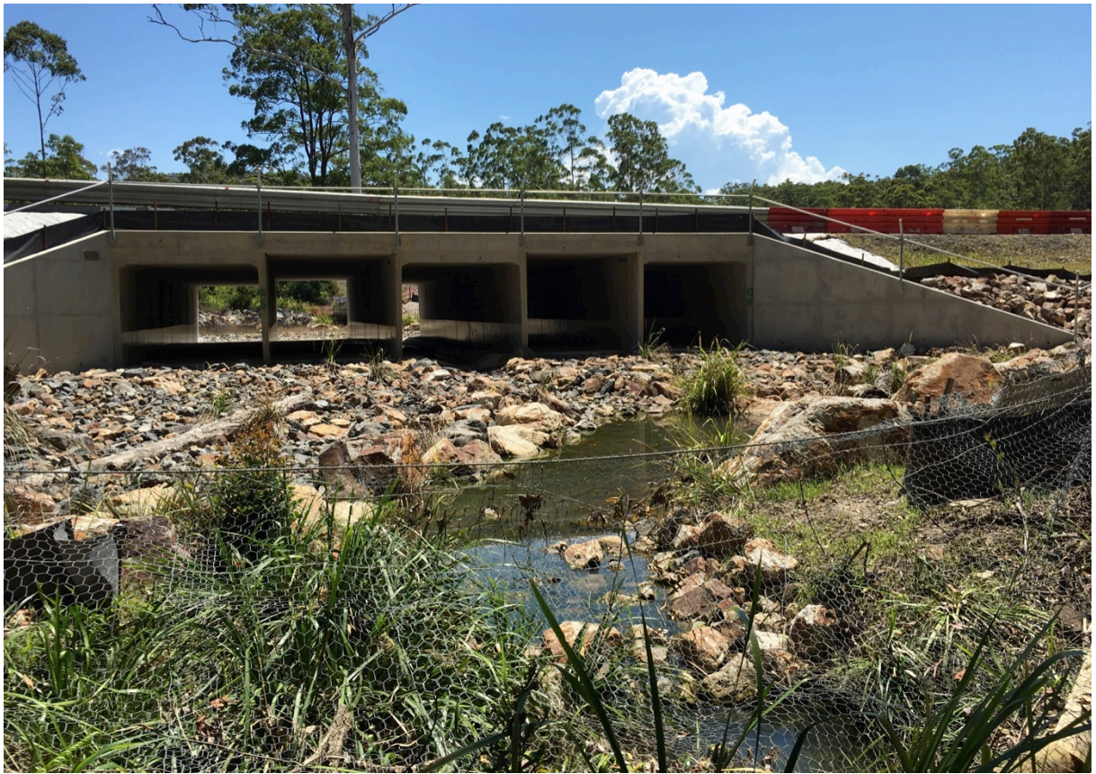
Barrys Creek waterway and culvert restoration (St 2)
