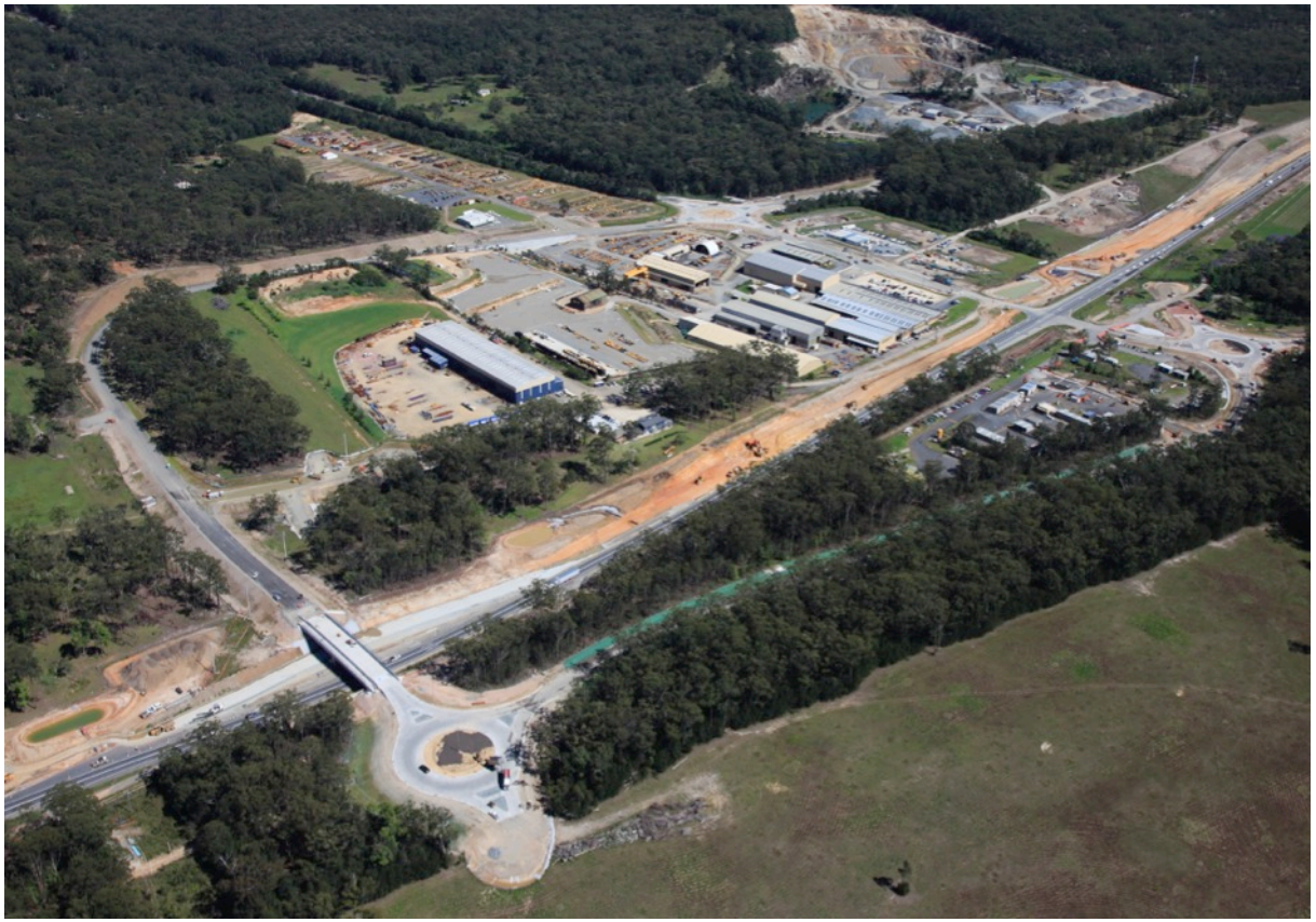
View northwest of Sancrox Traffic Arrangement works (St 1)
