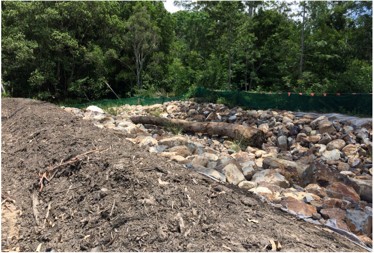
Finish treatment of drainage line near Smiths Creek (St 2)
