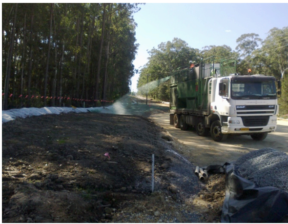
Hydromulching on Service Road 2 (St 1)
