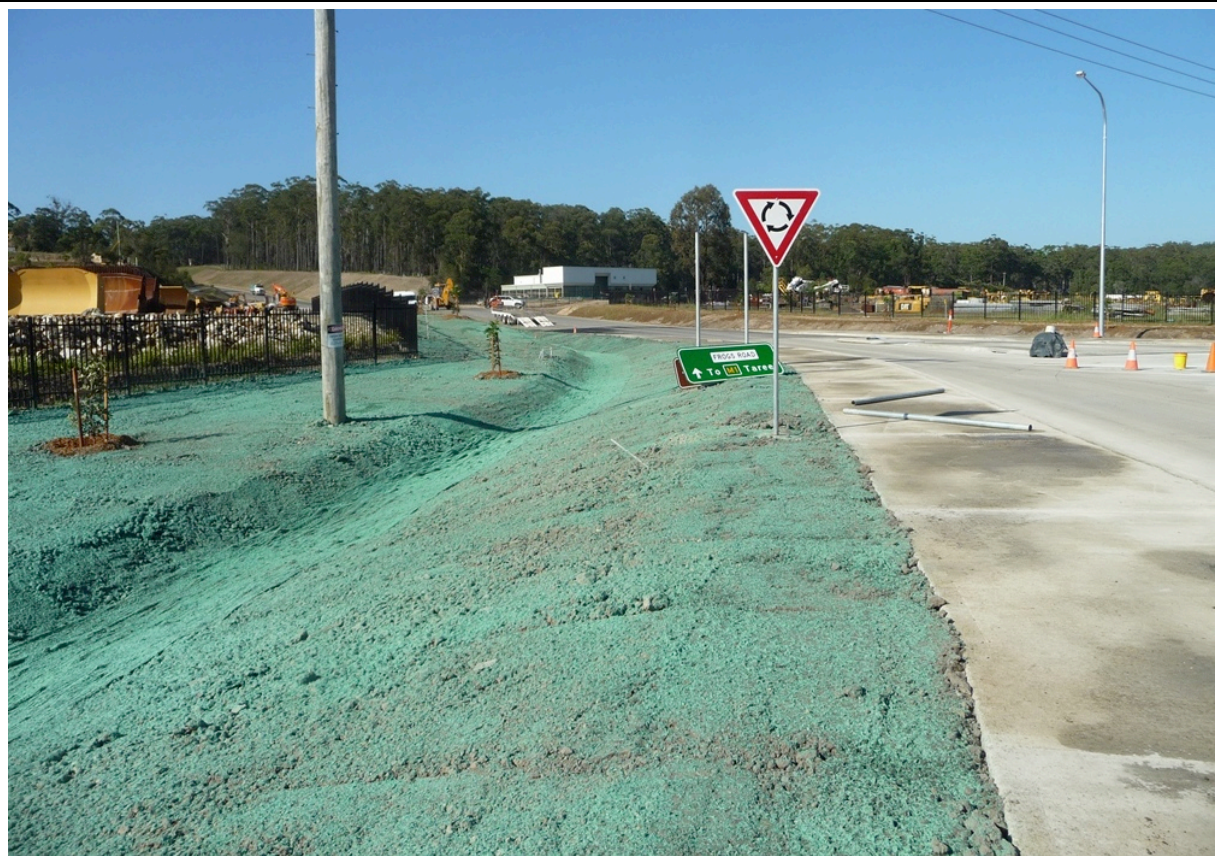
Service Road 1 following the application of hydromulch (St 1).
