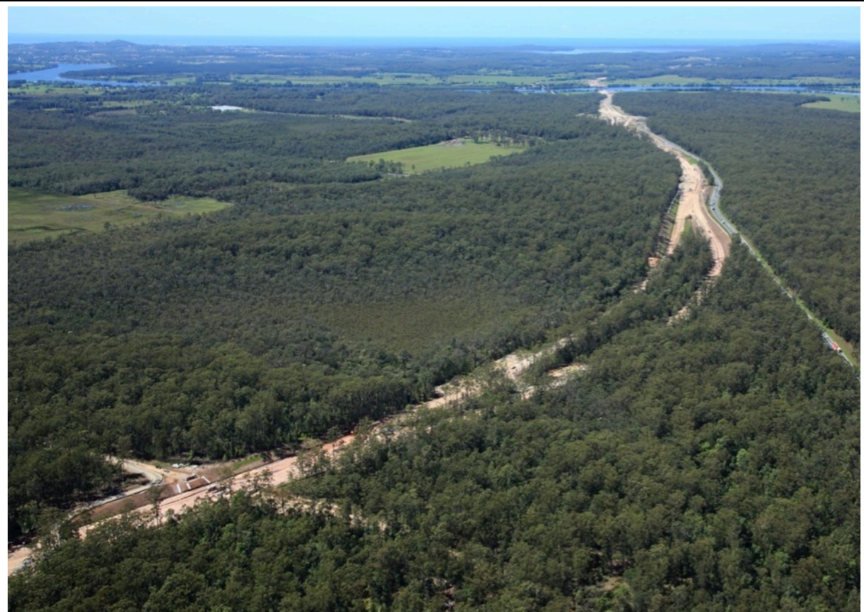
View south from about Bill Hill Road toward the Hastings River (St 3)
