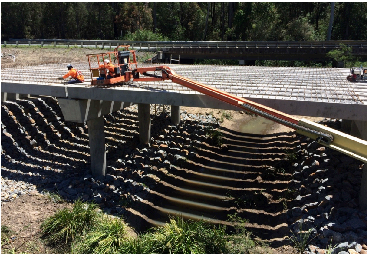
Restoration of Smiths Creek under the new northbound bridge (St 2)
