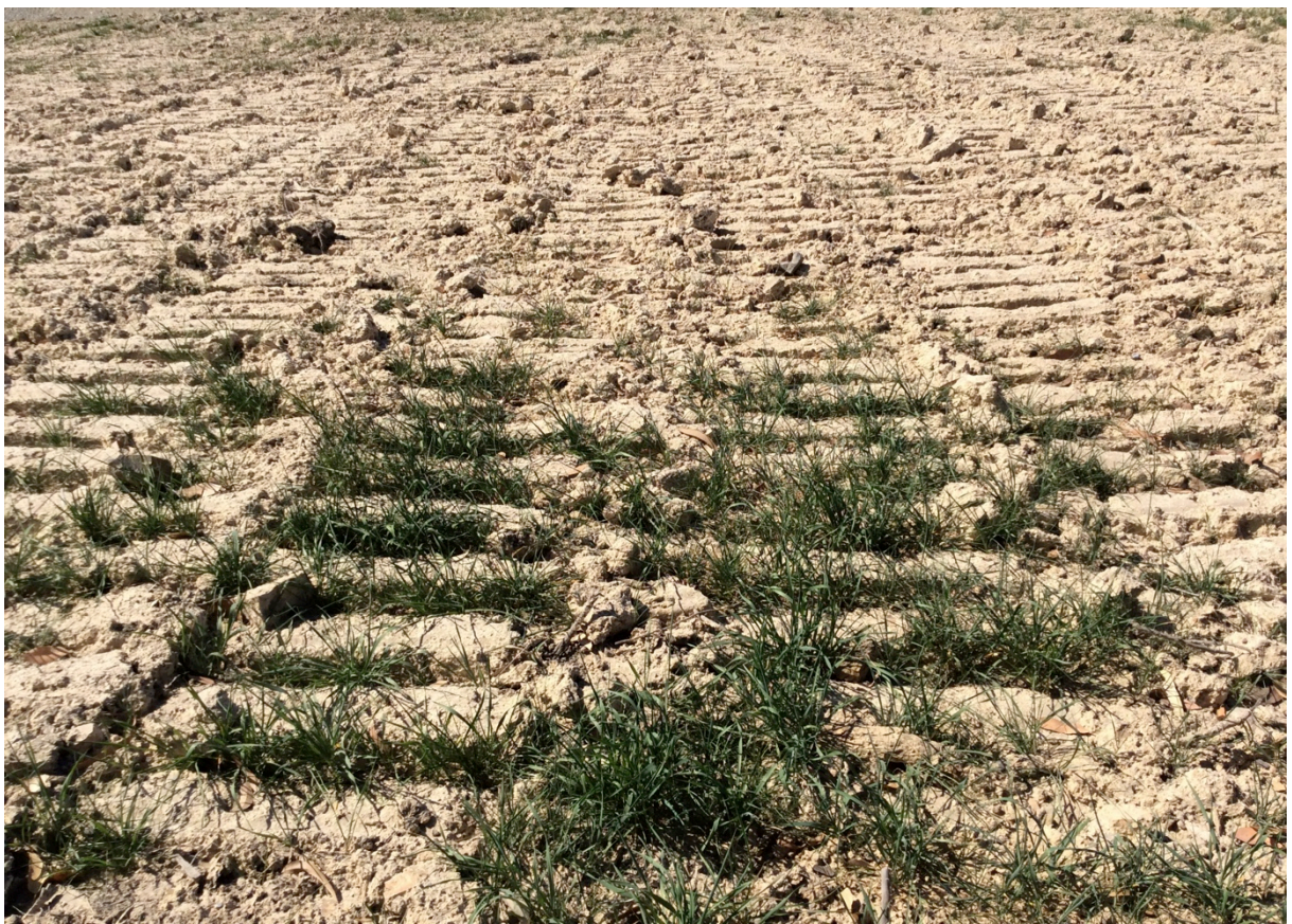
Batter preparation for revegetation (St 3)
