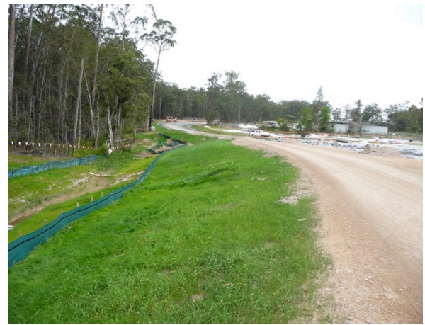
Stabilisation of drainage line on North Eastern Roundabout (St 1)
