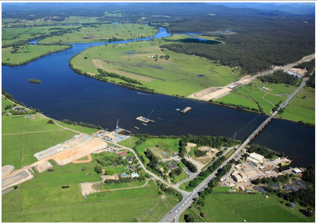
View north of the Hastings River crossing (St 3)
