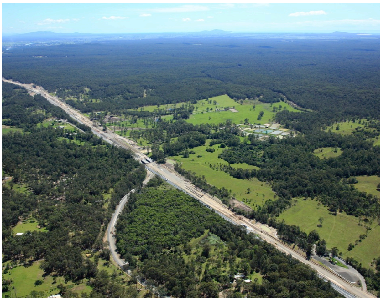
View south along alignment of Pipers Creek (St 2)
