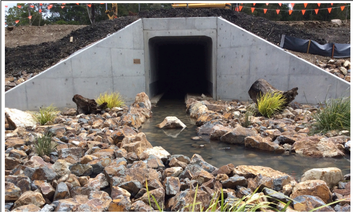
Finishing works and low flow treatment for fish passage (St 2)
