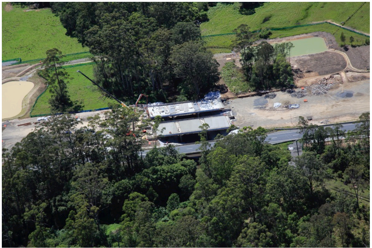
View of Pipers Creek crossing (St 2)
