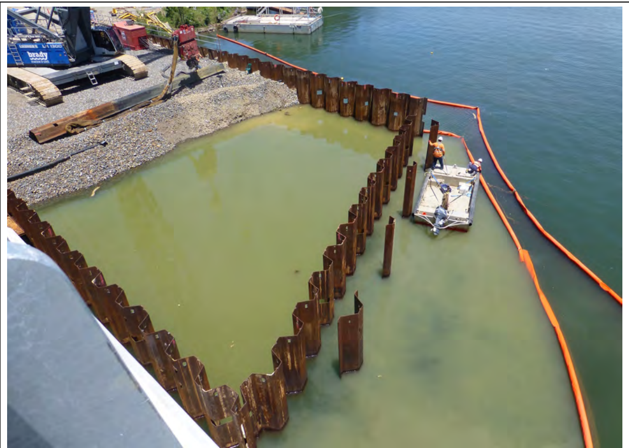
Sheet pile removal on Hastings River (St 3)
