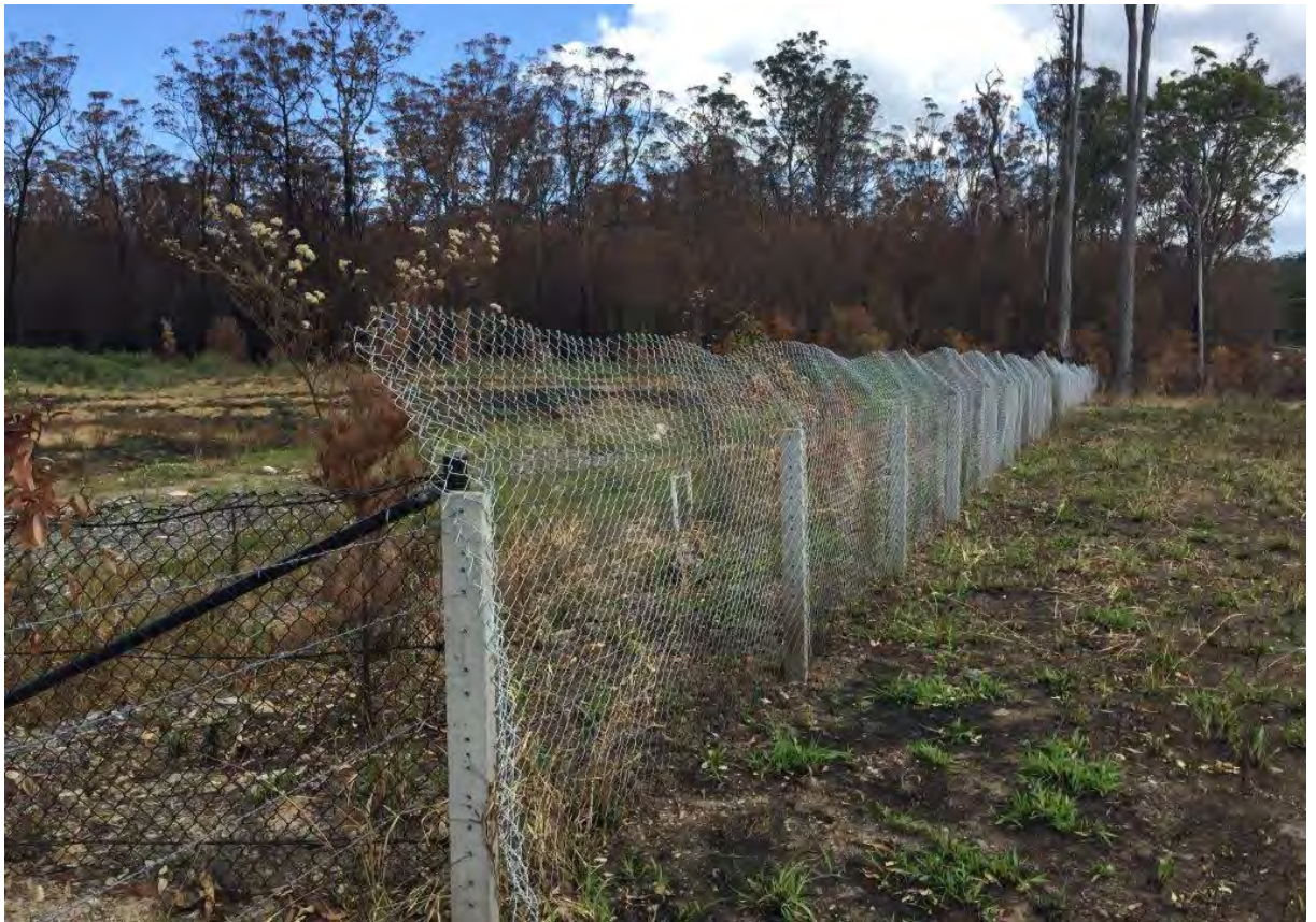
Retro-fitting fauna fence (St 2)
