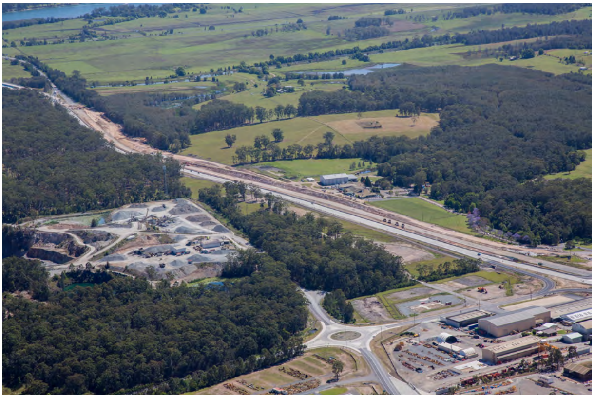
View north along main alignment beyond Stage 1 traffic arrangement works (St 3)
