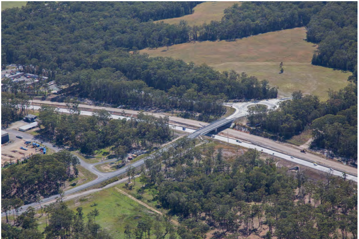
View east of main alignment through Stage 1 traffic arrangement works (St 3)
