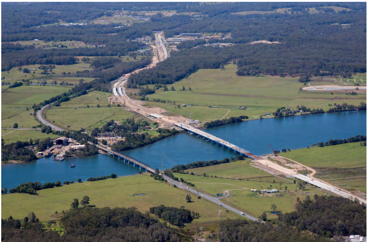
View of Hastings River crossing looking south along alignment (St 3)
