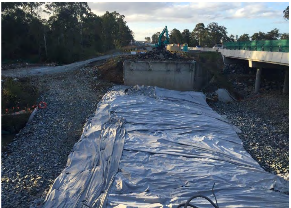
Controls in place during Smiths Creek northbound bridge demolition (St 2)
