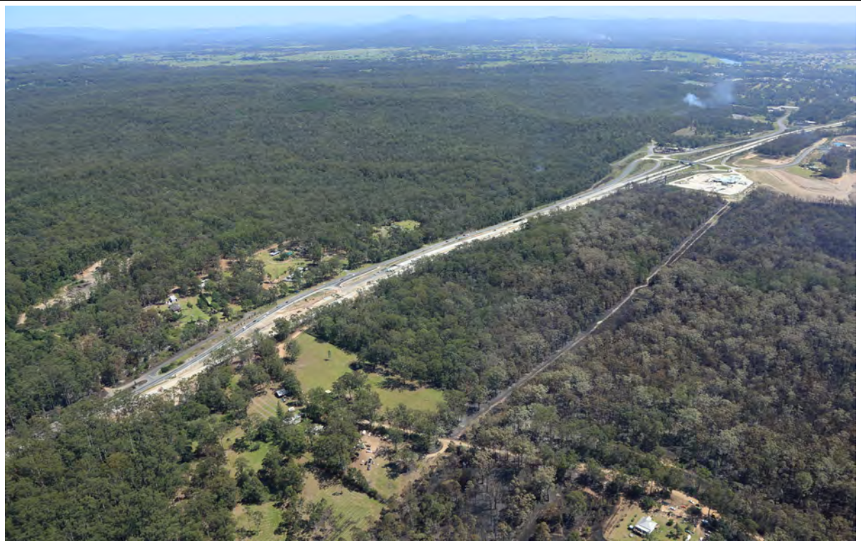
View north toward tie-in to Kempsey bypass (St 2)
