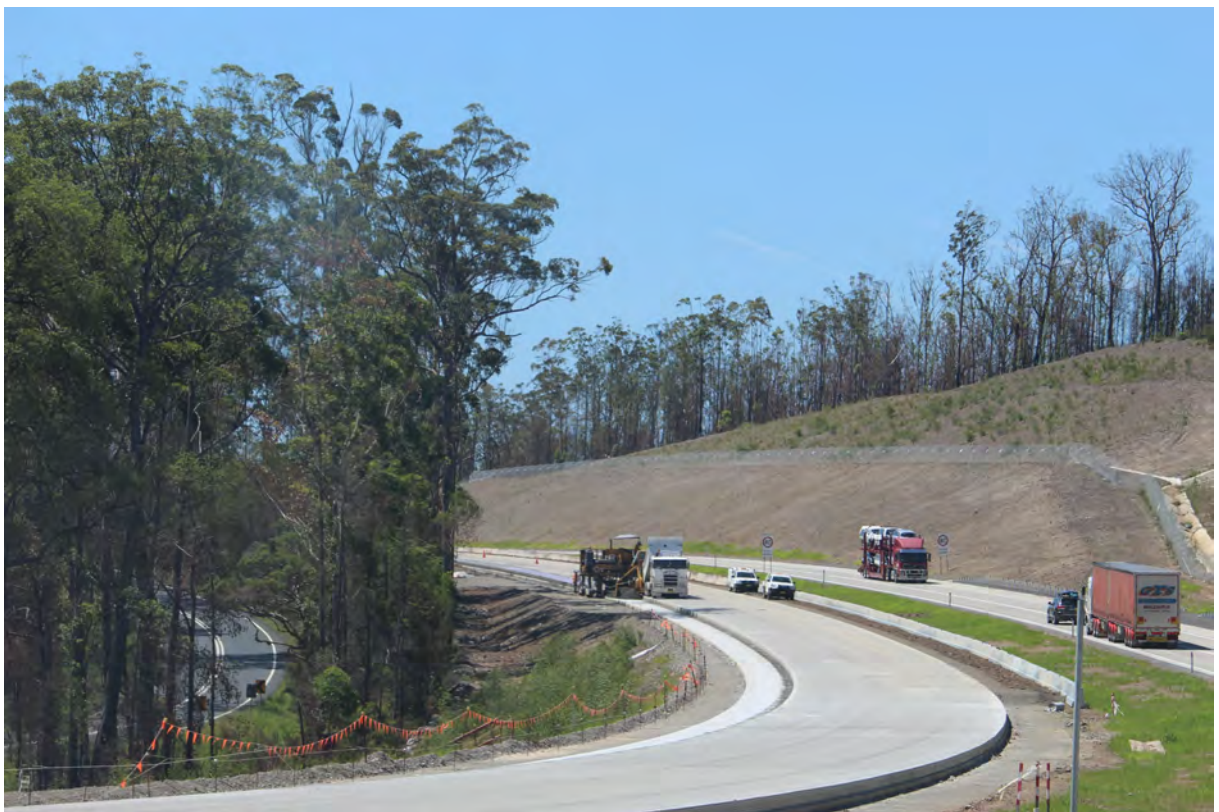
Topsoil application and landscaping on deep cut (St 2)
