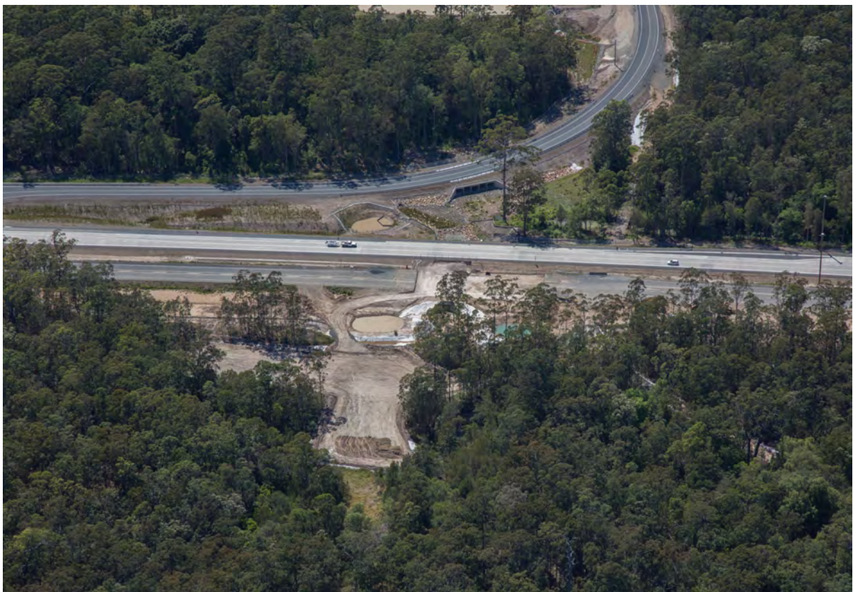
View of Barrys Creek at Mingaletta Road looking east (St 2)
