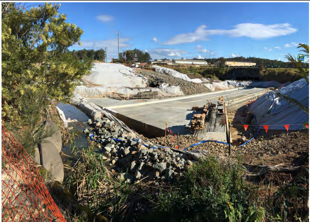
Clean water diversion at Fernbank Creek tributary during culvert construction (St 3)
