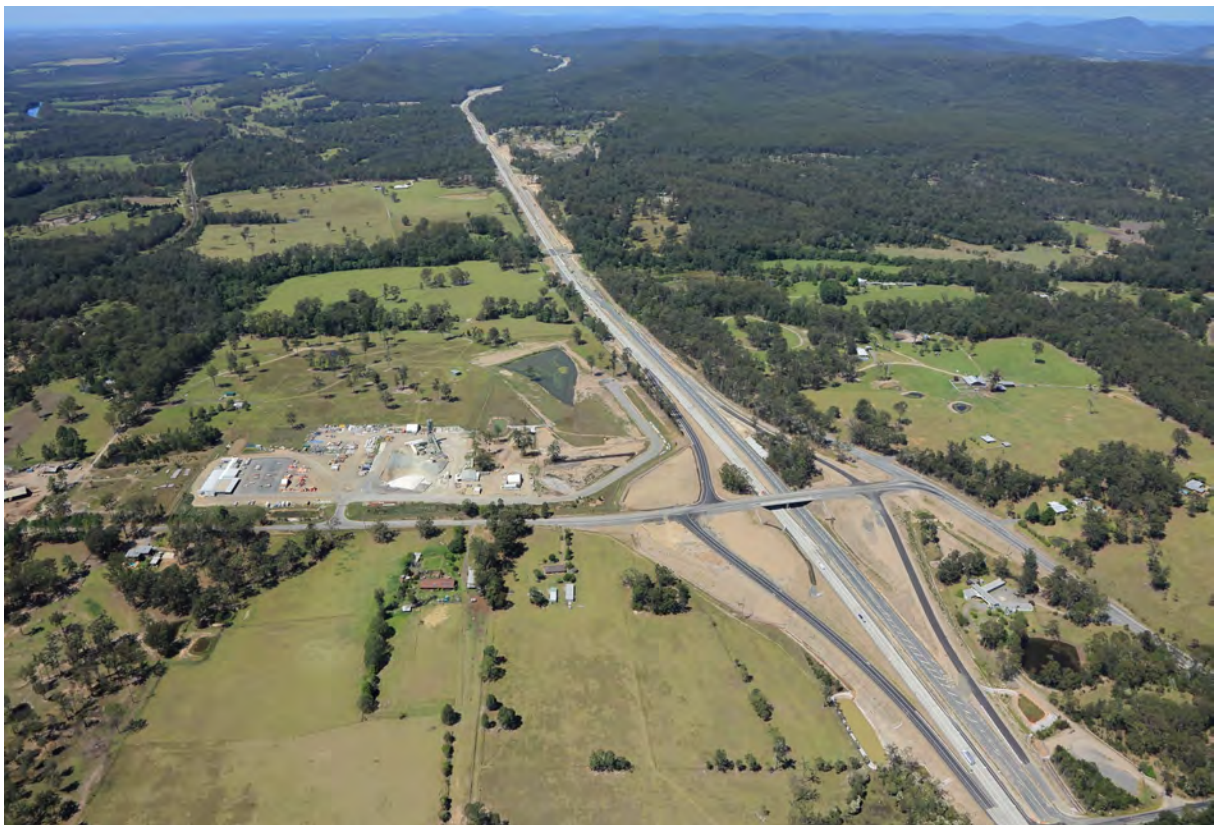
View of main compound and Kundabung interchange looking south (St 2)
