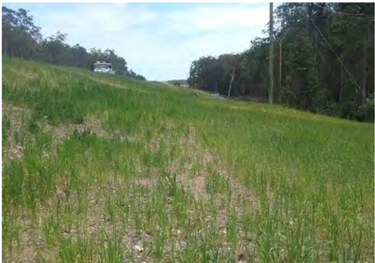
Rehabilitation of decommissioned water quality basin and adjacent earthworks formation (St 3)
