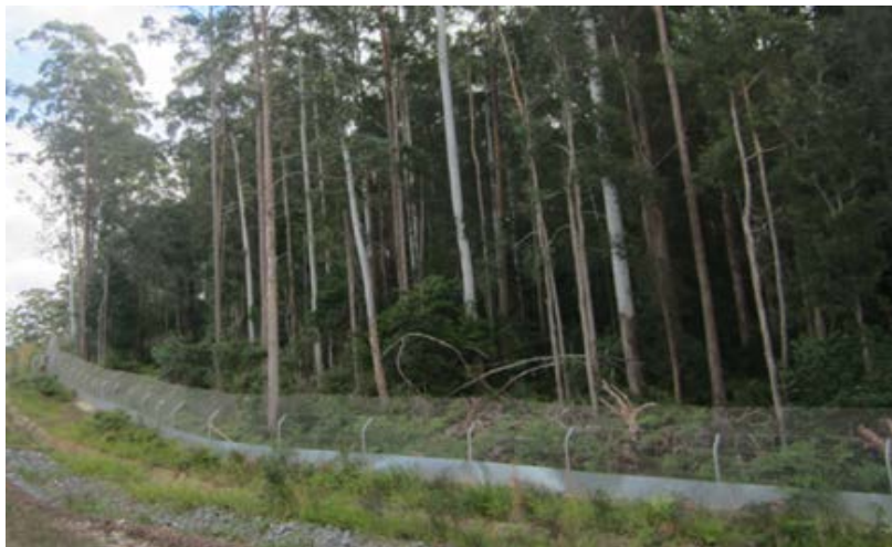
Figure 17 Fauna fencing, Oxley Highway (Source: SHJV)
