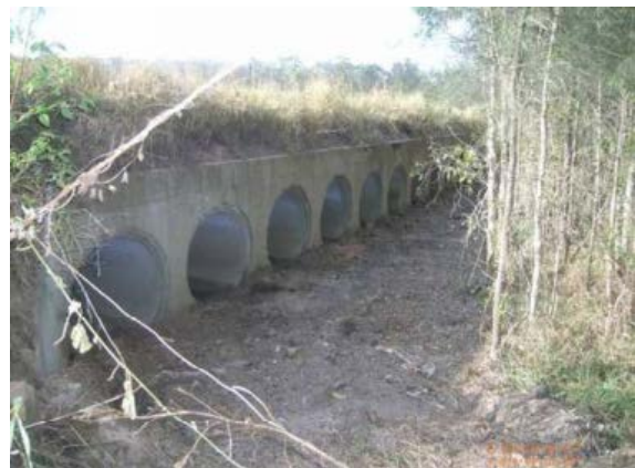
Figure 8 Incidental fauna underpass culvert, Pacific Highway upgrade (Source: RTA 2010)
