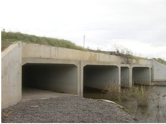
Figure 5 Combined fauna underpass culvert with dry cell for fauna passage, Pacific Highway upgrade (Source: RTA 2010)
