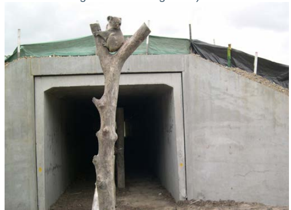
Figure 16 Koala using refuge pole at underpass entrance, Pacific Highway upgrade (Source: RTA 2010)
