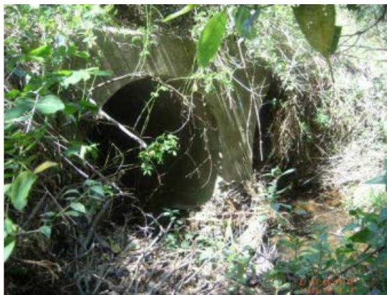
Figure 7 Incidental fauna underpass culvert, Pacific Highway upgrade (Source: RTA 2010)
