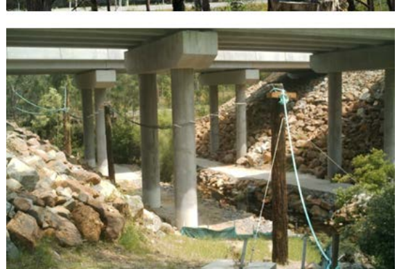
Figure 10 Rope bridge under dual carriage bridge, Pacific Highway upgrade (Source: RTA 2010)
