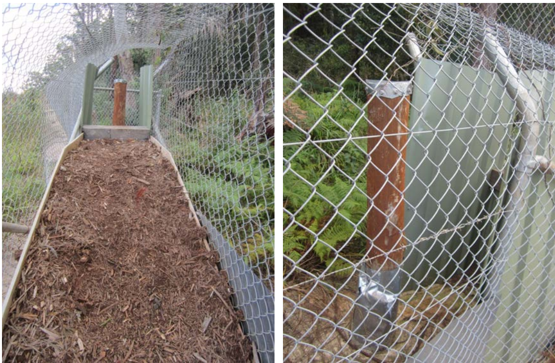
Figure 18 Example Fauna Drop Down Structure, Oxley Highway NSW. Left to Right: Compacted earth ramp and corrugated sheet metal tied to mesh fencing (Source: Hyder Consulting)
