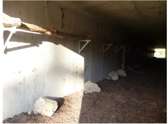
Figure 12 Bingis Lane dedicated culvert, Kempsey Bypass (Source: Lewis Ecological Consulting 2012)
