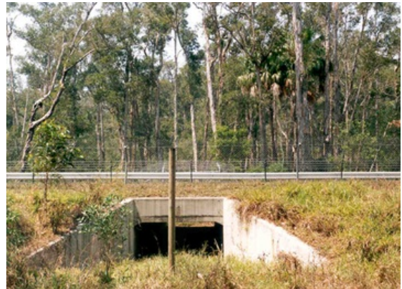
Figure 4 Dedicated fauna underpass, Pacific Highway upgrade (Source: RTA 2010)
