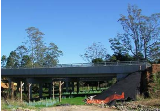
Figure 9 Koala poles under dual carriage bridge, Pacific Highway upgrade (Source: RTA 2010)
