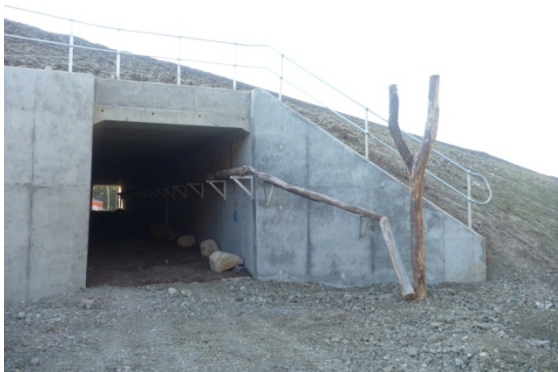
Figure 3 Bingis Lane dedicated culvert, Kempsey Bypass (Source: Lewis Ecological Consulting 2012)
