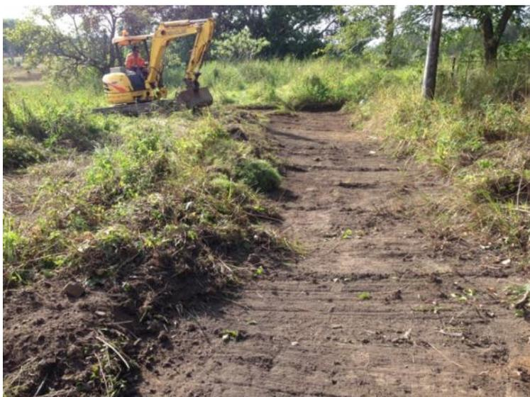
**Plate 2:** Area 1 (stripping topsoil); View E (Niche, 2014)
