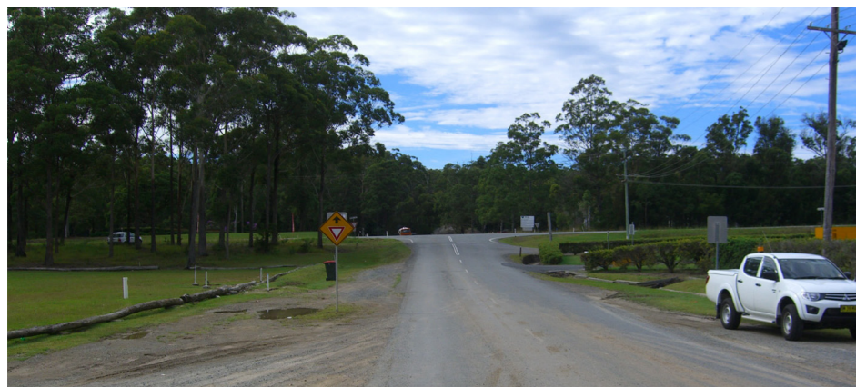
Looking east along Sancrox Road towards the existing Pacific Highway.
