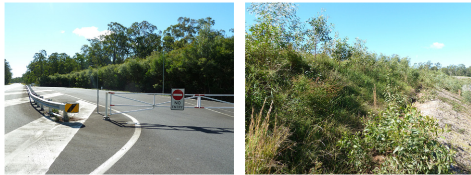
Photo to the left illustrates the few species established via hydromulching, while the photo to the right illustrates the diversity achieved through direct return of topsoil containing a soil seedbank. Glenugie Upgrade.
