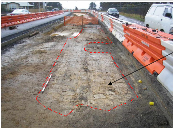
Figure 1: Telford road uncovered on the Great Western Highway (Leura) in 2008.
