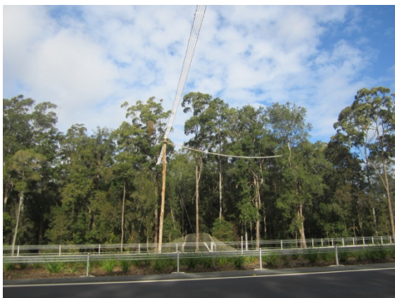
Figure 3: Rope bridge, Oxley Highway (Source: Laura Worthington, Hyder Consulting)
