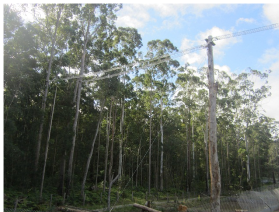
Figure 4: Rope bridge, Oxley Highway (Source: Laura Worthington, Hyder Consulting)
