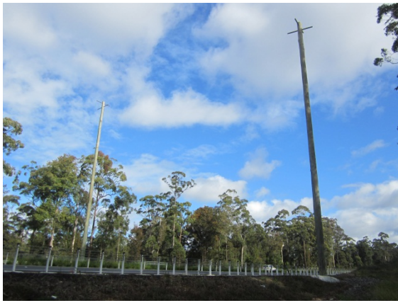
Figure 1: Example of glider poles at Oxley Highway (Source: Laura Worthington, Hyder Consulting)
