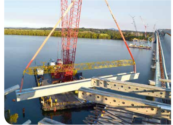
Last girder placement for the bridge
