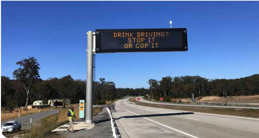
New Variable Message Sign for southbound traffic commissioned at Cooperabung
