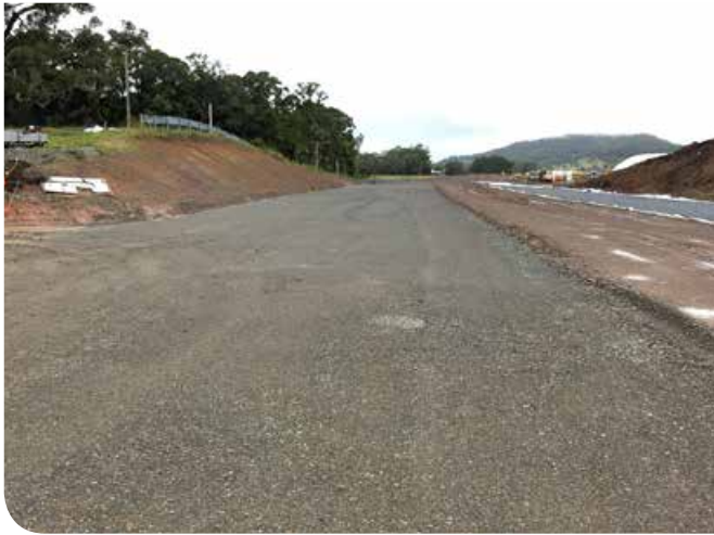
Foundation layer for paving at Wardell Road at Wardell
