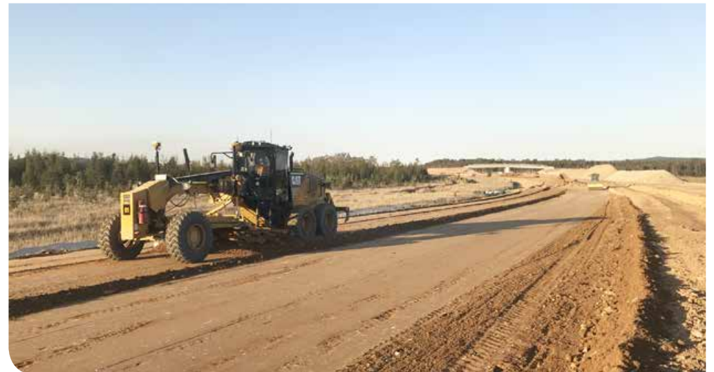
Foundation work for paving south of Byrons Lane at Tyndale
