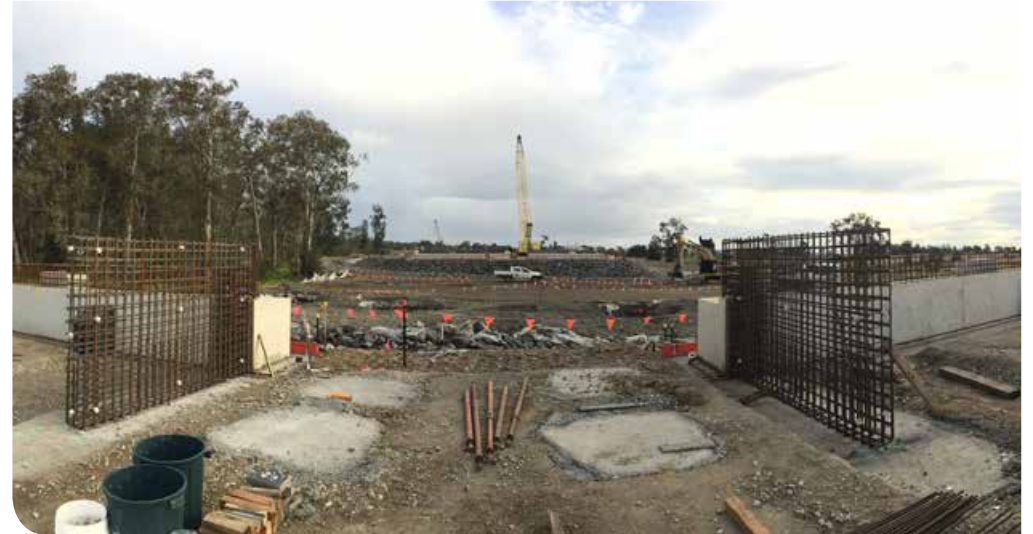
Building the bridge substructure near Watsons Street at Woodburn
