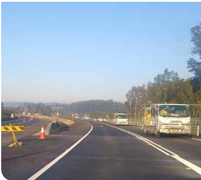
Traffic switch at Pimlico completed
