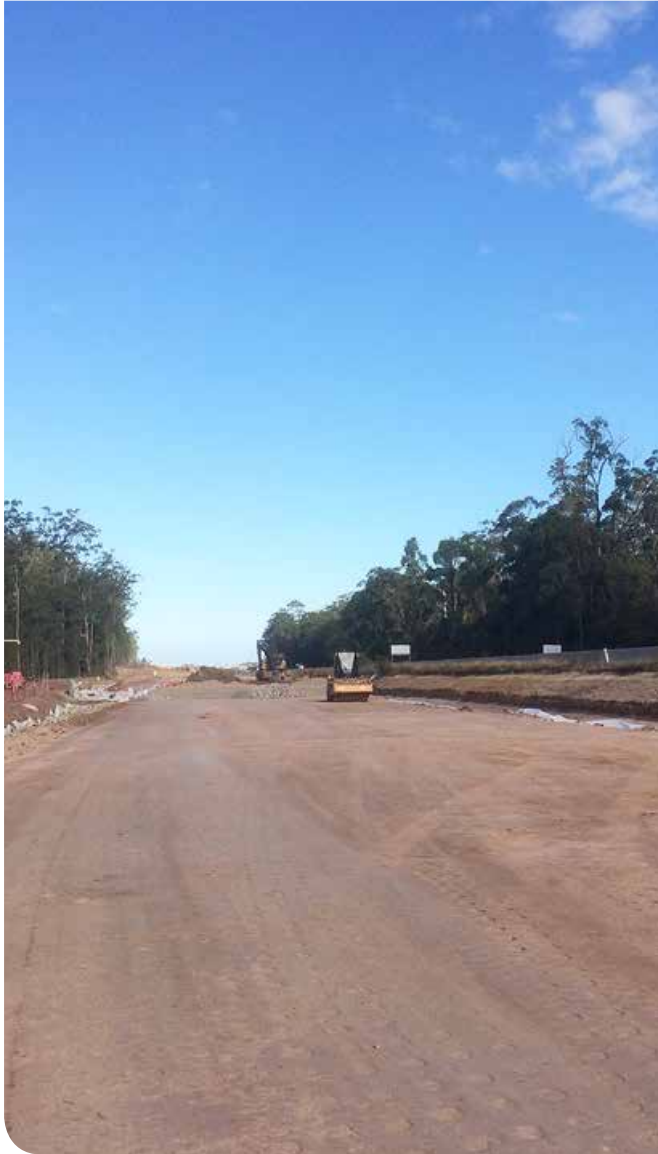
Foundation treatment for paving between Iluka Road and Devils Pulpit
