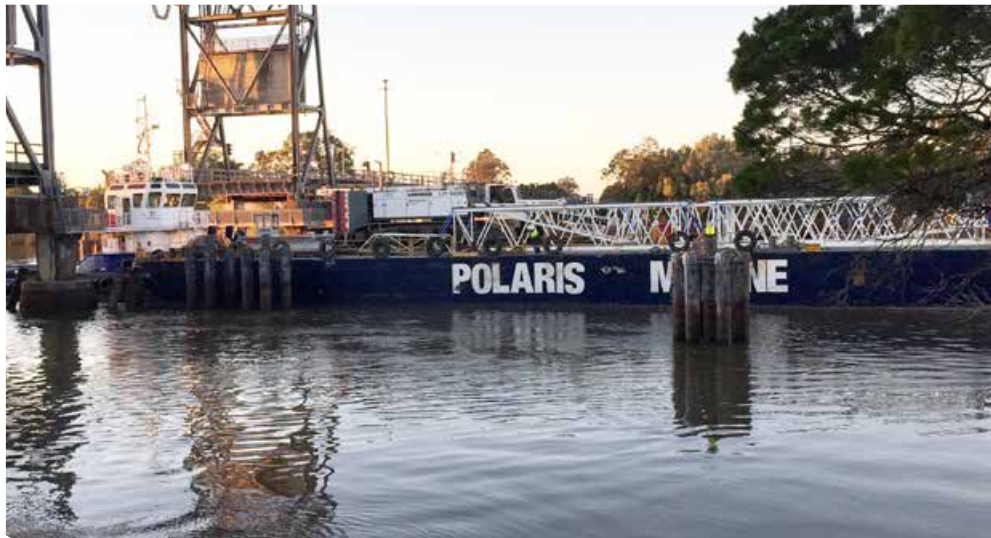
Barge travelling to site on the Richmond River for marine work
