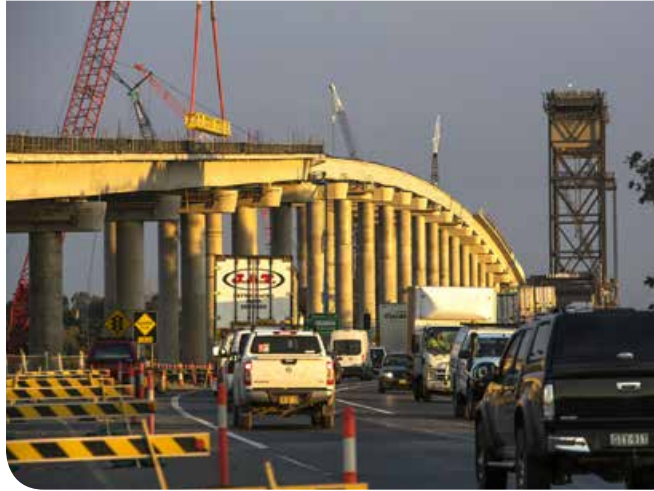
Installing transfloor panels on the bridge
