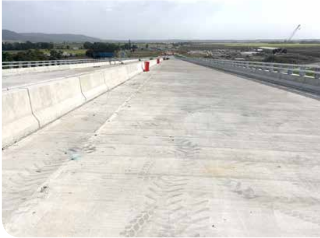
Northern landside parapet and bridge railing
