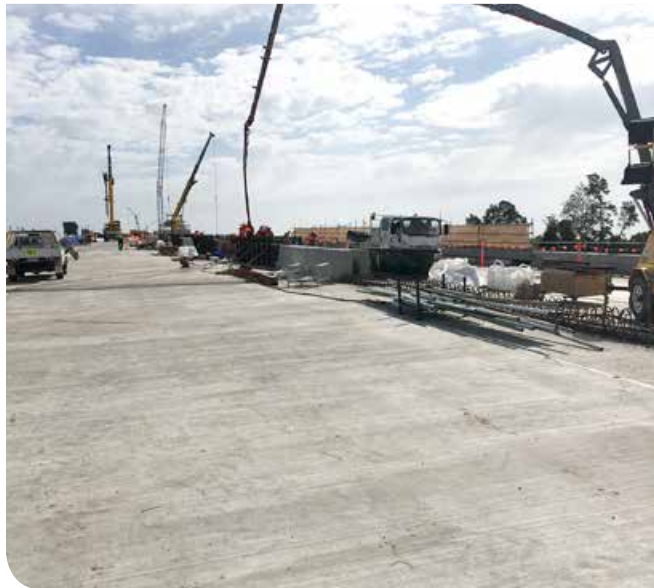
Installing of southern median barriers
