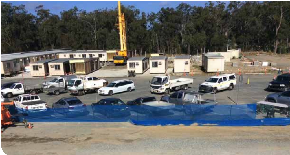
Demobilisation of office buildings at the main site compound
