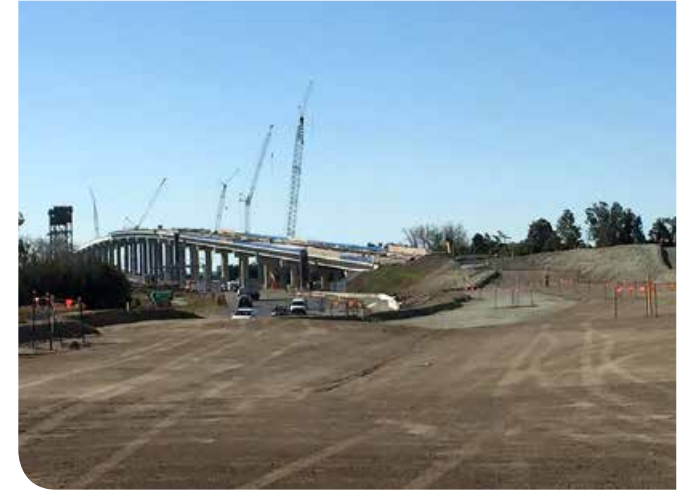
Progress of work at the Yamba interchange
