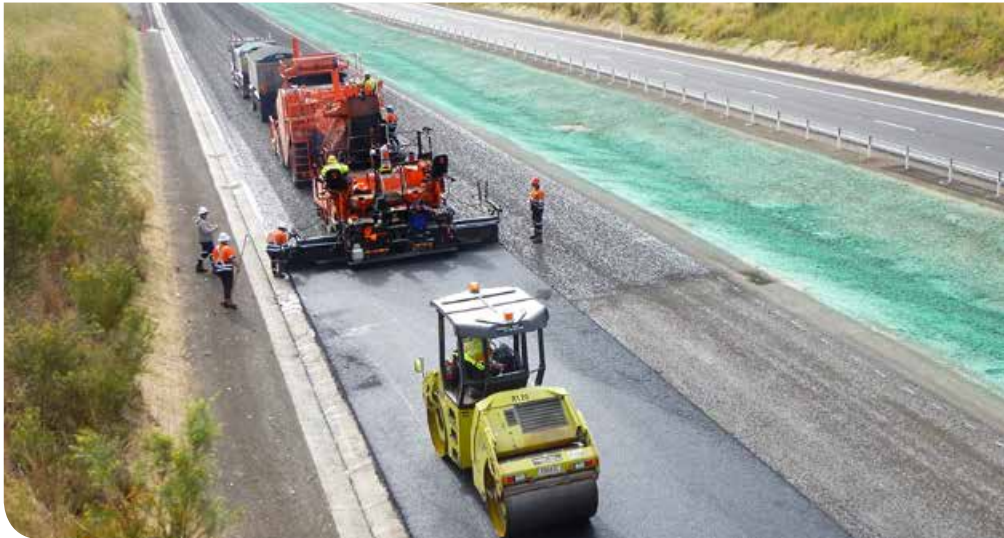
The final asphalt layers being applied near Rosewood Road, looking north
