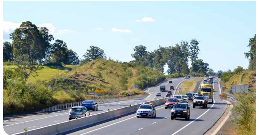
The first southbound vehicles on the new highway: A police car and a project vehicle
