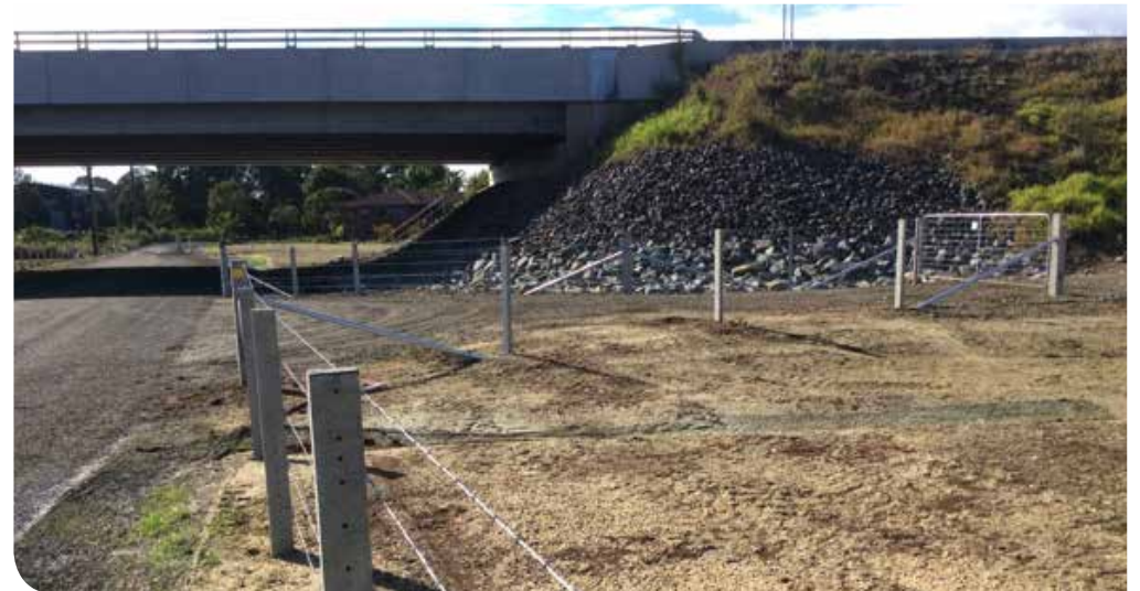
Final fencing and pavement work completed at Glen Ewan Road
