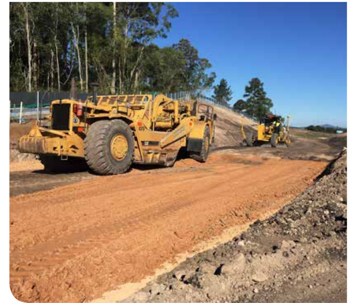
Earthwork at Iluka interchange
