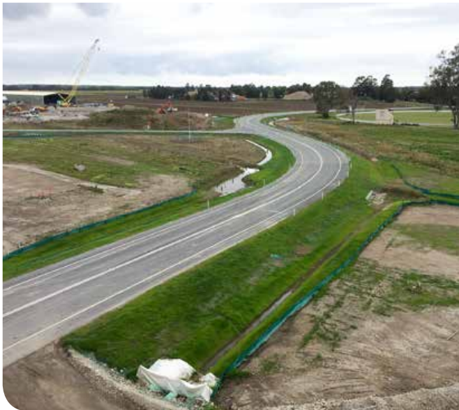
Link Oval Road extension complete
