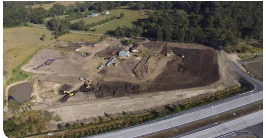
Restoration of the northern compound site at Cooperabung
