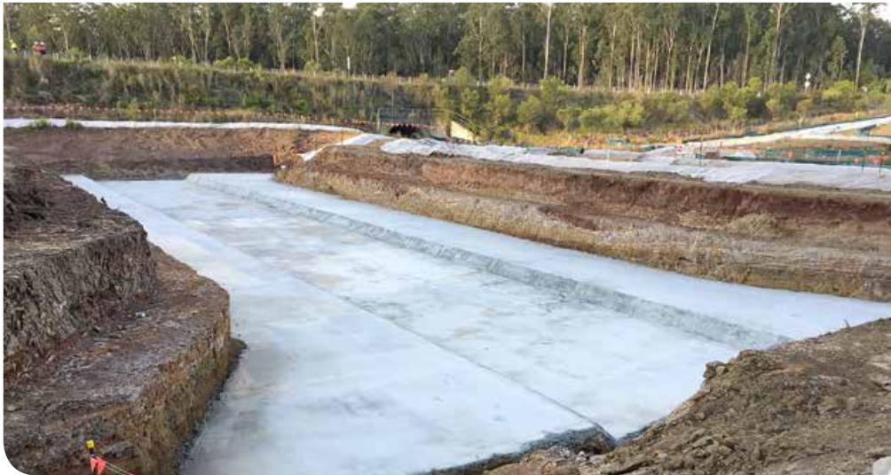
Drainage work at Glenugie
