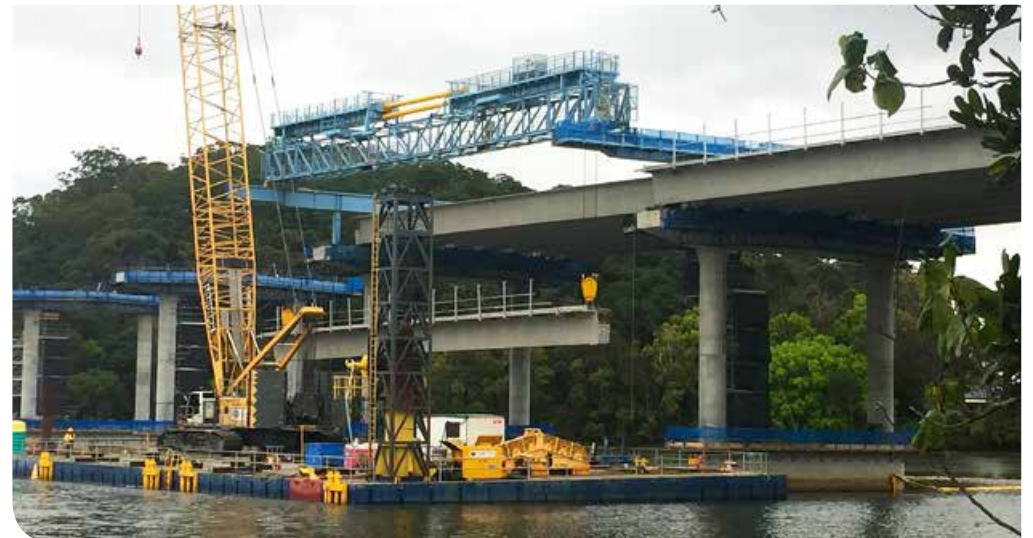
Installing marine girder at span 19
