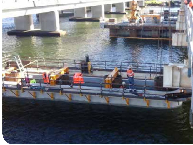
Installing pilecap shells for the new bridge at Mororo
