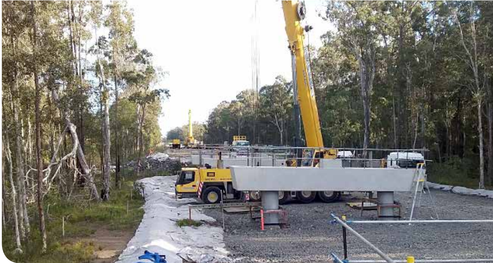
Installing headstocks on bridge at Tabbimoble
