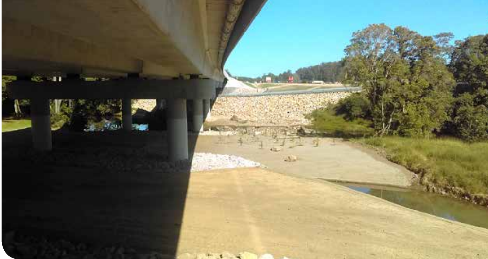
Revegetation and rock placing at Upper Warrell Creek
