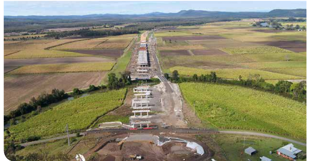
Aerial of bridge over Shark Creek at Shark Creek
