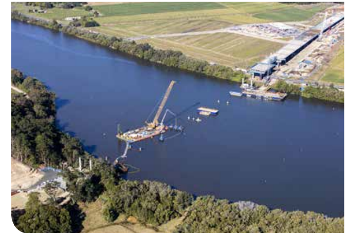
Aerial view north of Broadwater (June 2018)
