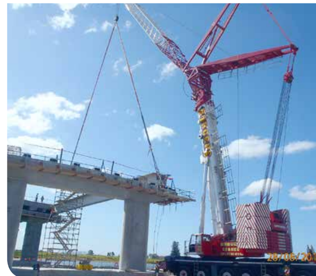
Girder delivery by crane, Harwood bridge
