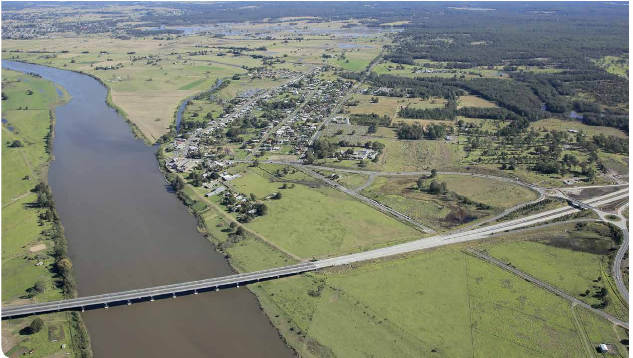
Macleay Valley Bridge, part of the Kempsey bypass
