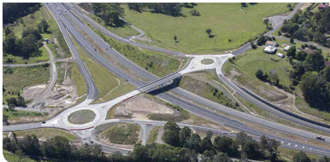
Bald Hill Road interchange looking south (April 2018)
