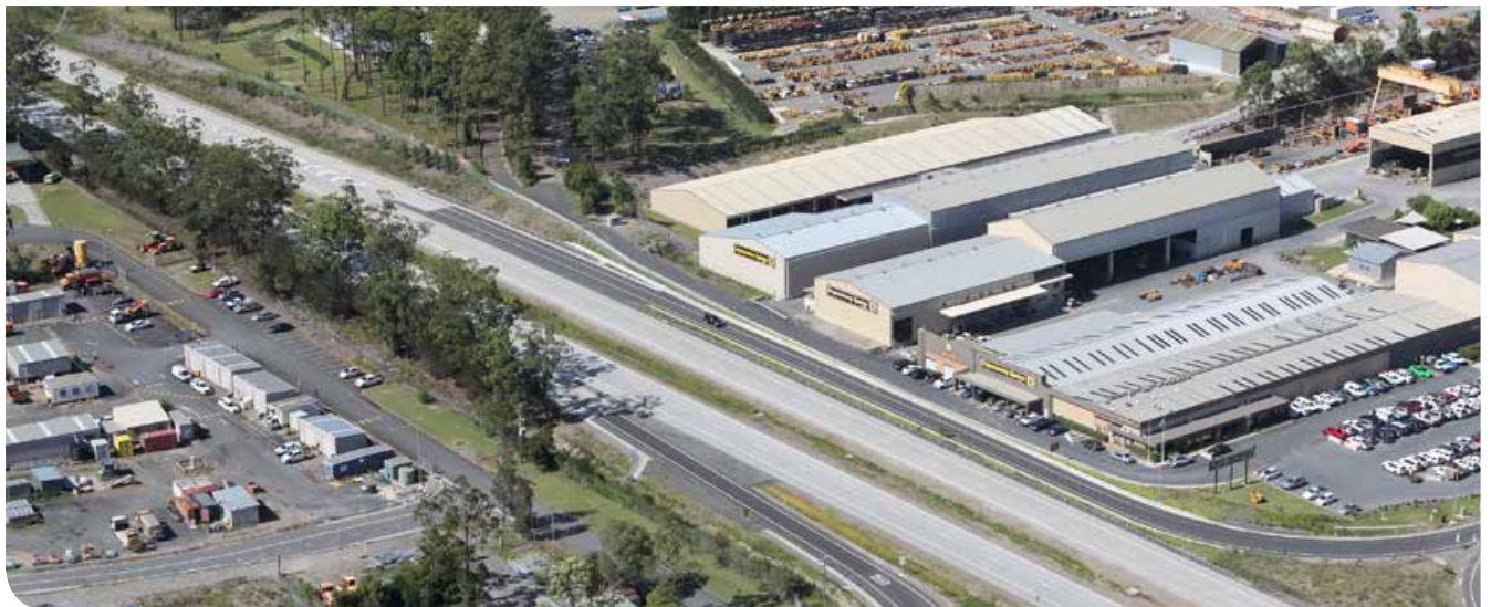
View of the Oxley Highway to Kundabung upgrade of the Pacific Highway and the growing industrial precinct at Sancrox, December 2017
