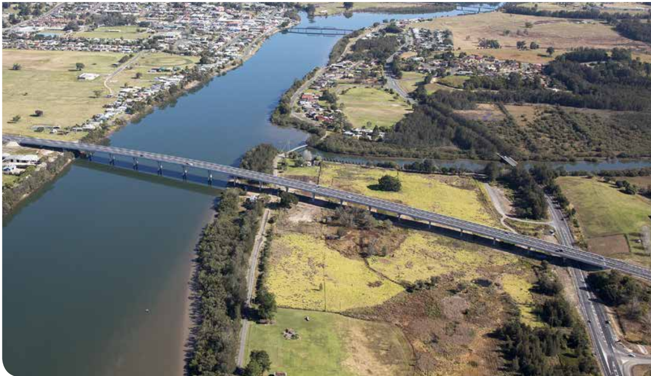
Aerial view of the Phillip Hughes Bridge bypassing Macksville
