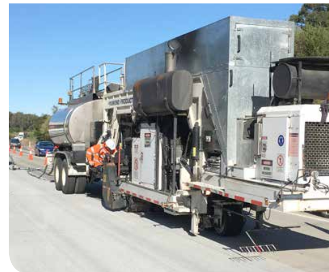
Diamond blade pavement grinding machine used to cut grooves into the concrete road surface as part of the pavement grinding trial and road noise perception survey on the Pacific Highway
