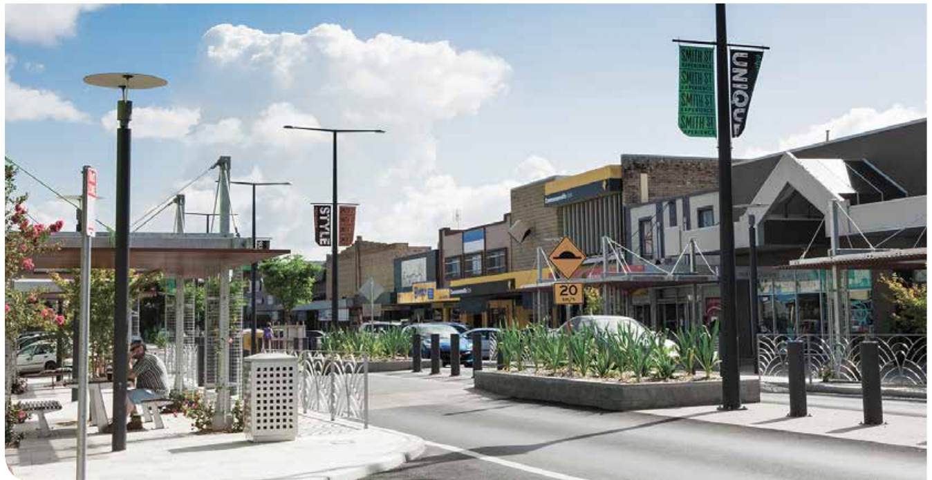
After Kempsey bypass
