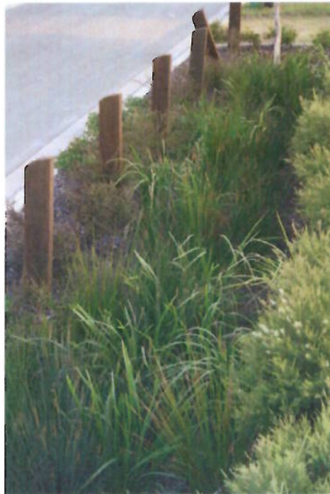
Figure 2B Example of a streetscape bioretention system at Bellvista on the Sunshine Coast, Queensland
