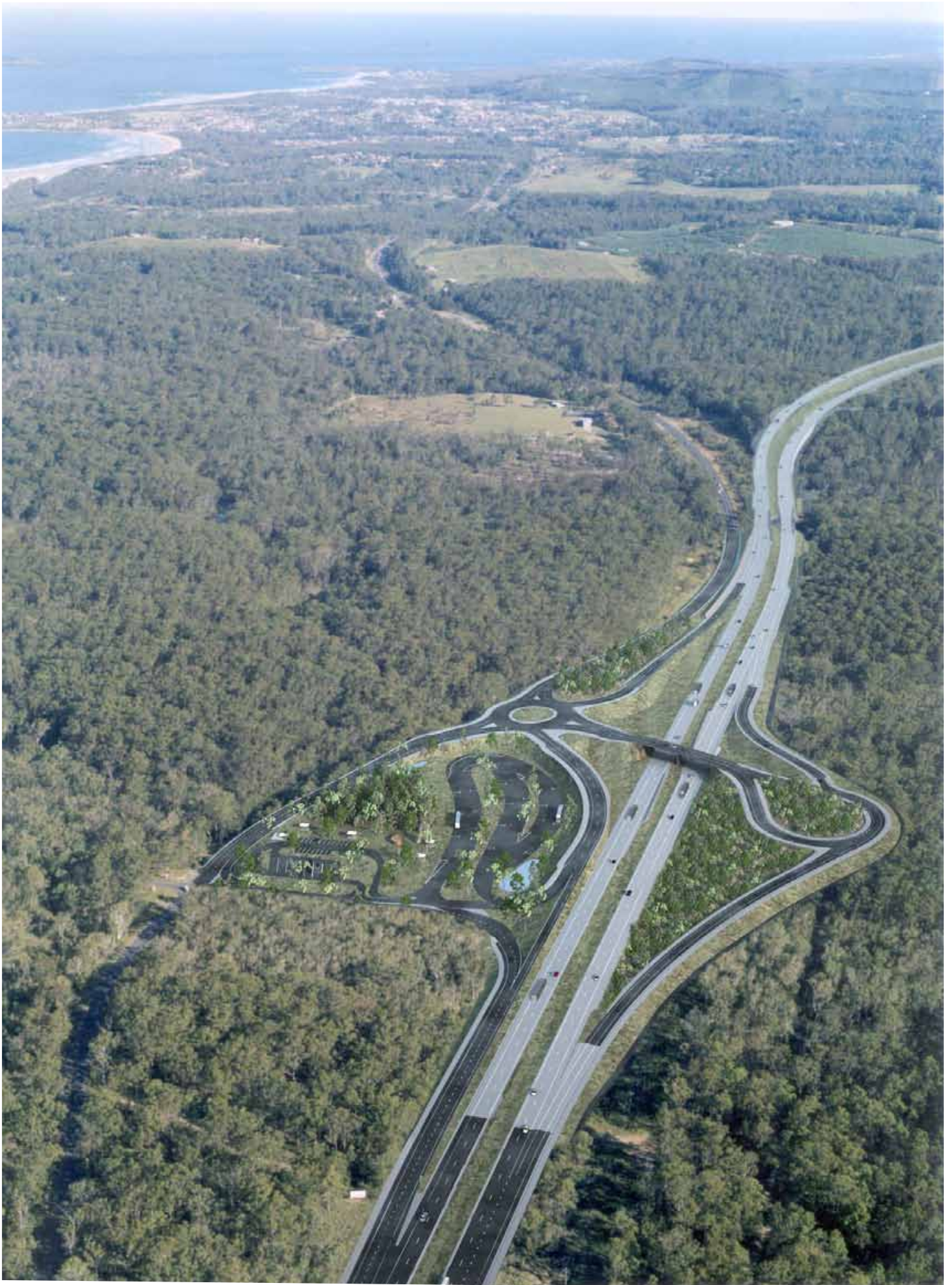
Sapphire to Woolgoolga Pacific Highway upgrade rest area modification EA
