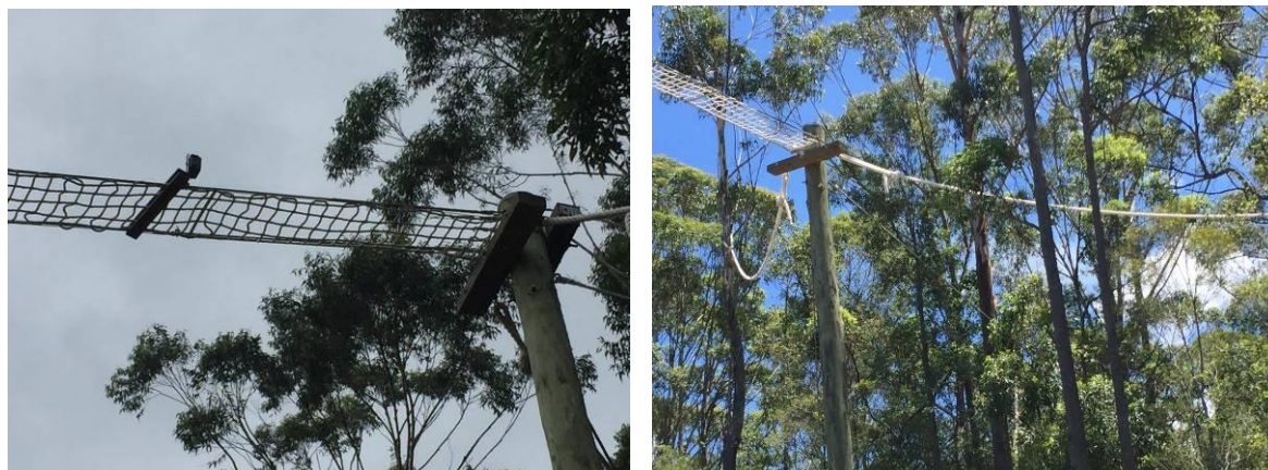
Plate 15: A Reconyx camera mounted to a wooden ‘sandwich board’ was positioned ~2m from each end of the rope bridge to capture moving fauna (L). 25mm silver rope was used to link the bulkhead to surrounding trees (R).
