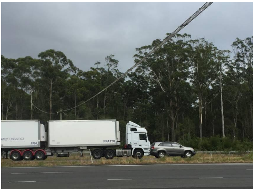
Plate 1: Expanse of the 86m-long Moonee rope bridge (ch.10720) looking north (upper). Habitat adjoining rope bridge on the east (middle) and west (lower) side of the alignment.
