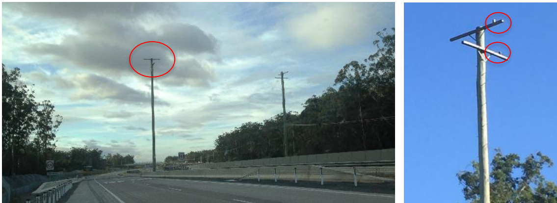
Plate 16: View of the glide pole array at Arrawarra creek looking north where cameras were installed on the central glide pole positioned between the carriageways (red circle) (L). Solitary Islands Way adjoins the dual carriageway immediately to the east (right of the photo). A Reconyx camera was mounted near the end of each arm of the pole (R).
