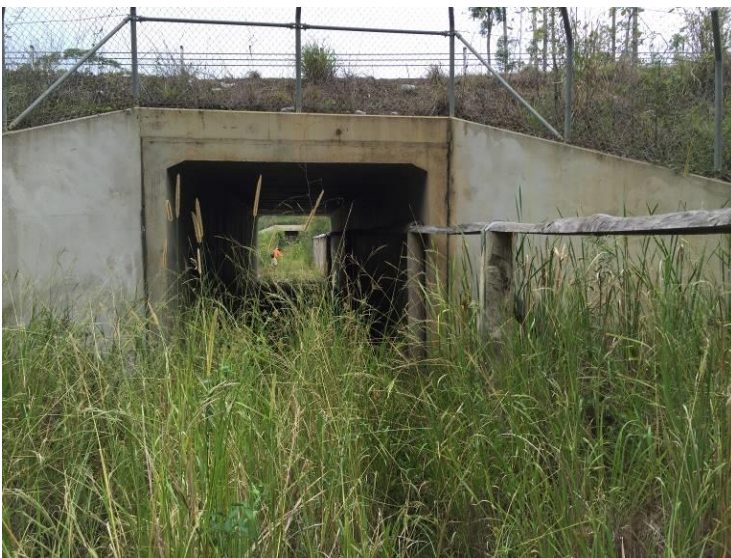
Plate 11: Arrawarra underpass north (ch.29930) viewed from the east (top), across the vegetated median (middle) and from west (bottom).
