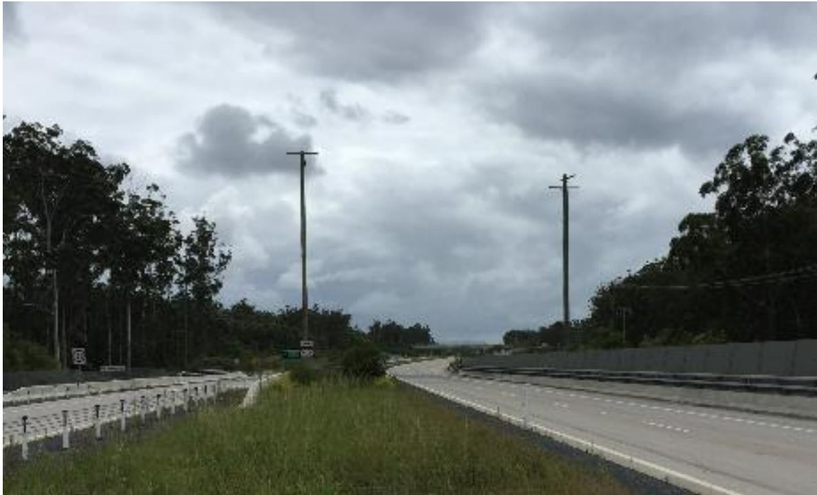
Plate 7: Habitat adjoining Arrawarra Creek glide poles (ch.31000) looking north. Cameras were installed on the central pole in the highway median.
