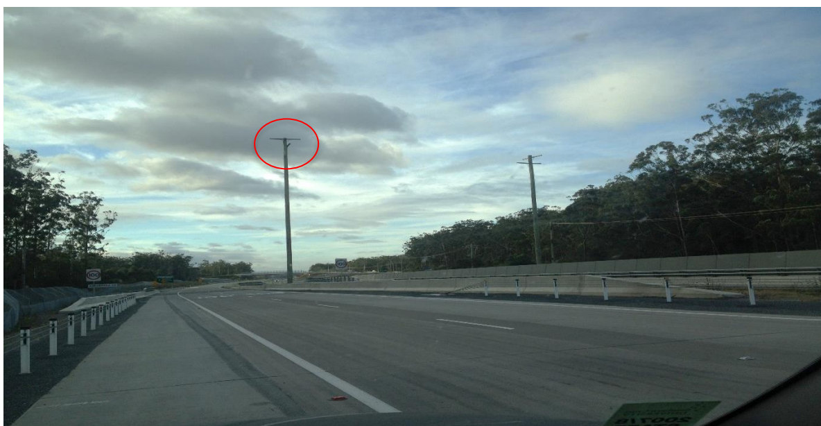
Plate 16: View of the two glide poles at Arrawarra creek looking north. Cameras were installed on the central glide pole positioned between the carriageways (red circle). Solitary Islands Way adjoins the dual carriageway immediately to the east (right of the photo).
