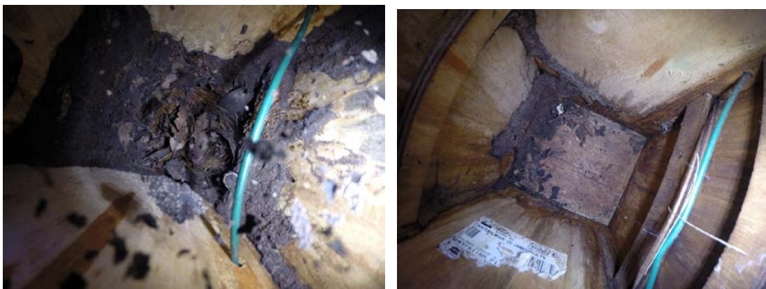
Plate 7: Box damage/deterioration was largely attributed to detached lids and termite attack as evident in a sugar/squirrel glider box (left) and a greater glider box (right).
