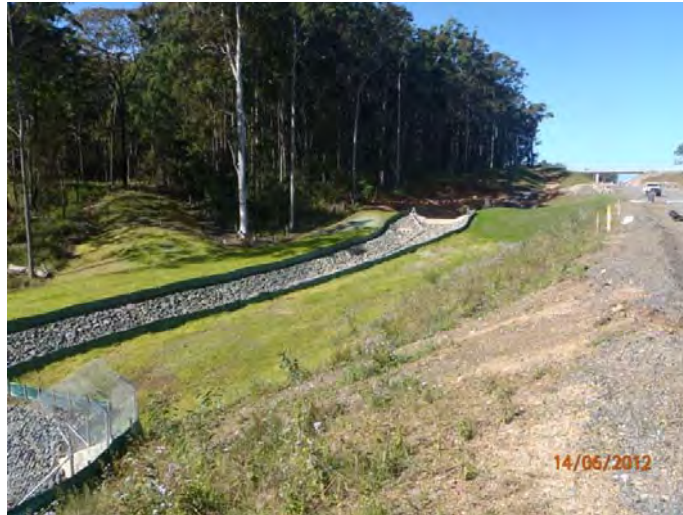
Photo – Sediment Basin (249) outlet and associated restoration and revegetation
