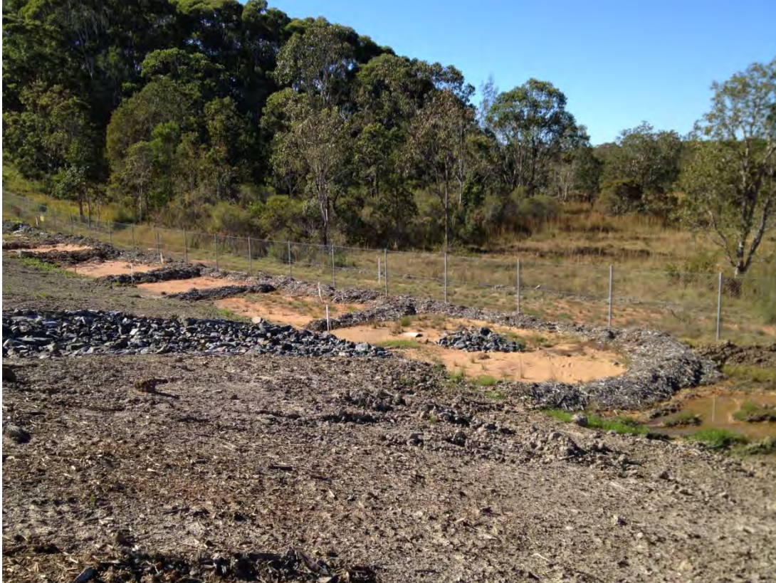
Photo 3: Mulch controls in series
