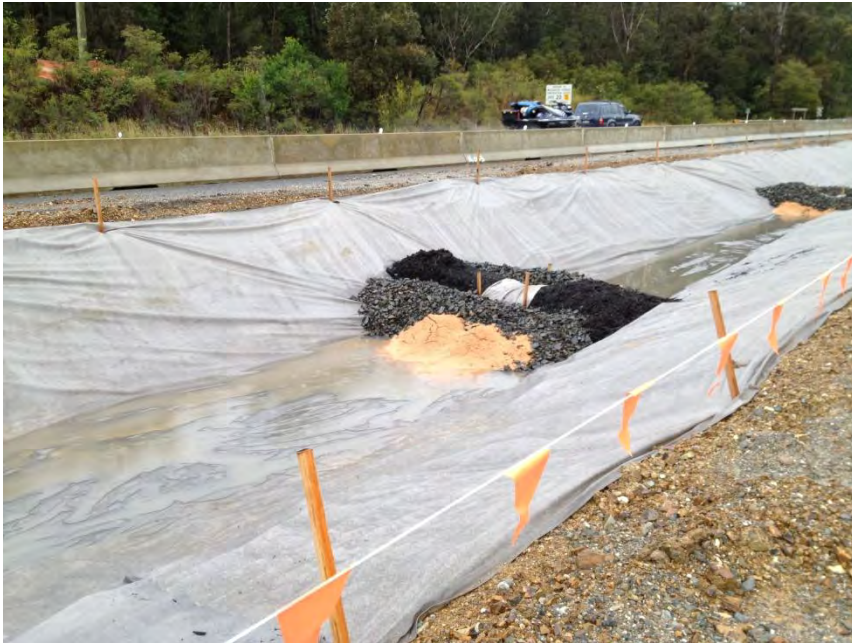
Photo 1: Controls within edge drain
