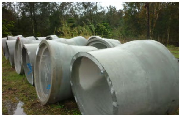
Photo – Pipe offcuts for reuse
