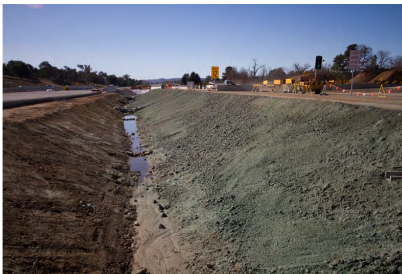
Photo – Gluon being used to stabilise batters
