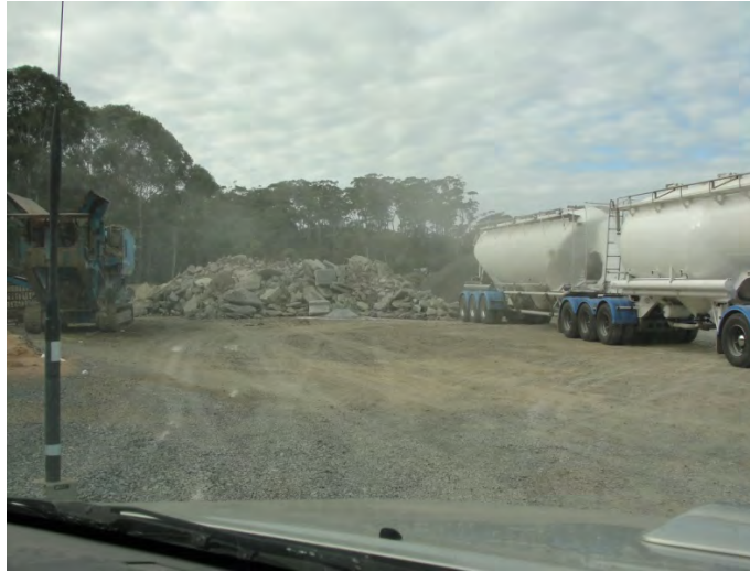
Photo – Concrete brought to Graham Drive for recycling for project use
