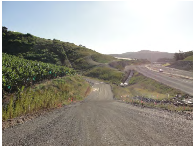
Photo- Revegetation of Cut 19, highlighting good integration of this cut batter into the landscape and progressive revegetation
