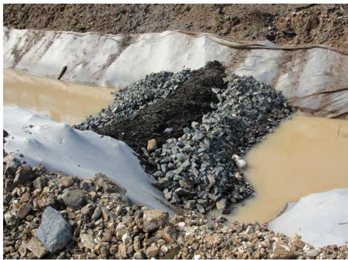
Photo – Use of combined mulch/ rock checks and gypsum.
