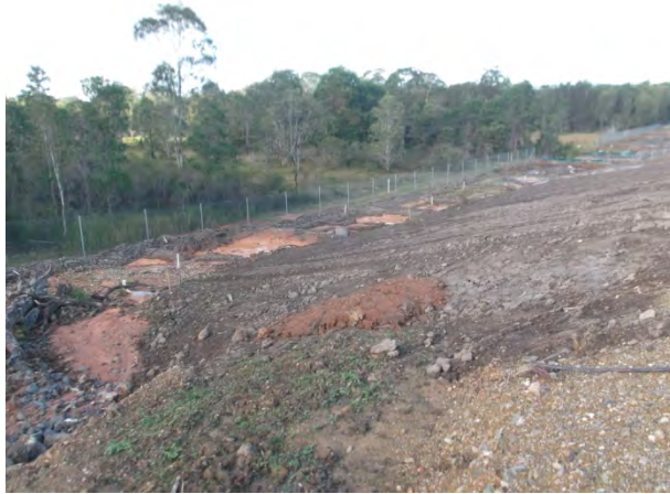
Photo – Use of controls in series, in this case using mulch.
