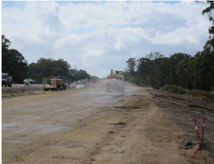
Photo – Water cart application to assist in dust suppression at Fill 10
