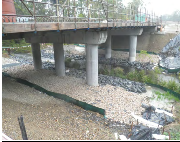
Photo-Fauna passage provided under Skinners Creek bridge.
