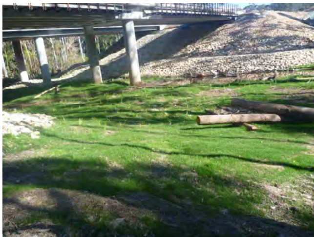
Photos-Restoration, revegetation and use of logs at Woolgoolga Creek.
