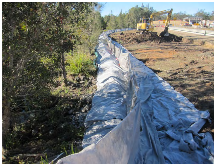
Photo – Use of multiple controls (sediment fence, geofabric, rock bund) near waterways.
