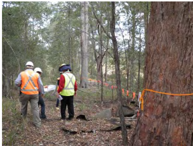
Photo – Two stage clearing process
