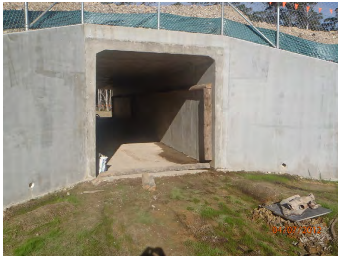
Photo – Fauna underpass with refuge poles and connecting rails
