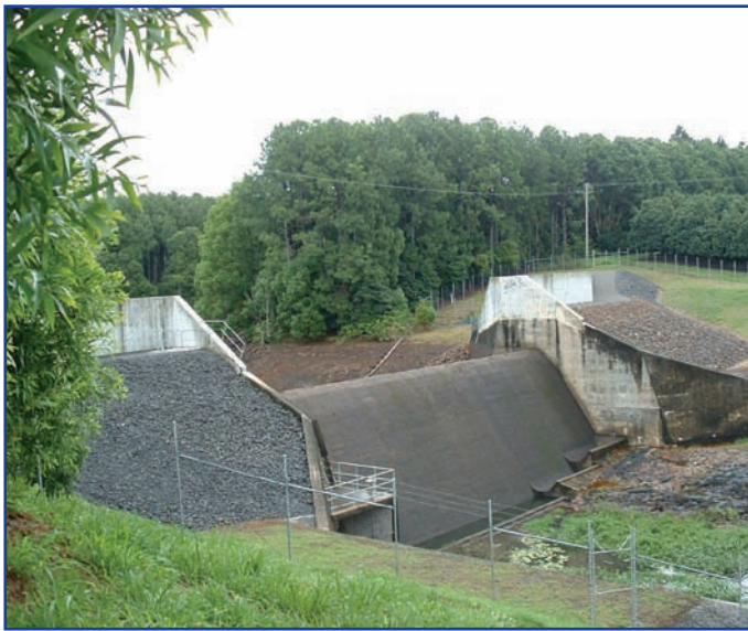
Emigrant Creek dam
