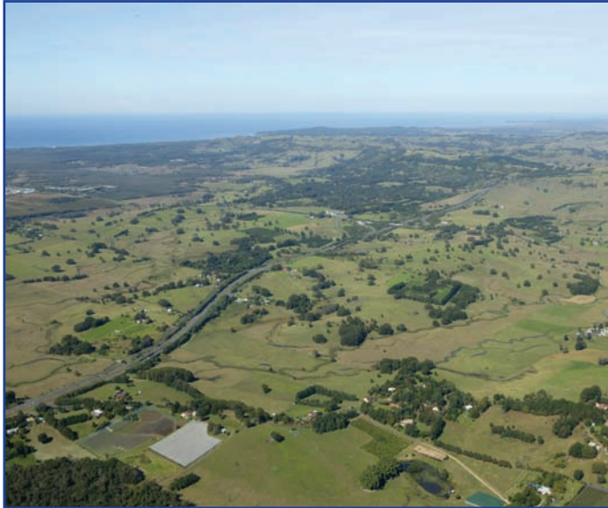
Visual assessment precinct 5 looking south-east. Ewingsdale interchange is in the centre of the photograph.
