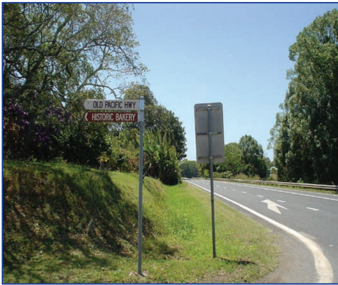
Existing at-grade intersection on the Pacific Highway at Newrybar.
