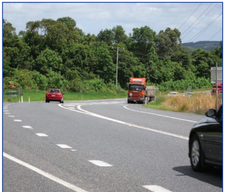
The existing at-grade intersection between the Pacific Highway and Ross Lane.
