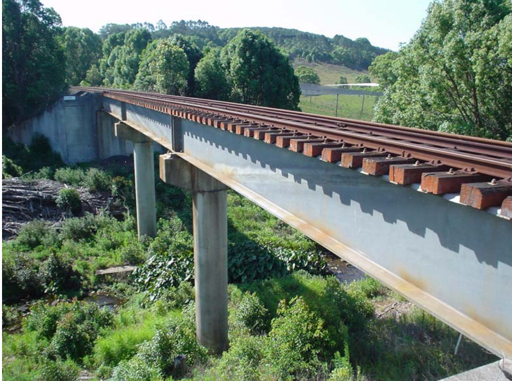
Figure 2 High Level Rail Bridge over Tinderbox Creek
