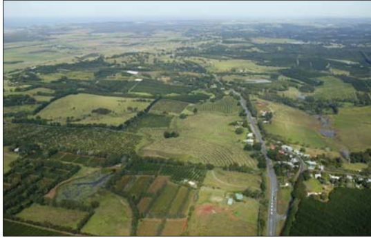
Illustration 31: Aerial Overview of the Emigrant Creek precinct
