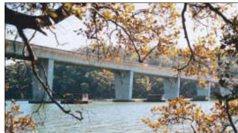
Illustration 93: Reverse tapers on the long elevation of the Alford's Point Bridge (source: RTA 'Bridge Aesthetics', p 17)
