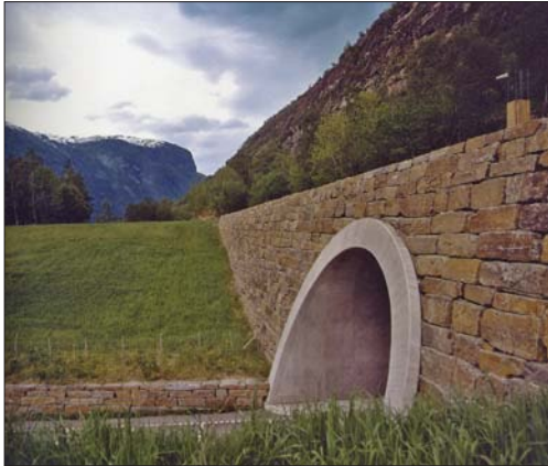
Illustration 101: Detail of the simple but refined suite of materials used around the portal of the Laerda tunnel. The smooth concrete tunnel creates an attractive contrast with the head wall made from local rock material.
