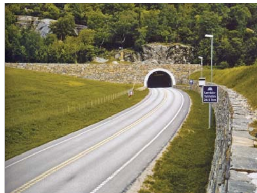
Illustration 100: The Laerda tunnel in Norway is a good example of an integrated design of the tunnel portal, safety barriers, cuttings and retaining structures that is sympathetic to the surrounding landscape. A similar approach may be suitable for the prominent southern tunnel portal on the Ewingsdale spur.
