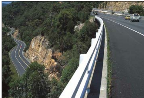
Illustration 96: This transparent barrier along the F3 Freeway allows good views of the surrounding landscape. Using round instead of square sections would further reduce the perceived thickness of rails (image source: RTA)
