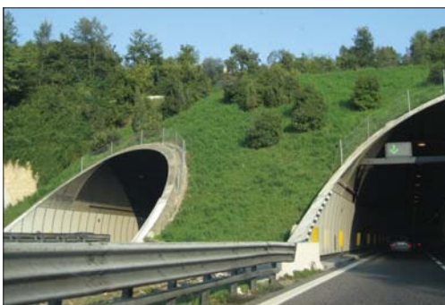
Illustration 103: Example of a tunnel portal shaped to correspond to the natural hill slope.
