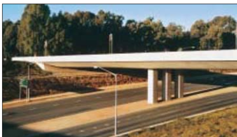
Illustration 92: The bridge is tied to the surrounding landscape by the parapet that continues past the abutments (source: RTA 'Bridge Aesthetics', p 26)
