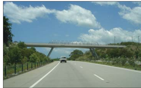
Illustrations 97 and 98: Two examples of overbridges on the Pacific Highway with symmetrical pier layout and piers meeting the bottom of spill abutments, resulting in good transparency of the structure.
