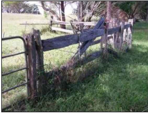
Plate 4.48 T2E H31 – Remnant post and rail fencing
