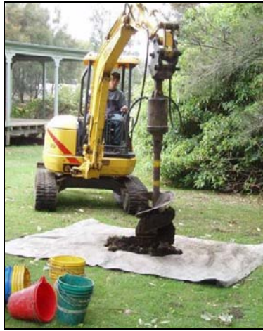
Excavating a mechanical auger test pit
