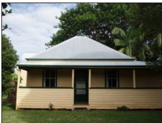
Plate 4.52 T2E H32 – Front view of cottage, looking west
