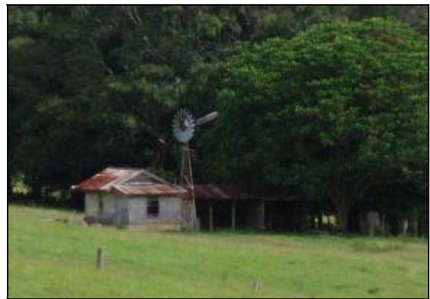
Plate 4.47 T2E H30 – View of disused farm buildings, looking southwest
