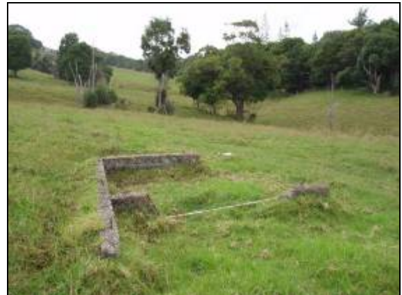
Plate 4.68 T2E H40 – Concrete footings and floor, looking south
