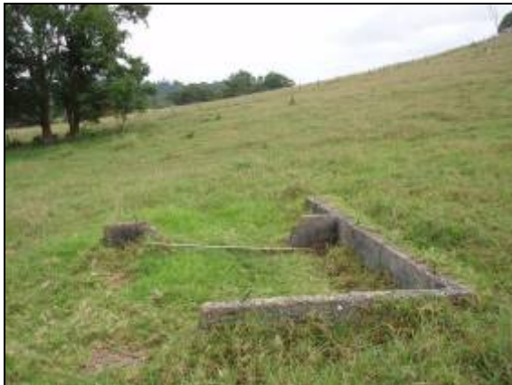
Plate 4.67 T2E H40 – Concrete footings and floor, looking northeast
