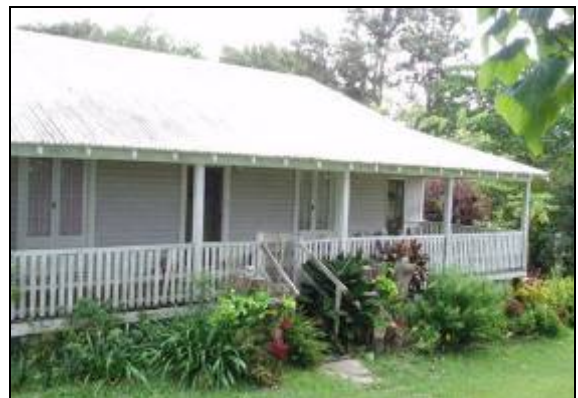
Plate 4.28 T2E H18 – view of eastern face (front) of former teacher's residence
