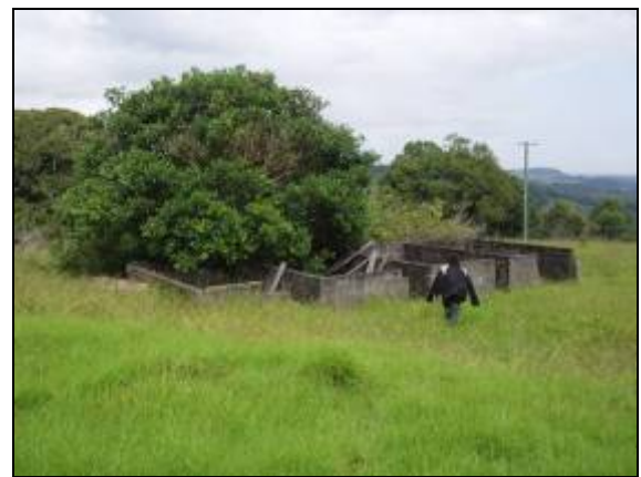
Plate 4.24 T2E H13 – The remains of concrete animal pens (possibly a piggery) at the southwestern end of the complex
