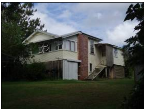
Plate 4.29 T2E H18 – view of rear (northwest corner) of former teacher's residence
