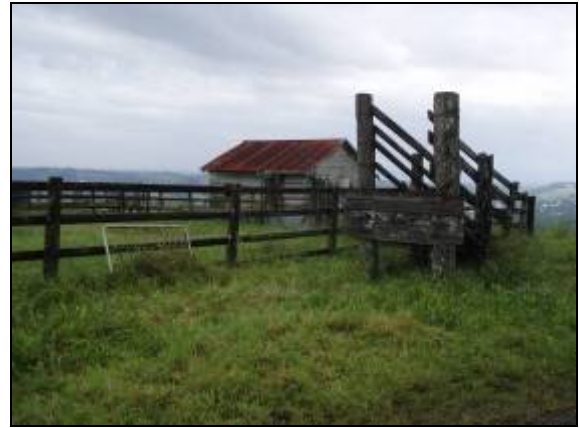
Plate 4.22 T2E H13 – View looking west towards former dairy building and modern yards
