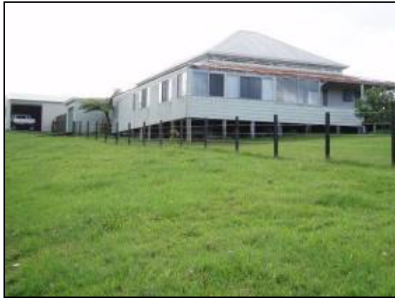
Plate 4.35 T2E H21 – The southeastern aspect of the western cottage.
