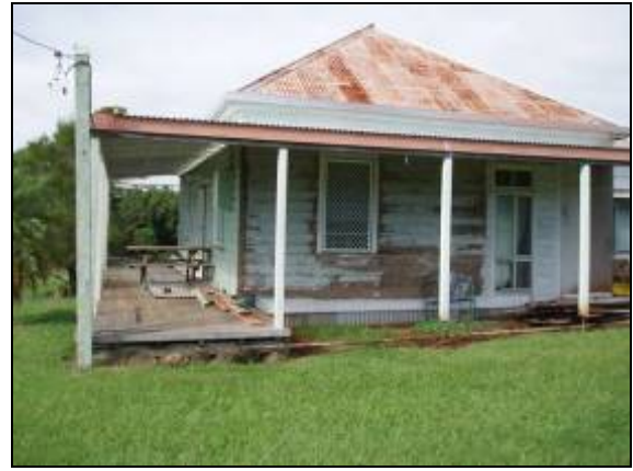
Plate 4.36 T2E H21 – Detail of veranda on first (eastern) cottage.
