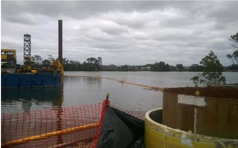
Photo 1: Oil boom surrounding waterways working platform – Nambucca River
