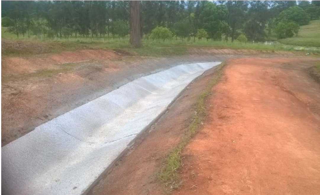
Photo 7: Permanent drainage works (northern zone)
