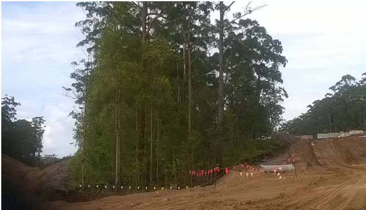
Photo 5: Widened median with retained vegetation for glider crossings (northern zone)
