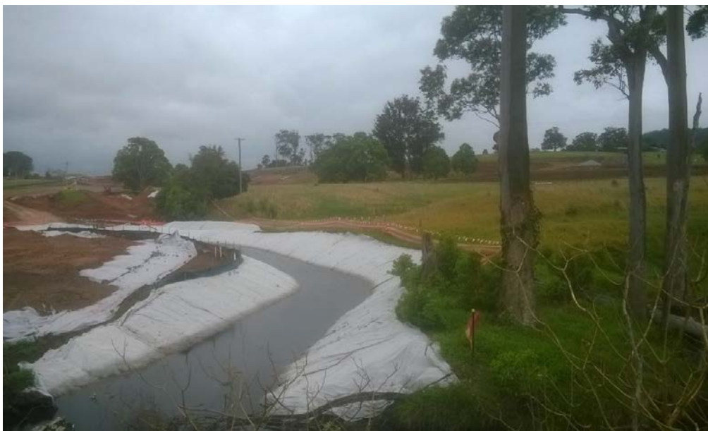
Photo 2: Temporary cross drainage (south zone)
