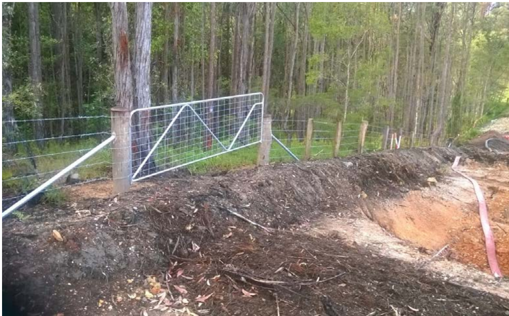
Photo 4: Permanent boundary fencing and property access (northern zone)
