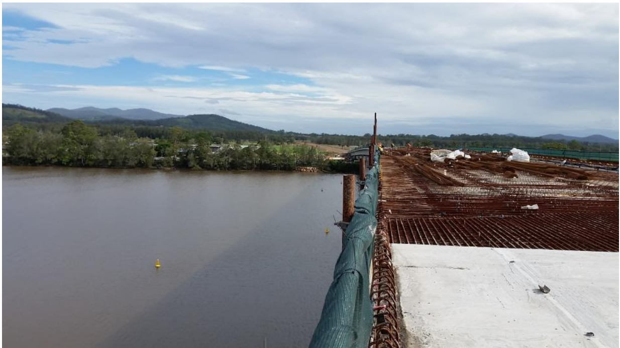
Photo 4: Nambucca River Bridge deck construction is ongoing.
