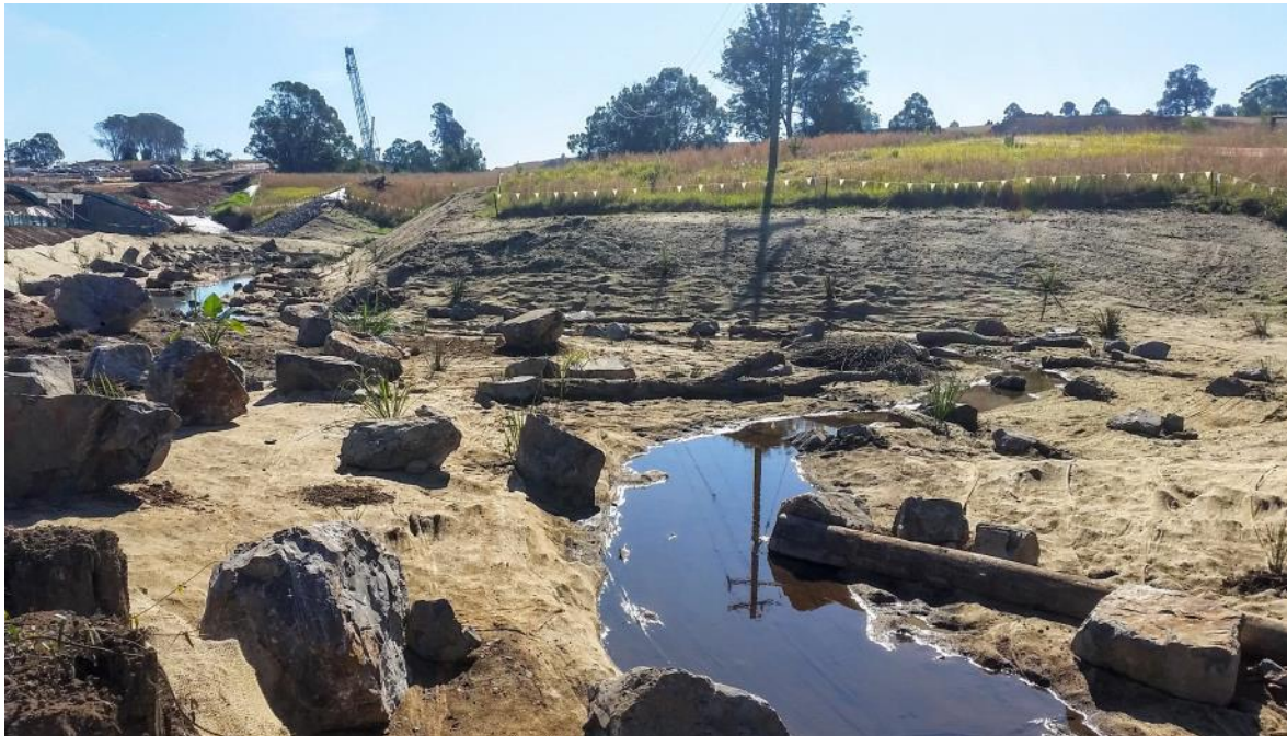
Photo 10: Stoney Creek after diversion and soft landscaping treatments have been installed
