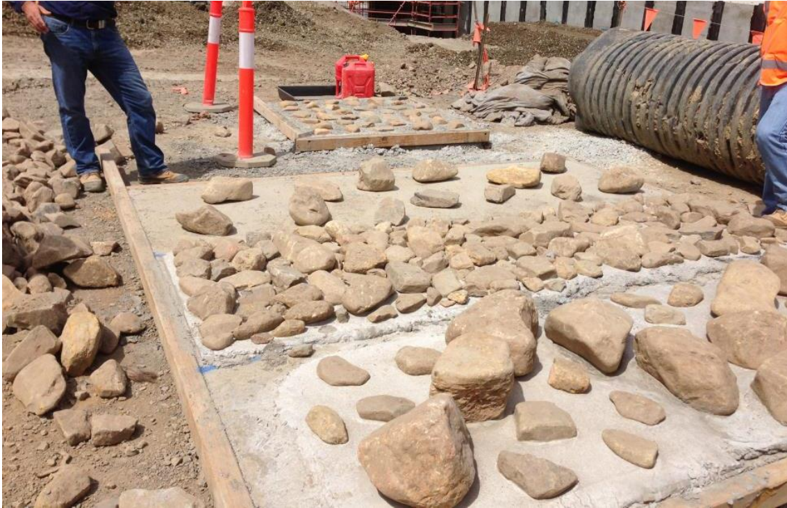
Photo 8: Test panels used to determine the most ideal rock/stone pitching
