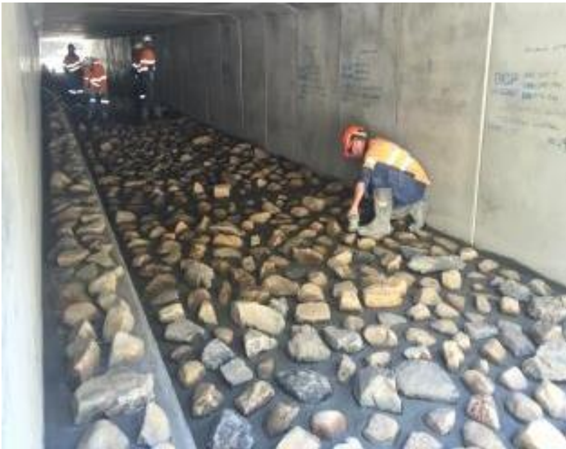
Photo 9: Installation of the chosen rock placement
