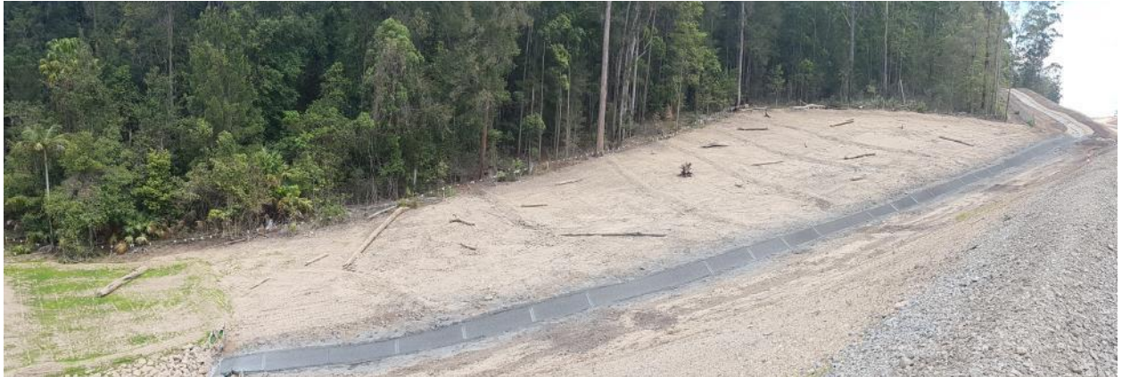
Photo 5: Permanent landscaping and rehabilitation works have commenced.
