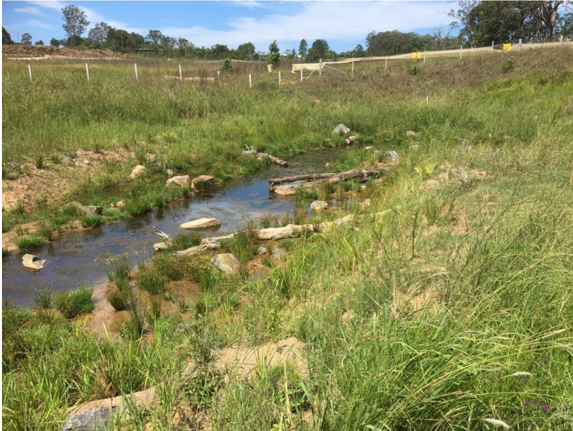
Photo 11: Stoney Creek after landscaping treatments have established, the creek line has withstood several large rainfall events and is stable.
