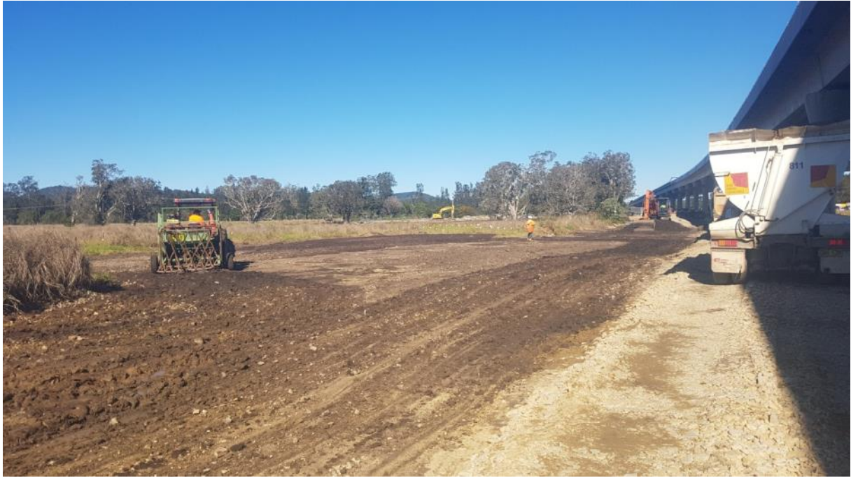
Photo 4: Rehabilitation of floodplain on the northern side of Nambucca River
