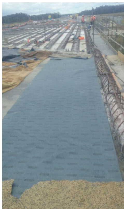
Photo 8: Use of carpet underlay for wet curing
