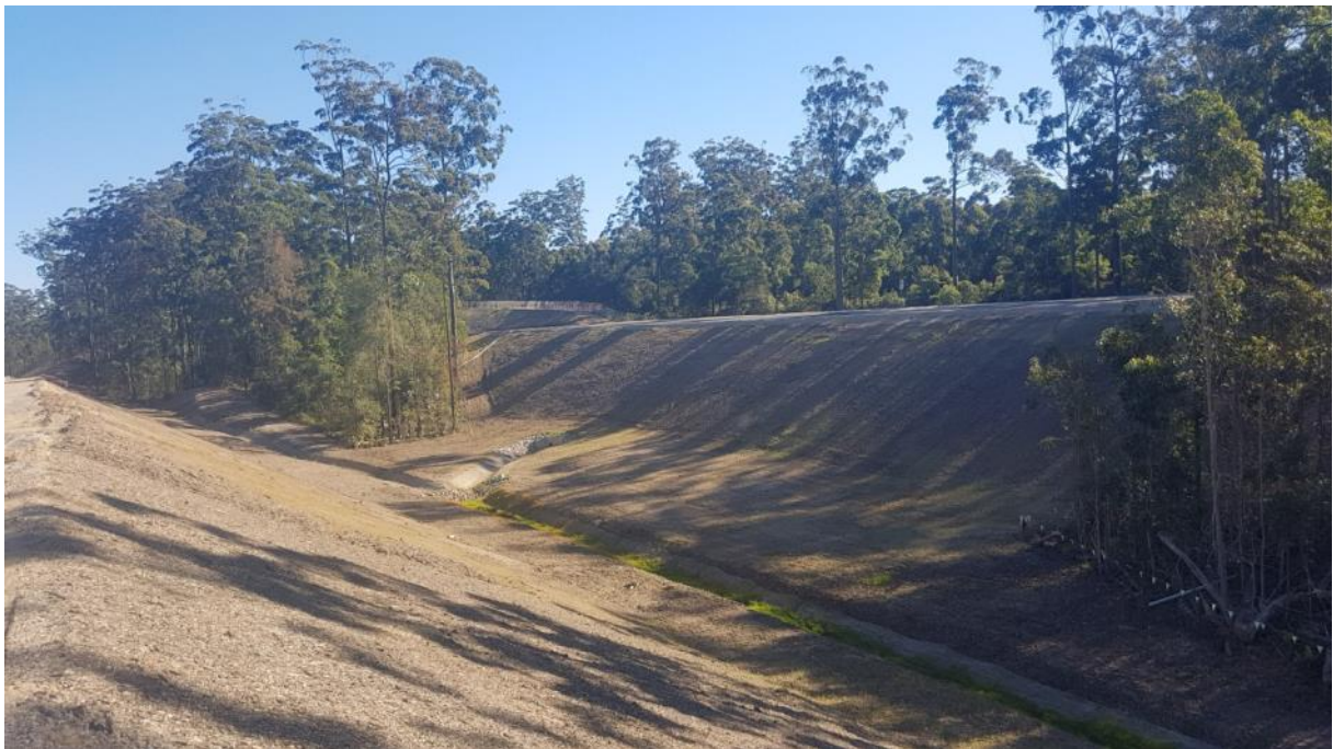
Photo 5: Widened median through the Nambucca State Forest to allow glider crossing points.
