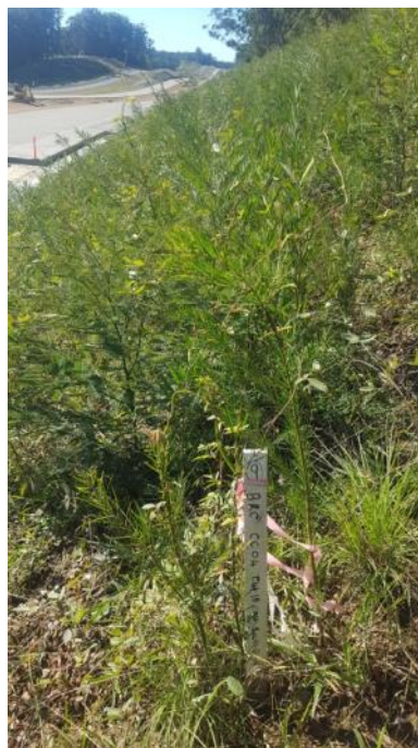
Photo 3: Revegetated batter, part of the permanent landscaping in the Southern area of the Project
