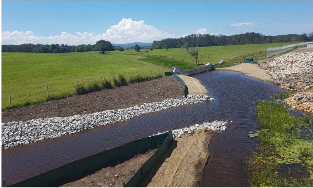
Photo 4: Temporary Waterway Crossing Rehabilitation Works at Floodplain Bridge 1
