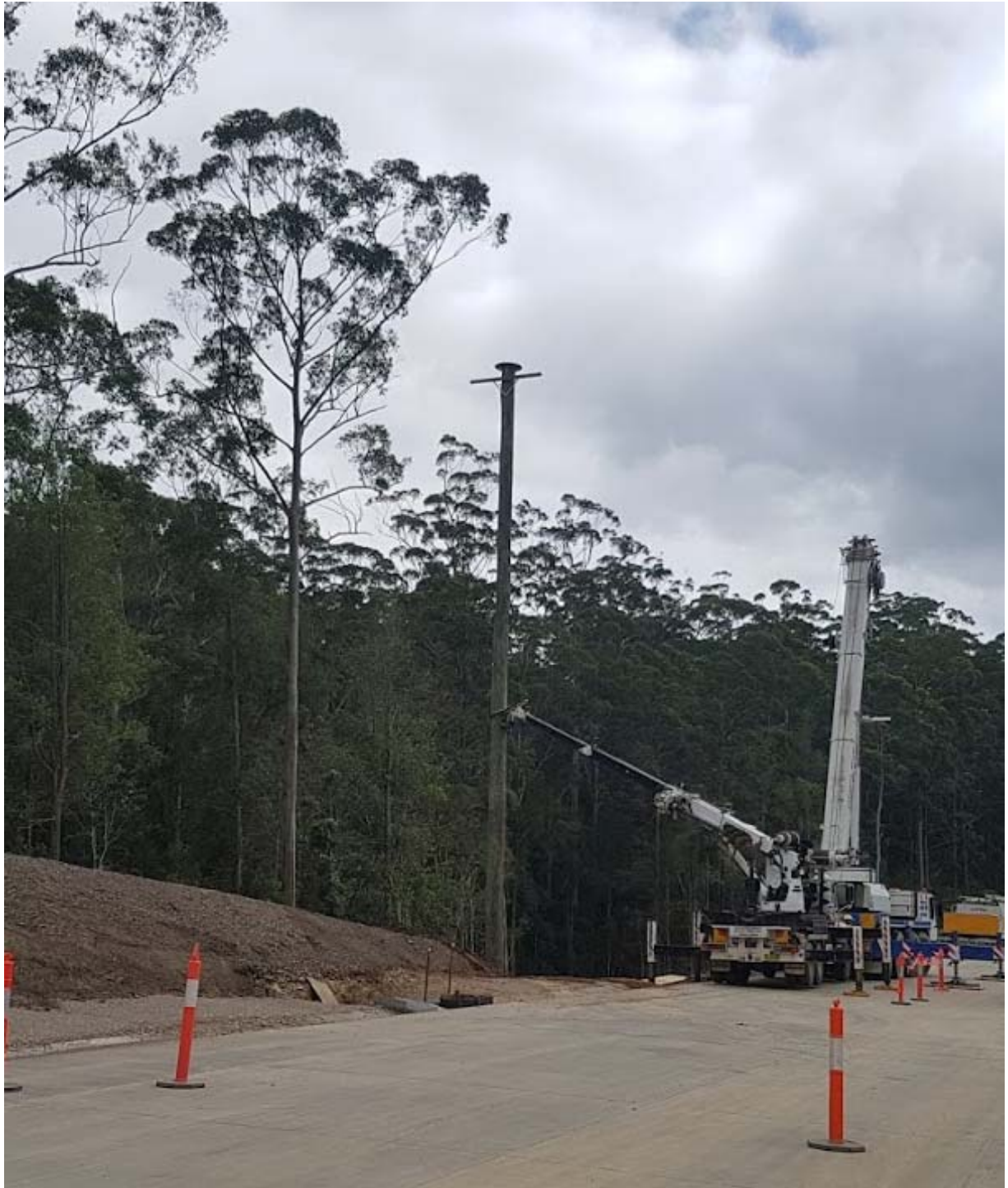
Photo 1: Glider Pole Installation – Widened Medians (Nambucca State Forest)
