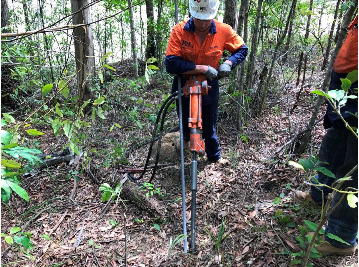
Photo 5: Installation of the Hulk Anchor on the WC2NH Project (Widened Medians)
