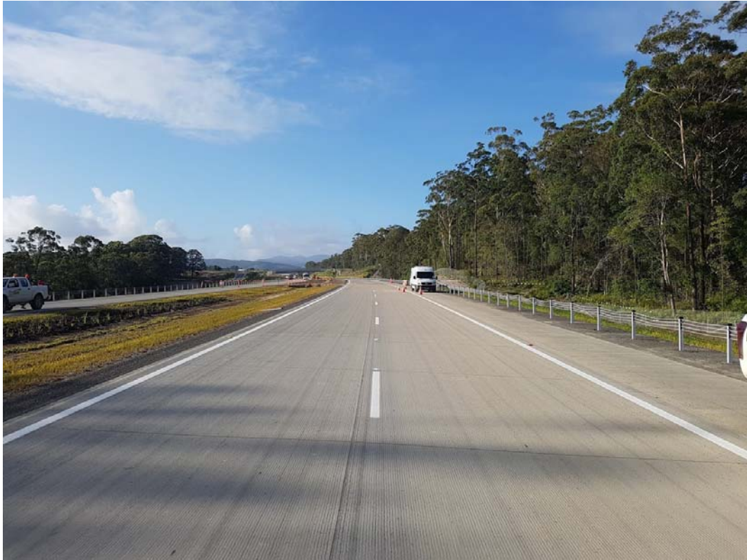
Photo 2: Line Marking and Finishing Works – Northern Section (Partial Opening Stage 2A)
